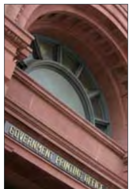
GPO entrance on North Capitol Street, NW.
