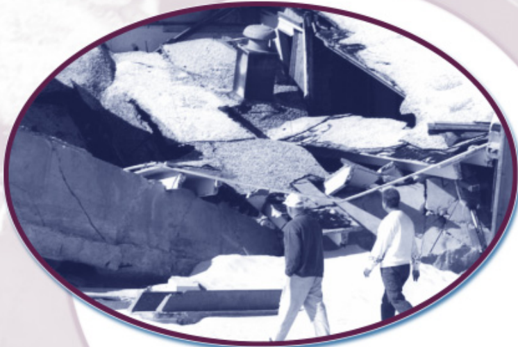
A house wrecked from a hurricane on a Pensacola, Florida, beach.
