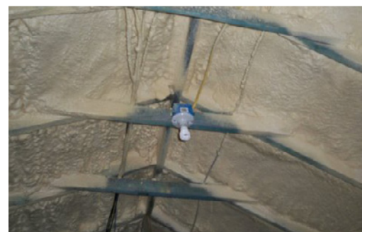
(1) Batt insulation in ceiling. (2) Blown-in insulation. (3) Spray foam. (Photo source: Sam Garst). (4) Spray foam applied along the underside of the roof deck to provide a conditioned and non-vented attic space for ducts and air handlers.
