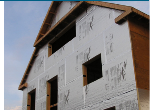
Nelson Construction of Farmington, Connecticut, uses two inches of foil-faced polyisocyanurate insulating sheathing taped at the seams for an insulated air sealed exterior that is finished with Tyvek house wrap and vinyl siding.
