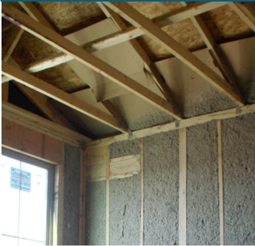
Baffles allow ventilation under roof decking while keeping wind from blowing insulation back from the edges of an attic.
