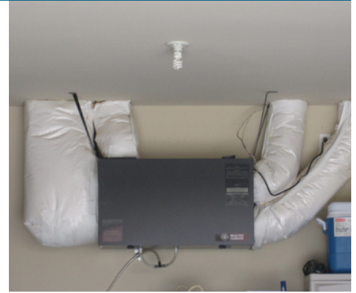
(top) Every home is equipped with an energy-recovery ventilator to provide conditioned fresh air throughout the home.
