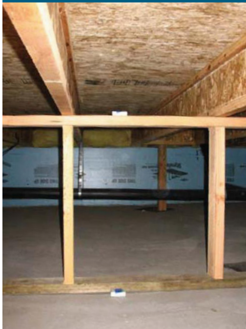
Unvented, insulated crawlspaces are recommended in the cold climate in the eastern and midwestern United States, where high humidity levels can cause moisture problems in vented crawlspaces.
