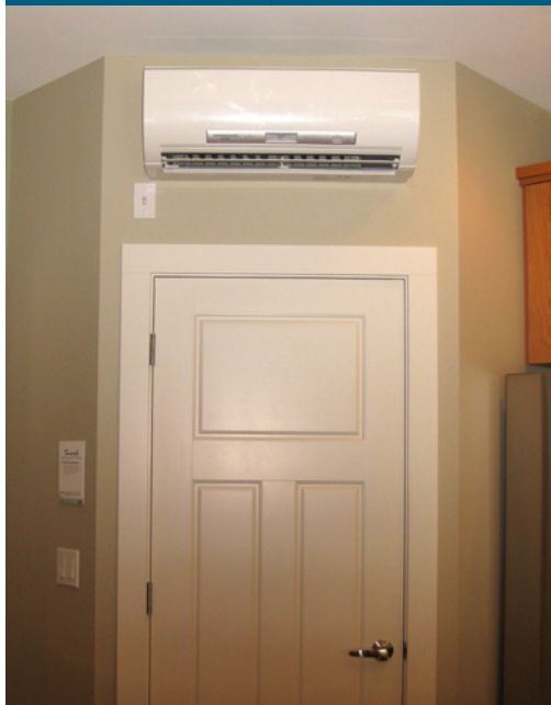
Ductless heat pumps mount to the wall to provide zonal heating and cooling with exceptional energy performance.
