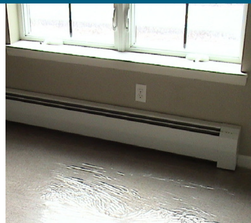
Hydronic heating in condominiums in Aspen, Colorado, uses water that is preheated by solar thermal panels, then heated by a gas boiler, and distributed via baseboard radiators.
