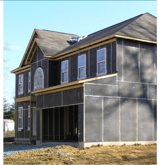
(top) Bob Ward Companies used an exterior wall sheathing consisting of a 1/8-inch layer of laminated fiberboard covered with 1/8-inch of extruded polystyrene foam board. This layer goes on the exterior side of the studs under the stone or wood siding. Joints are taped so the foam board serves as an air barrier as well, eliminating the need for housewrap. This exterior insulation layer moves the dew-point surface to the outside of the framing member, reducing the potential for condensation and moisture damage within the wall cavity. (Photo source: Bob Ward Companies)
