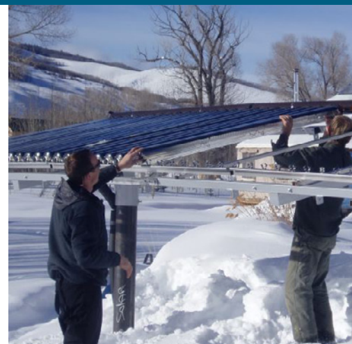
Evacuated tube collectors are one solar water heater type that works well in cold climates.
