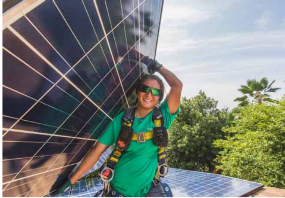
Technician installs rooftop solar system to boost residential energy efficiency. (Photo: SolarCity)
