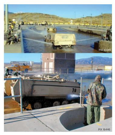
Soldiers hose down trucks with high-pressure water to clean off debris in the Fort Carson Central Vehicle Wash Facility. The basin, known as a "birdbath," collects the water for reuse.
