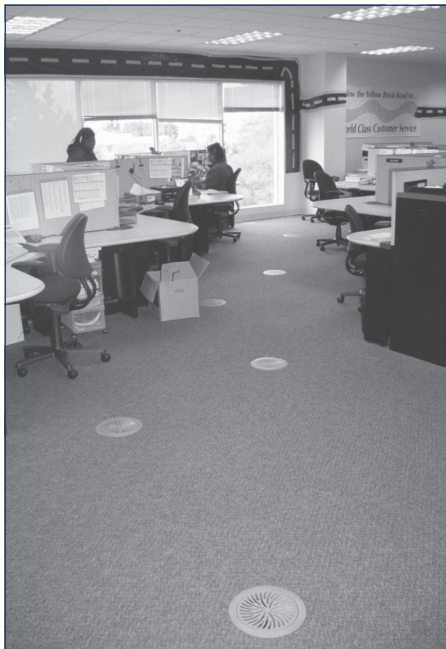
Figure 4. Typical interior swirl diffuser layout.
