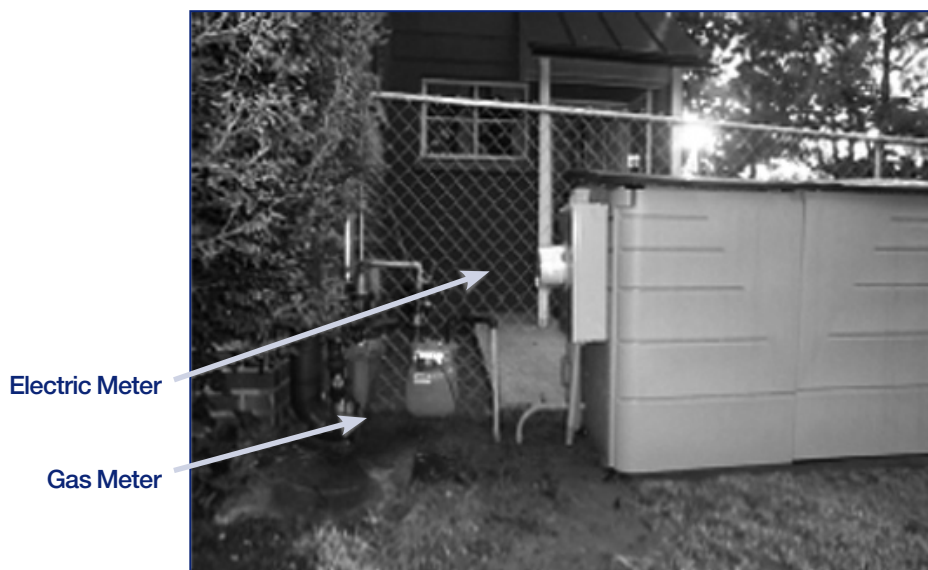
Figure 4. Residential-type meters to record gas input and electrical output.
