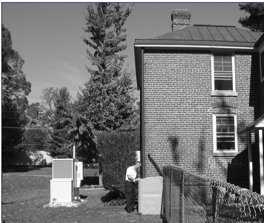
Figure 3. Demonstration PEM fuel-cell-based CHP unit (left) at Fort McPherson.
