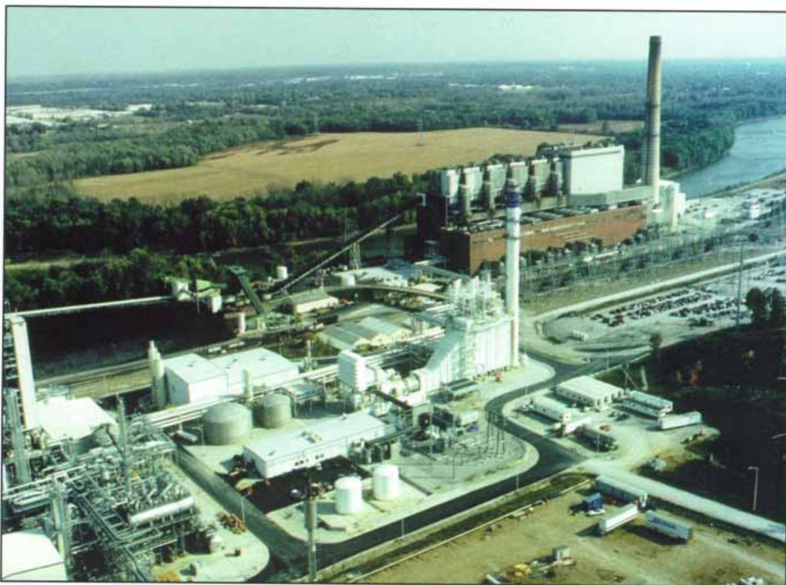
The Wabash River IGCC power plant. The gas cleanup system is on the left and the combustion turbine/HRSG unit is in the center. The Wabash River coal-steam plant is in the background by the Wabash River; repowered Unit 1 is on the left.
