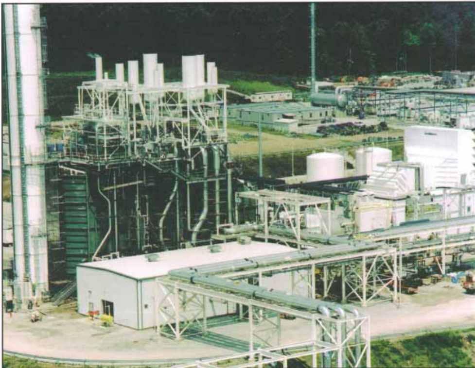
Wabash River gasifier/combustion turbine/HRSG train during construction. The pipe rack, foreground, connects to the repowered steam turbine Unit 1.
