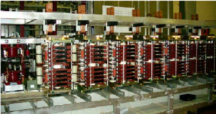
Figure 8-14b A 30MW Medium voltage power management system and the 9MVA IGCT power electronic building block (51)
