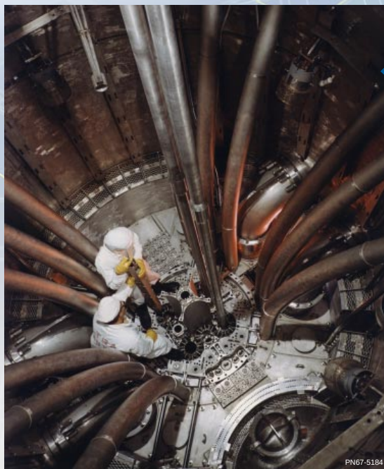
Advanced Test Reactor (No. 3) is used to study the effects of radiation on materials and also produces rare and valuable medical and industrial isotopes. It is the largest test reactor in the world.
