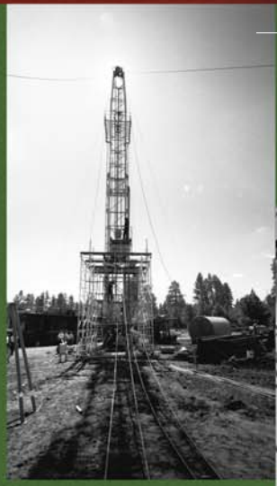
*** Dean List lowered canisters of SNL instrumentation 4,600 feet down into a drilling hole designed to measure the shock waves of the explosion.
