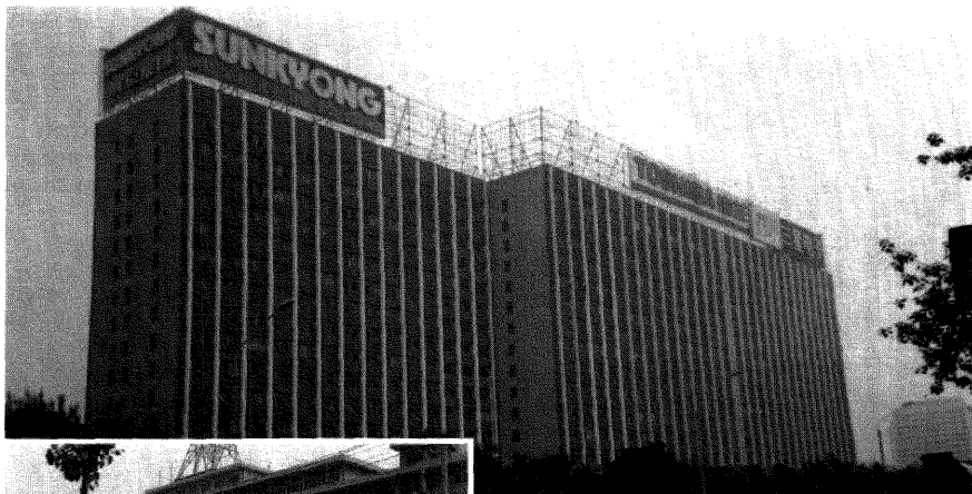
This office building in downtown Beijing houses most of the research institutes of the Chinese Academy of Social Sciences.
