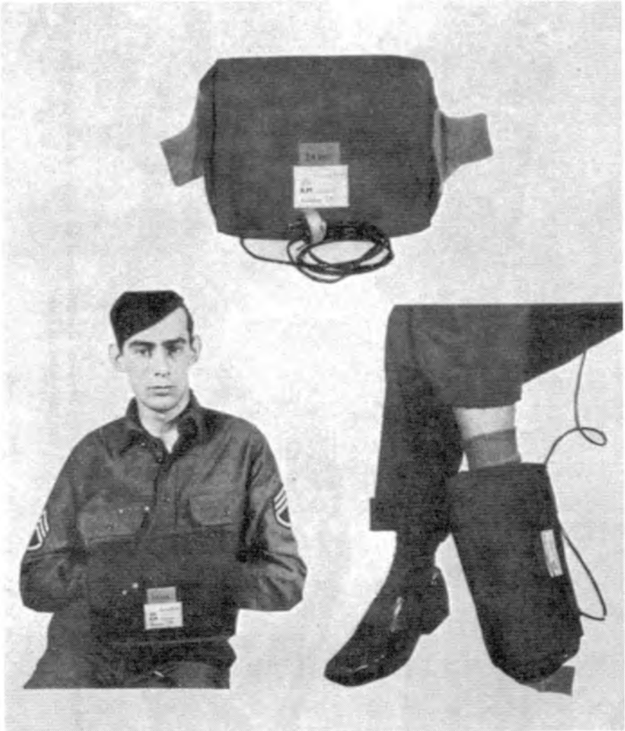
The electrically-heated muff shown here was developed by the Medical Department of the Eighth Air Force after much experimentation and service-testing. A number of prototypes were designed before a satisfactory one was finally developed.
