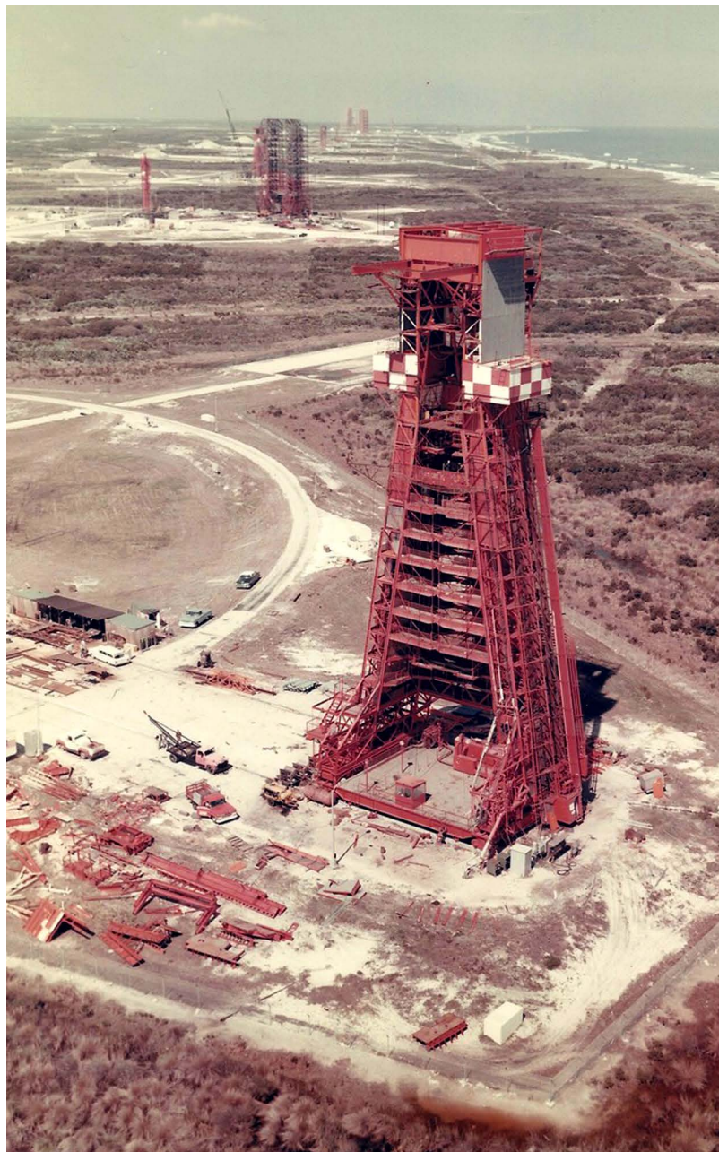
Fig. 8. LC-12 with its Mobile Service Tower, 28 February 1963. (Photo courtesy of John Hilliard)
