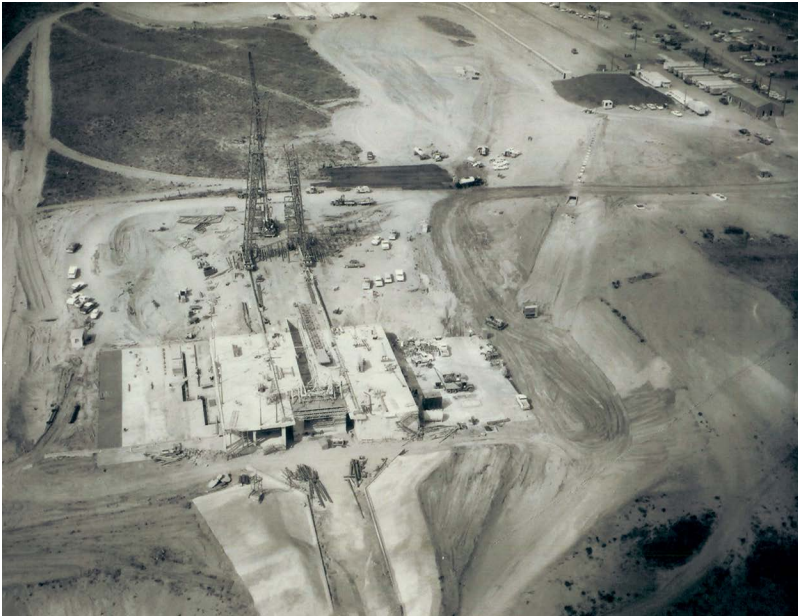
Fig. 6. Point Arguello Launch Complex (PALC) 1-2 (SLC-3E) under construction, 3 November 1959. (Photo courtesy of John Hilliard)
