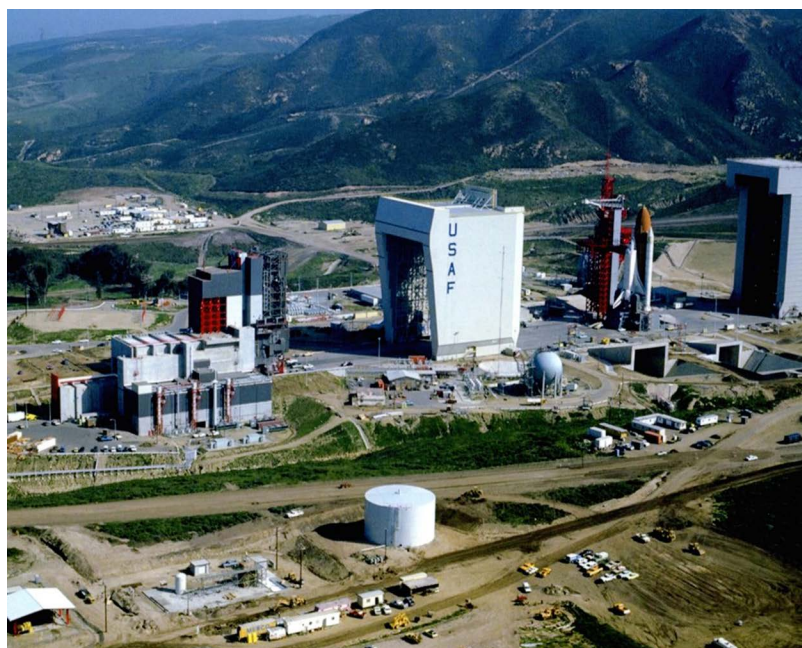
Fig. 15. This aerial view shows Vandenberg AFB’s Space Launch Complex (SLC) 6 from the south, with the shuttle Enterprise on the pad, October 1985. (Photo courtesy of John Hilliard)
