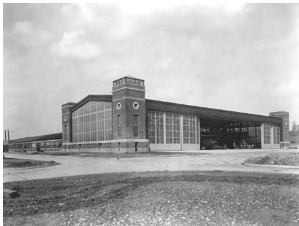
Building 31, Wright Field Assembly Hangar, with control tower atop southwest corner
