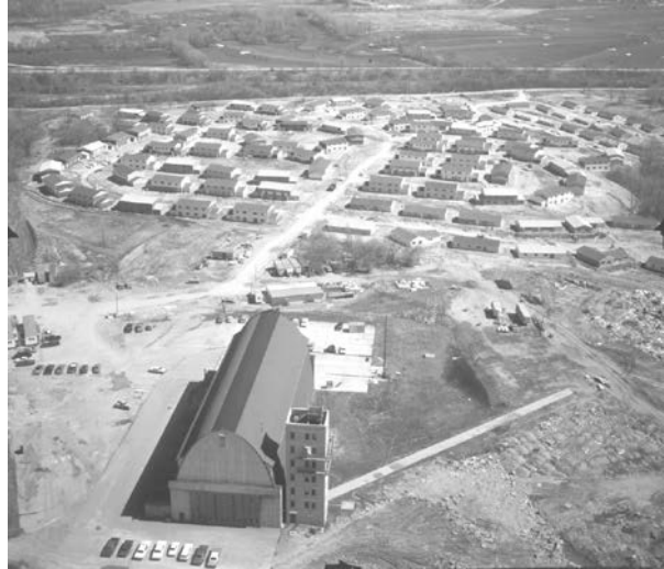
Woodland Hills housing complex under construction
