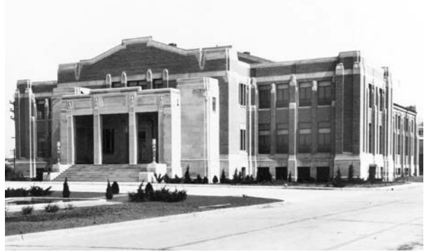
Building 12, Technical Data Library and Museum
