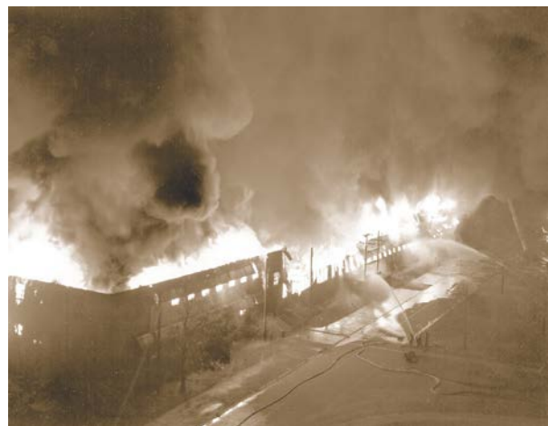
A tragic November 21, 1961 fire destroyed Building 262A, the AFLC Annex, and took the lives of two base firefighters
