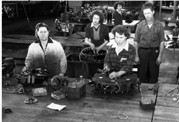
Civilian employees overhaul aircraft engines at Patterson Field
