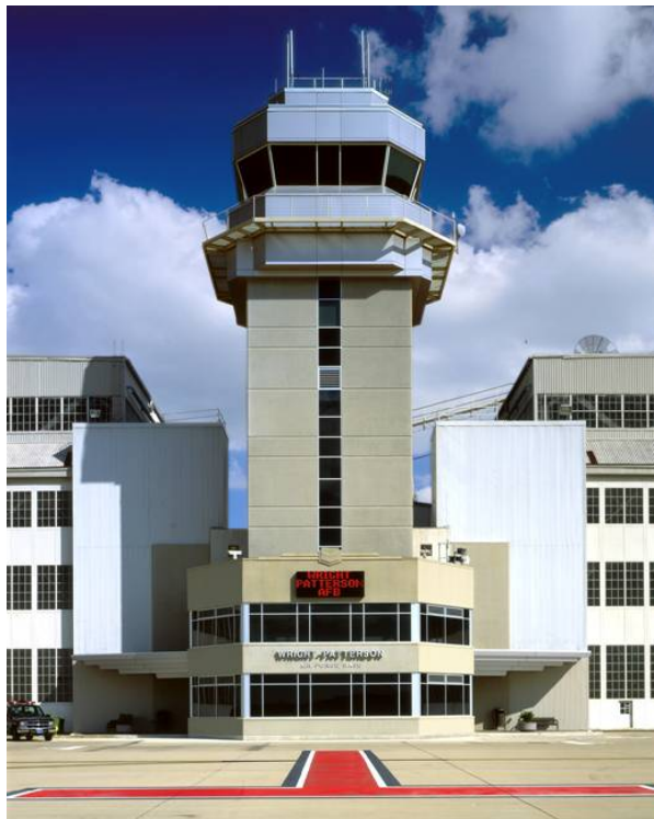
Wright-Patterson's new control tower, 2003
