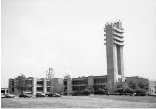
New Fuels and Lubrication Laboratory (Building 490)
