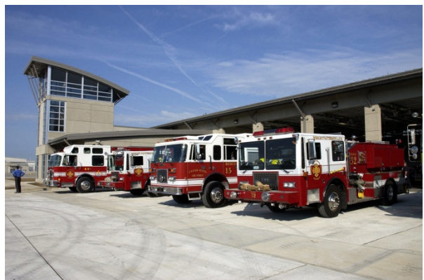
Wright-Patterson's new consolidated fire and crash rescue station
