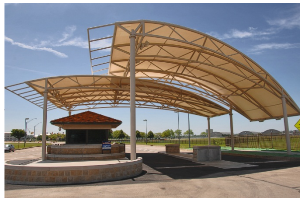
Gate 1B with its new canopy
