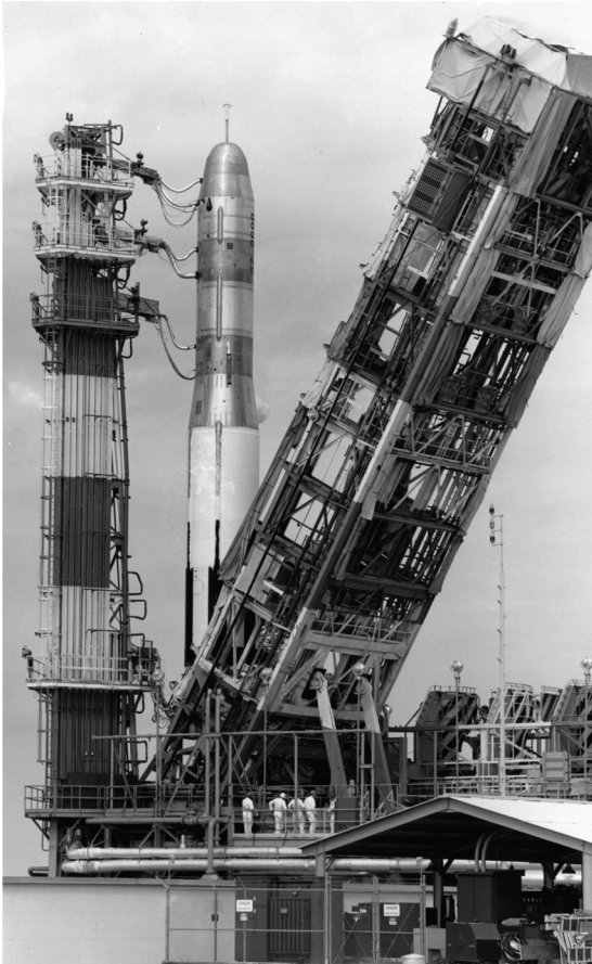
The erector is lowered away from a Martin SM-68 Titan ICBM prior to launching from Cape Canaveral Missile Test Annex.
