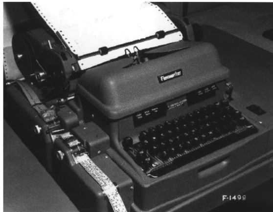
The Flexowriter, a SAGE input- output device.
