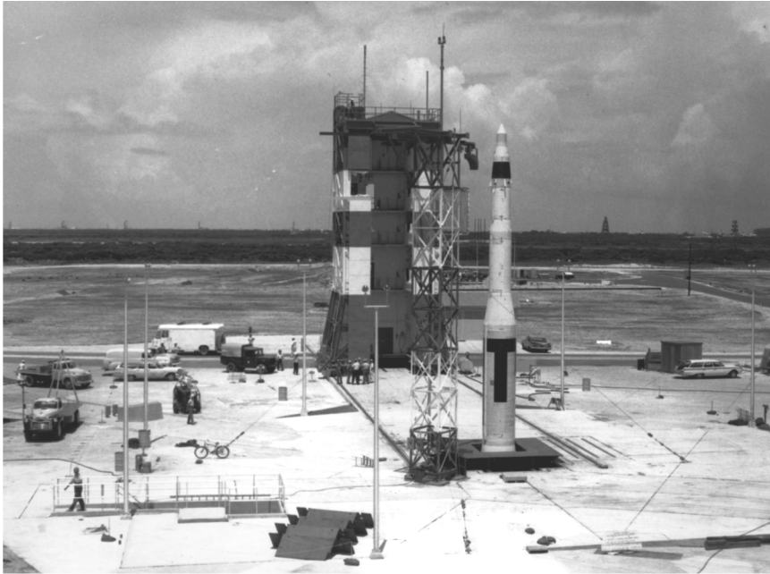
One of the pads at the Air Force Missile Test Center from which three-stage, solid-fuel-propelled Minuteman ICBMs were launched in the missile's development program.
