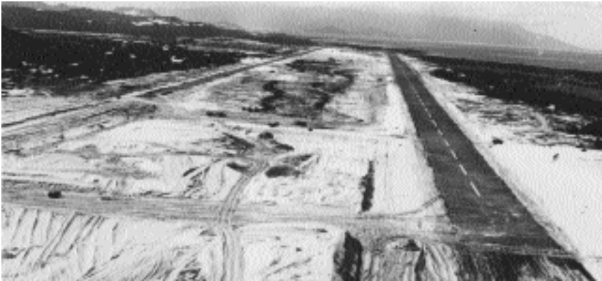
Runway construction at Cam Ranh Bay.
