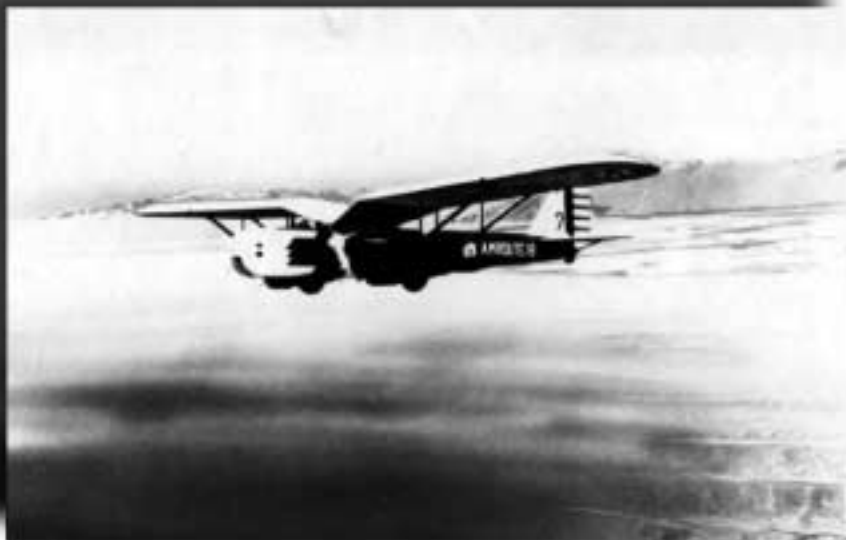
The Douglas B-7, designed as a fast day bomber, had fabric-covered wings, an all-metal fuselage, and hydraulically operated retractable landing gear. It flew airmail over the Salt Lake City–Oakland route in early 1934.
