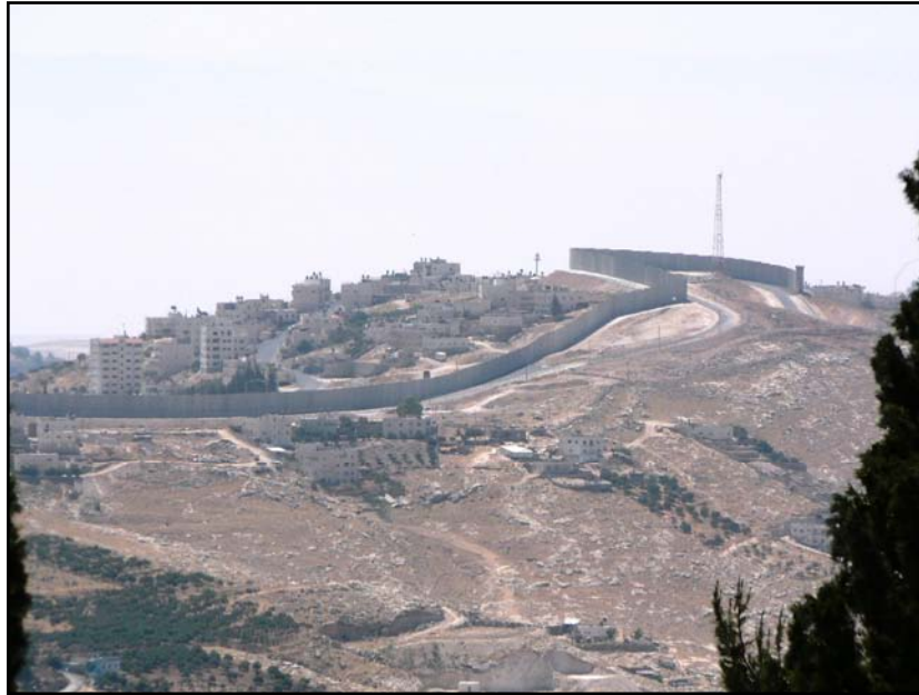
Figure 16. Security fence in Jerusalem viewed from the Old City (Larsen)
