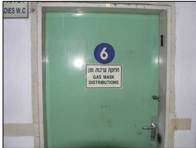
Figure 17. Protected space in basement of Tel Aviv Hilton Hotel (Larsen)
