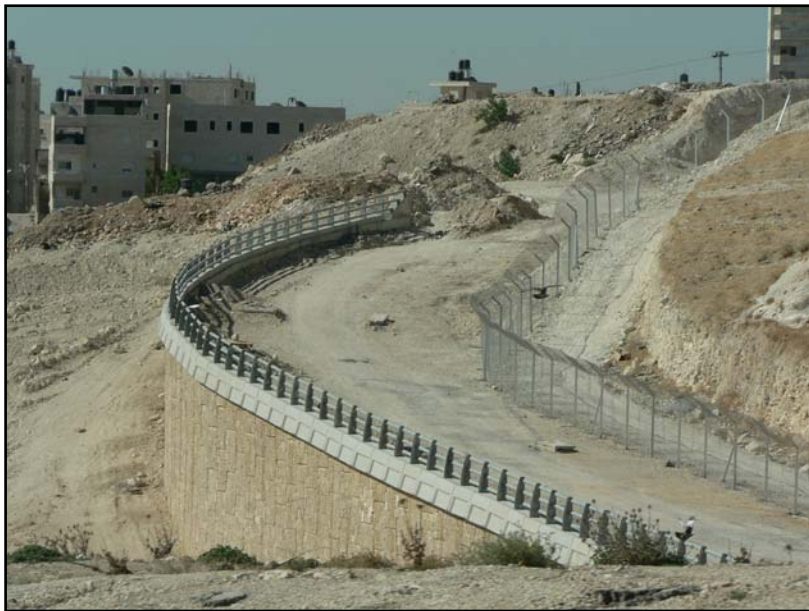
Figure 20. Security fence under construction, east side of Jerusalem (Larsen)
