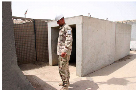
Figure 1.3. Protective Shelter Construction.
