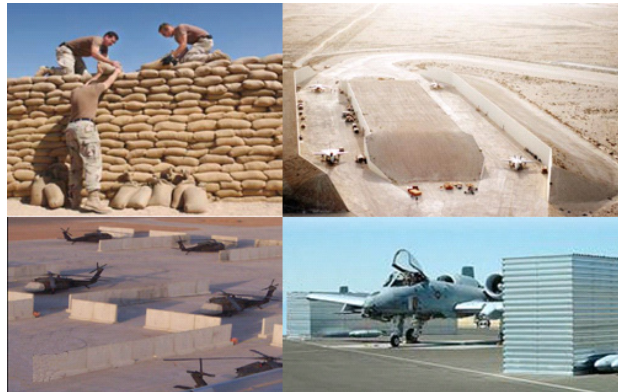
Figure 5.1. Various Types of Revetments.
