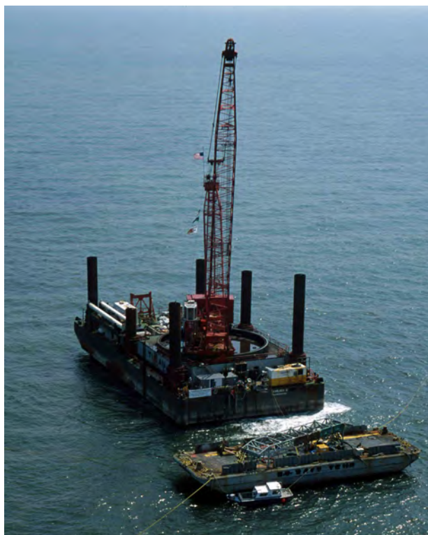
Figure 10.7. Karlissa-B in place over the site along with the supply barge, which housed the dredge pumps. The truss prior to installation is visible on the supply barge. Suction piles had already been placed on the sea floor. (Photo by Cramer Gallimore, courtesy of FOTH)
