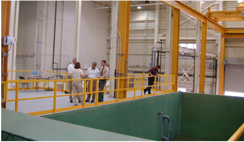
Figure 7.2. A view of the newly-constructed mezzanine looking down into the treatment tank. (Courtesy of FOTH)
