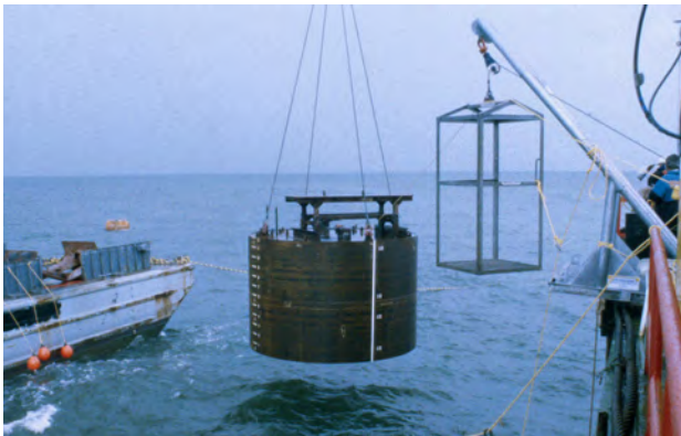
Figure 9.7. Fully rigged suction pile being lowered into the water. Depth markings can be seen down the side of the pile wall at left. (Courtesy of FOTH)
