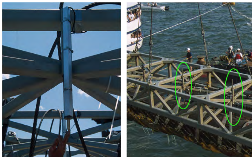
Figure 9.12. Linear variable displacement transducers (LVDTs), left, were planned for monitoring any longitudinal displacement of the hull. Two LVDTs were replaced with rods for manual monitoring (right). (Courtesy of FOTH)
