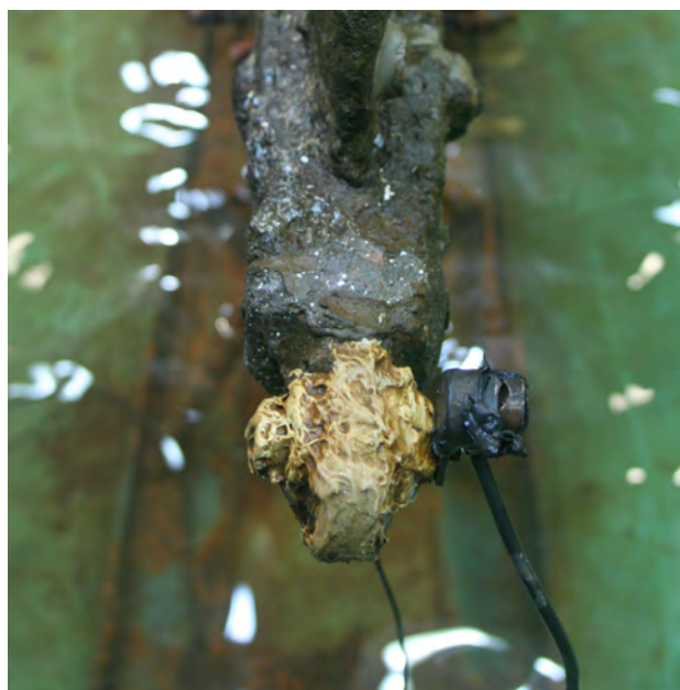
Figure 7.4. A negative cable for the impressed current system was attached to the bow where the spar was once mounted. A coating of epoxy protected the exposed metal. (Photo by H. G. Brown, NHHHC)
