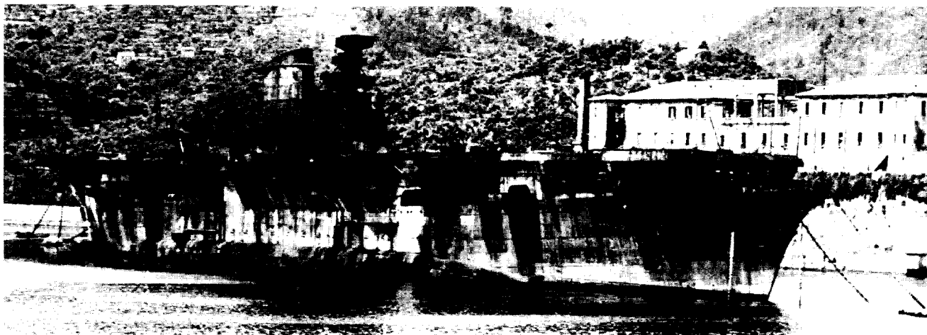
AQUILA, an attempt by the Italian Navy to convert a liner into an aircraft carrier, is shown as she appeared at LA Spezia in June 1951.
