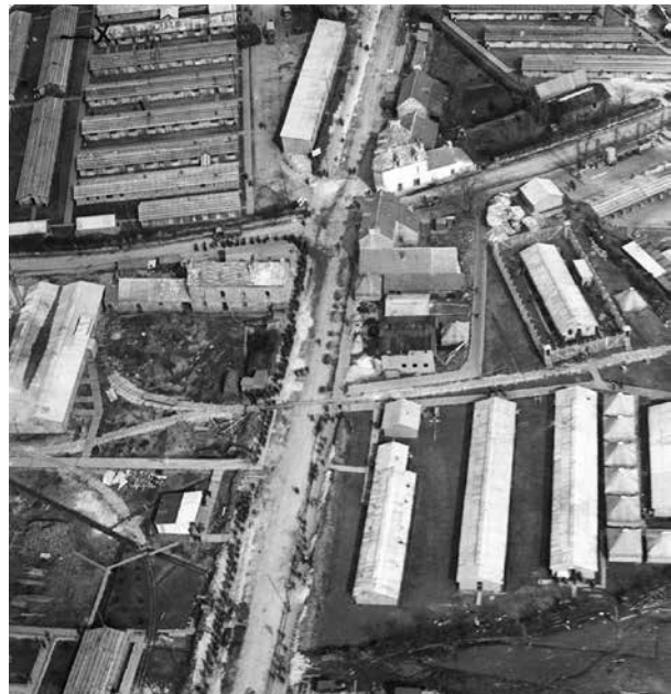
Aerial photograph of only a portion of Camp Pontanezen, near Brest, France.
