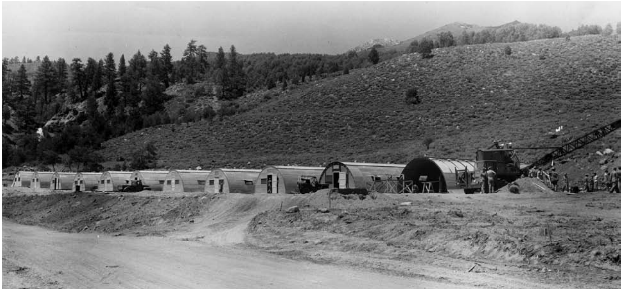
Marines of 7th Engineer Battalion, Force Troops Pacific, construct Quonset huts at Pickel Meadow base camp, October, 1952.
