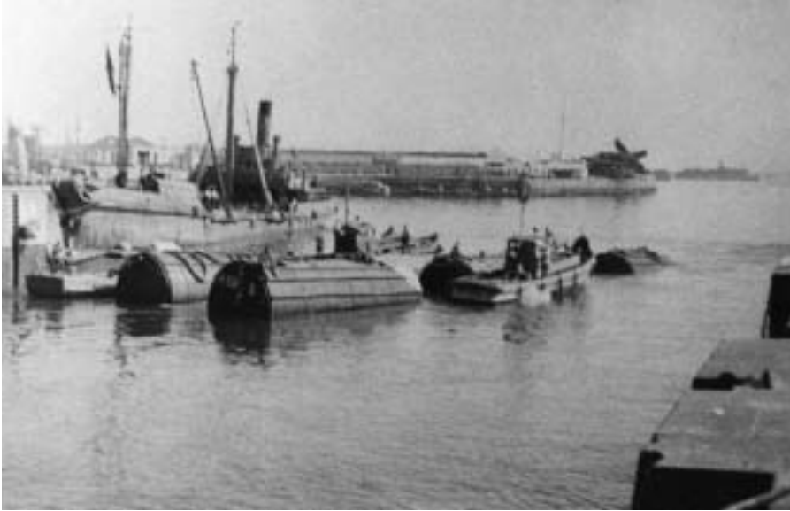
Supported by pontoons, a submerged tug is towed out of Le Havre under the direction of Lieutenant Frank N. Oberle. Photo courtesy Vice Admiral Bernard E. Manseau.
