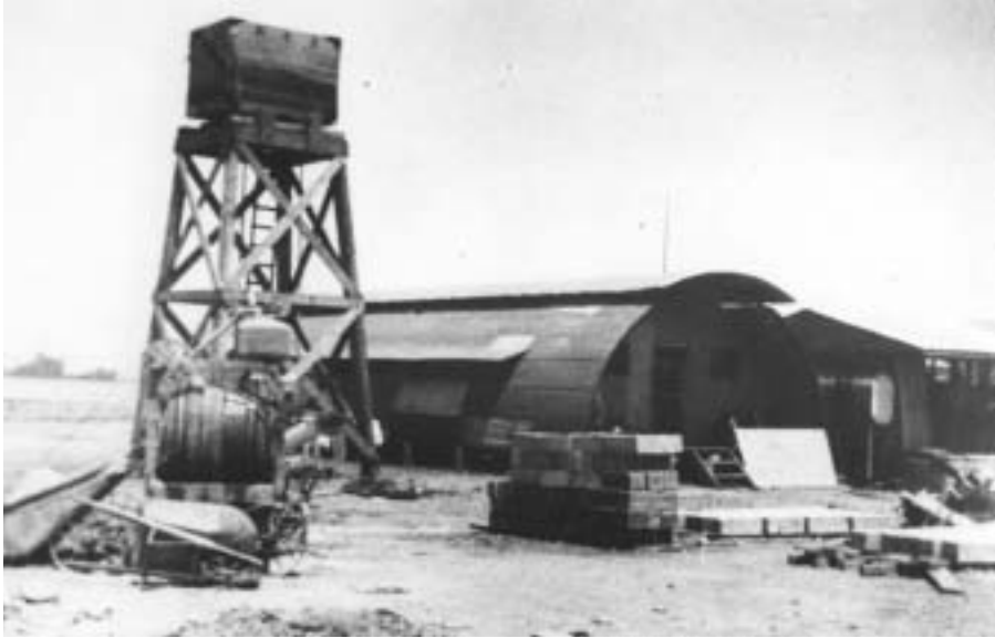
Accommodations for those clearing Manila harbor were far from grand. This Quonset hut served as Commodore Sullivan's quarters. Photo courtesy Vice Admiral Bernard E. Manseau.
