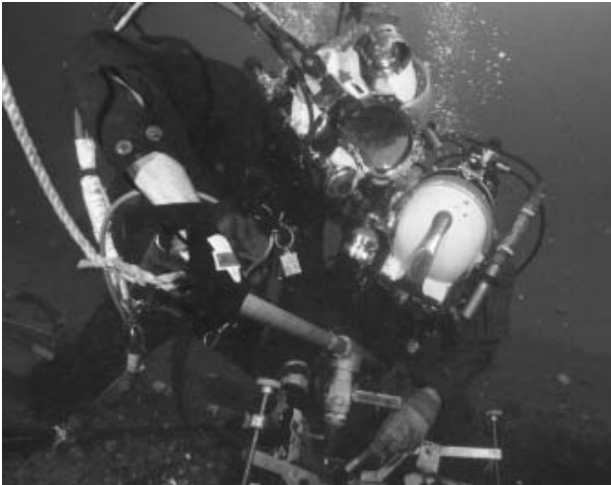
Navy divers hot tapping Mississinewa's tanks.
