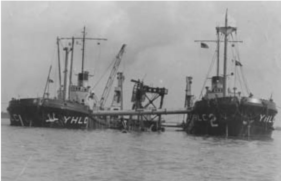
The heavy lift ships Crilley and Crandall , held apart by large spreader bars, lift the dredge Sandpumper in the My Tho River, Vietnam.
