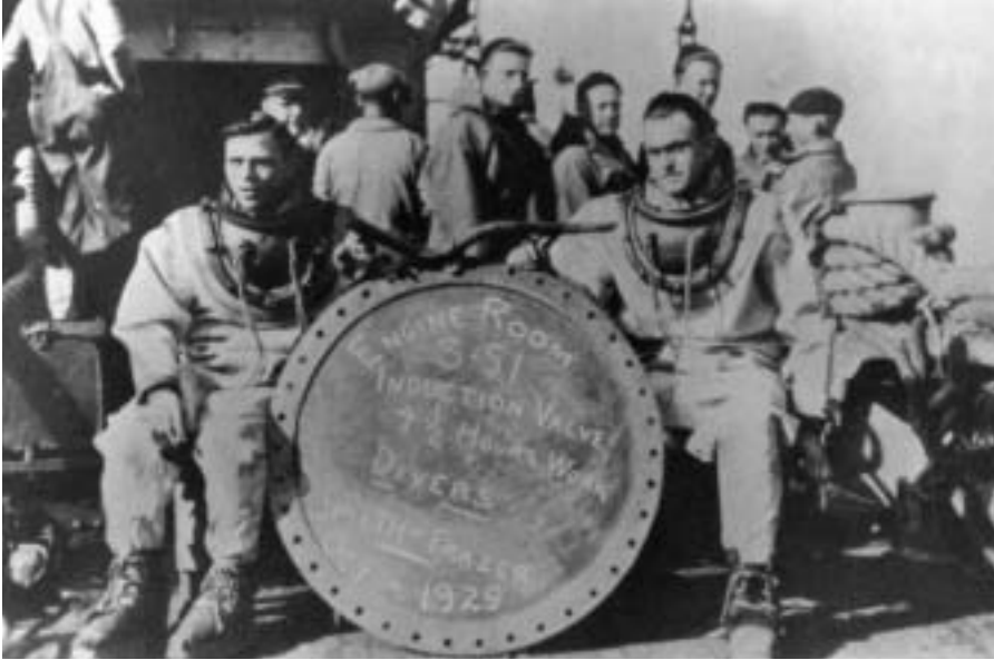
Divers Smith and Frazier display the induction valve that they removed from the submarine S-51 after 4½ hours work on the bottom.
