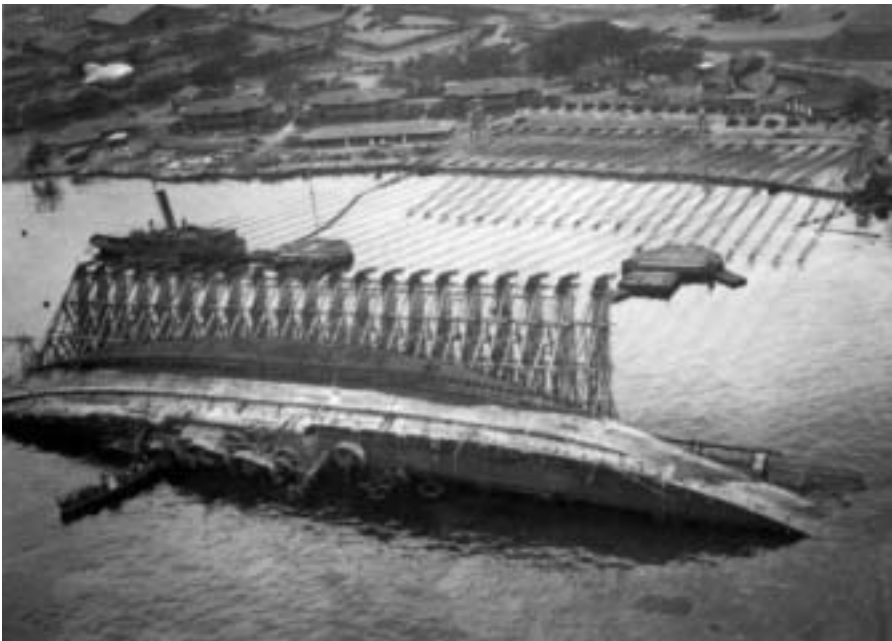
The capsized battleship Oklahoma was righted by building headframes on her side and pulling with purchases and winches mounted ashore on Ford Island.
