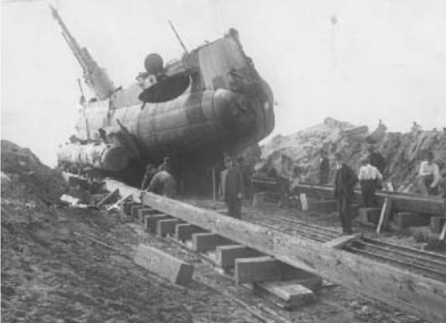
H-3 is moved overland on wooden tracks for launching in the calm waters of Humboldt Bay.
