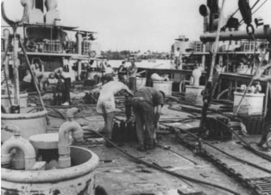
Salvors work “head down, backside up” on deck of their British lift craft during the Paul Bert salvage. The heavy pieces on deck are Bullivant clamps used to clamp the lift wires together. Unlaidd manila line in the clamps absorb grease squeezed from the wire and prevent slippage. The clamps are tightened by large pneumatic wrenches called “windy spanners.” Photo courtesy Commander Billie L. Delanoy.
