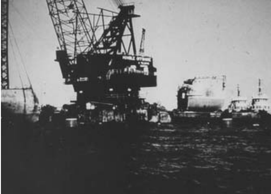
A 600-ton whirley crane lifts the stern section of the Corps of Engineers' dredge Mackenzie onto a waiting barge. The dredge's stacks still protrude from the water.
