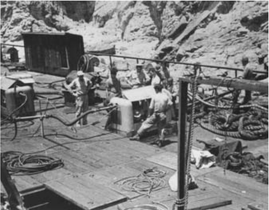
Salvors from the salvage ship Grasp , assisted by a Korean boy, study a recalcitrant air compressor used to blow air into the tanks of the South Korean LST M-370.
