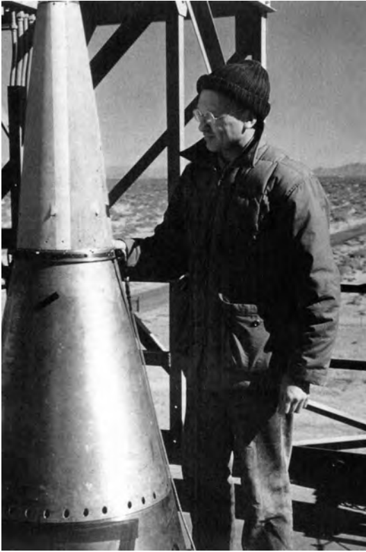
Sun Watcher. Dr. Richard Tousey, an optical scientist at NRL, examines an instrument-laden nose cone before a V-2 launch at White Sands Missile Range in New Mexico. (NRL photo newimage0(4))
