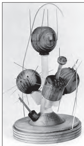
Buckshot. Three portraits, including an artist's rendition and a wooden model, of an ambitious and ill-fated attempt on January 24, 1962, by NRL, along with the Army, Navy, and Air Force, to launch five satellites with a single booster. The cluster was named Composite I, but the nickname Buckshot became its more familiar moniker. (NRL photos 60321.jpg, 60325.jpg, and 60327(2).jpg)
