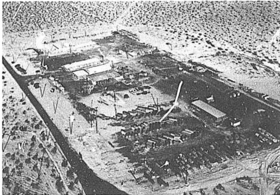
Salt Wells Pilot Plant under construction, July 1945.
