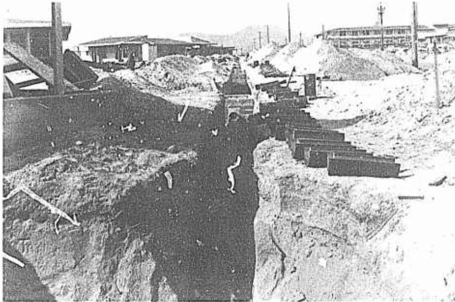
Typical construction at NOIS showing one of many inconveniences—the open trench!
