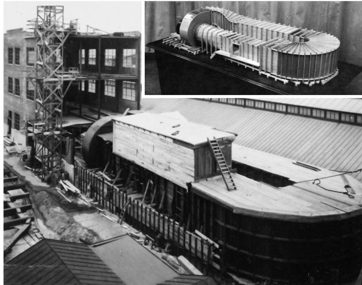
Figure 9. Wind Tunnel under construction (c1913) for the Navy’s Aerodynamics Laboratory, Washington Navy Yard (inset shows replica model).
