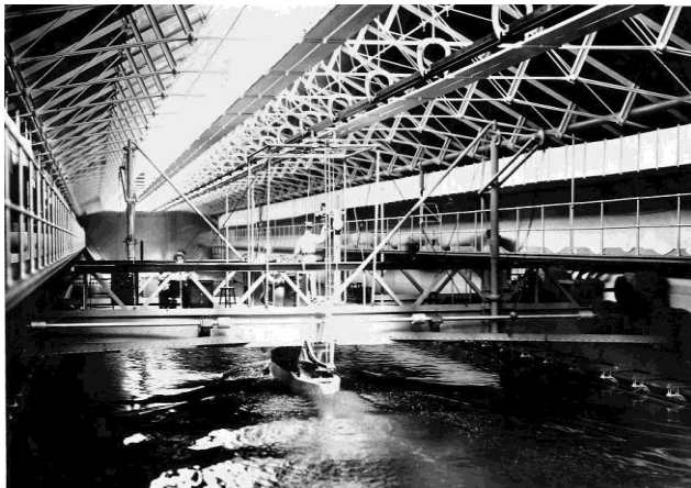
Figure 2. The Experimental Model Basin (EMB), was established in 1898 at the Washington Navy Yard, for the testing of ship hulls.
