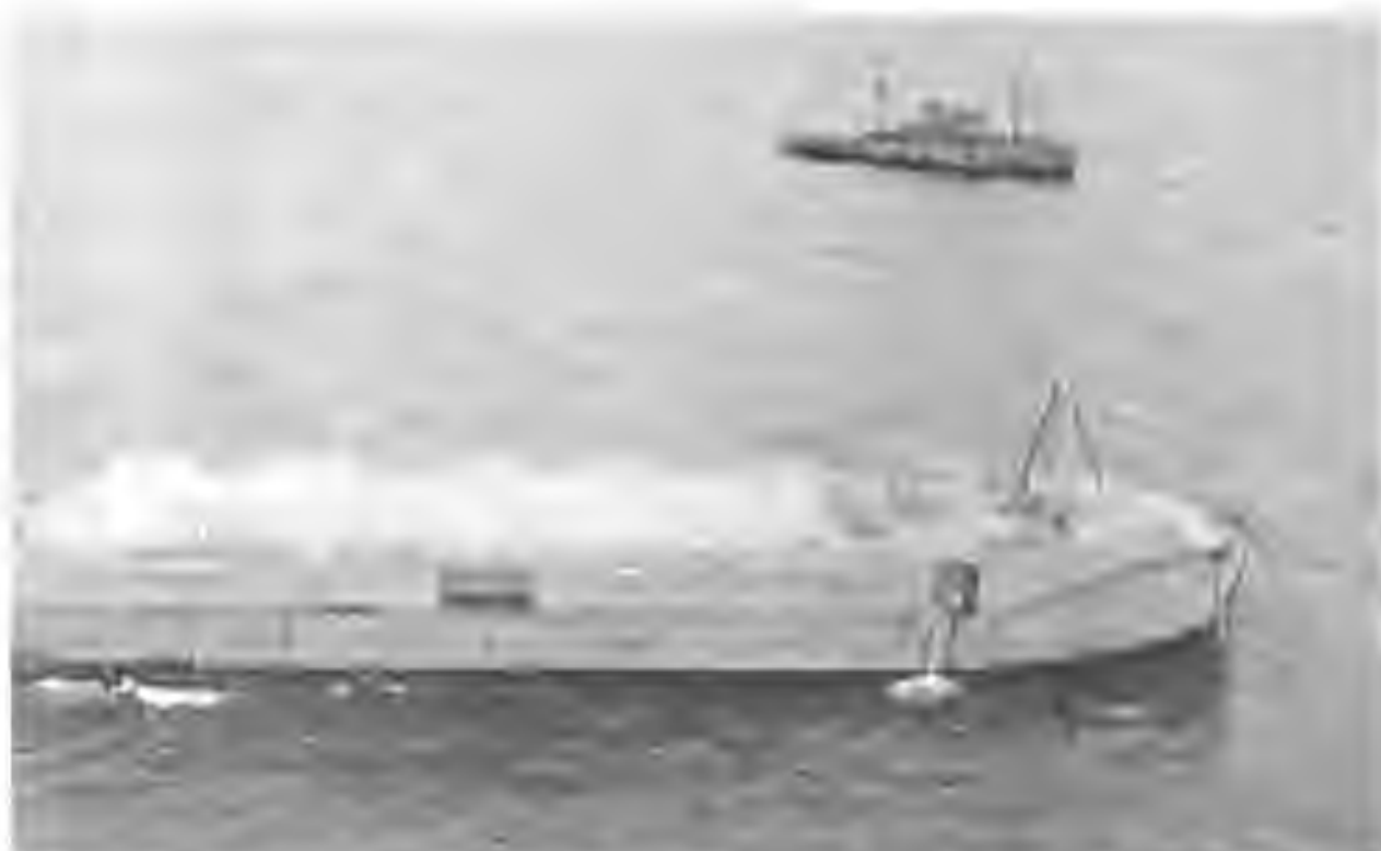
Figure 65. Flush-deck steel barge with washdown system; USS Bolster (ARS-30) is in background, HARDTACK .
