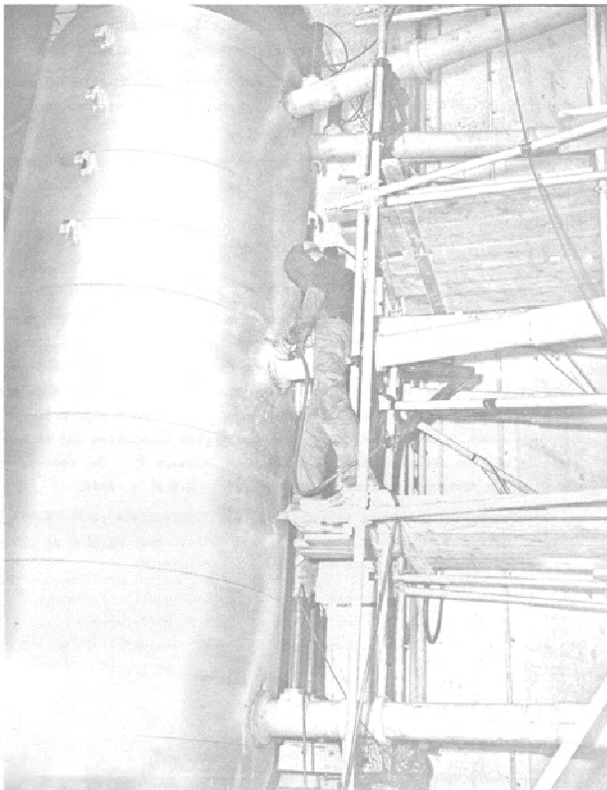
Figure 19. Welder attaching hot-spot tubes to IVY, MIKE device.
