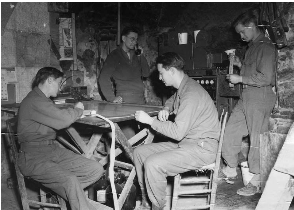
15th Field Artillery Observation Battalion soldiers operating sound-ranging equipment in Italy in March 1945
