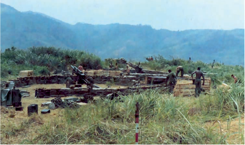
Artillerymen of Battery A, 6th Battalion, 33d Artillery, build protective sandbag walls around their 105-mm. howitzers.
