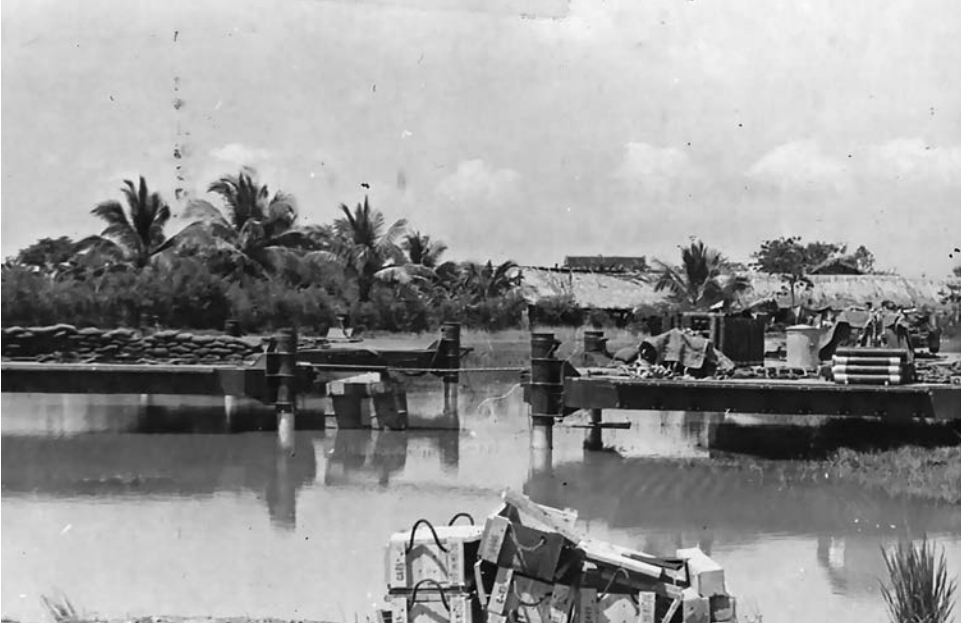
Airmobile artillery platforms were designed to overcome the swampy conditions in the Mekong Delta.
