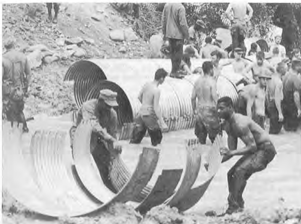
MARINE ENGINEERS IN VIETNAM. Men of the 11th Engineer Battalion move culverts into place in a mountain stream during "Operation Pegasus."
