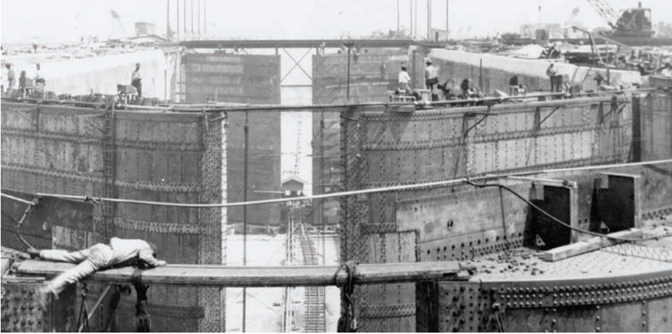
Locks of the Panama Canal under construction
