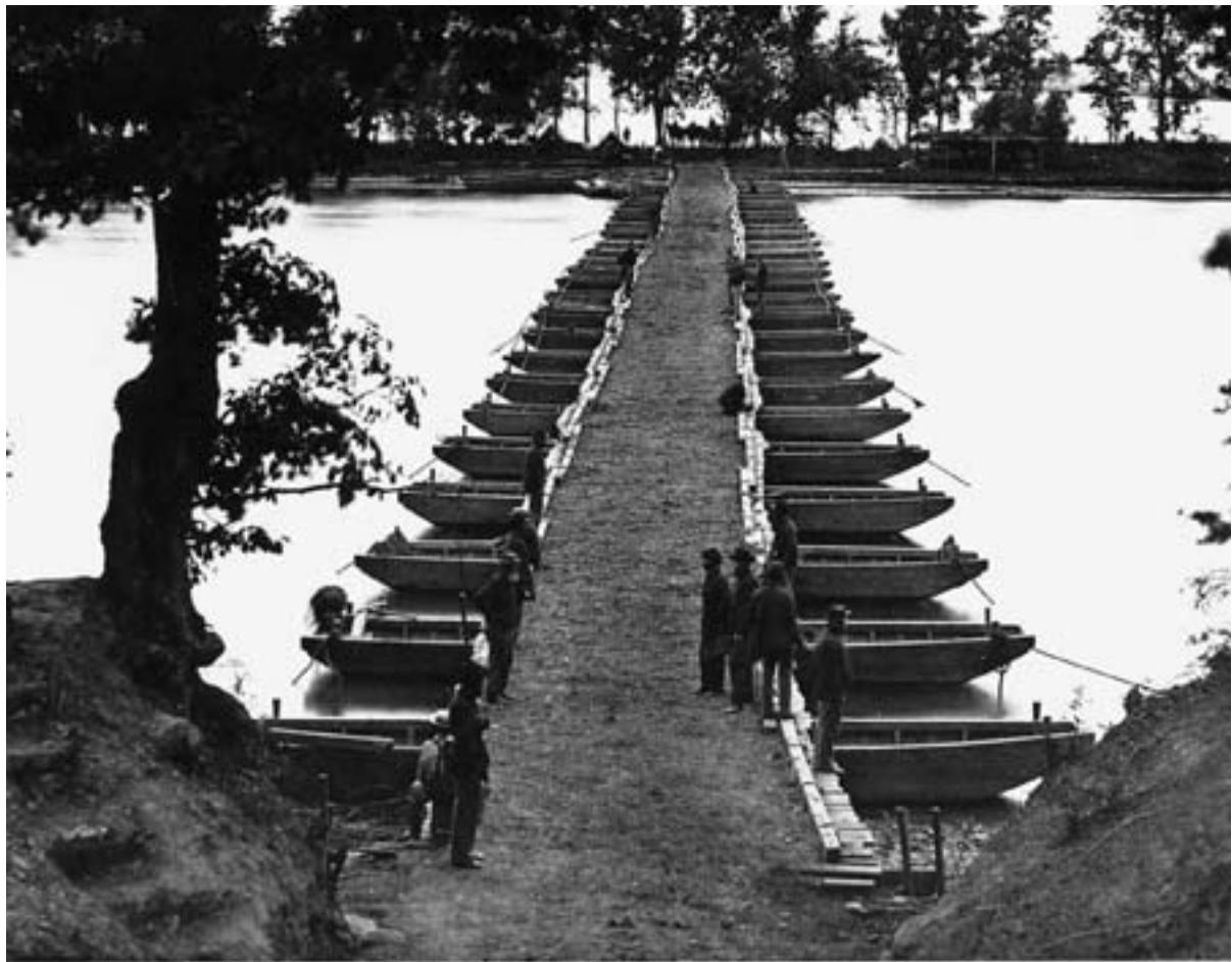
*A Civil War Pontoon Bridge, c. 1863. Whether assigned to combat or construction duties, NCOs of the Corps of Engineers enable the Army to reach its destination and support the troops on the way.*
