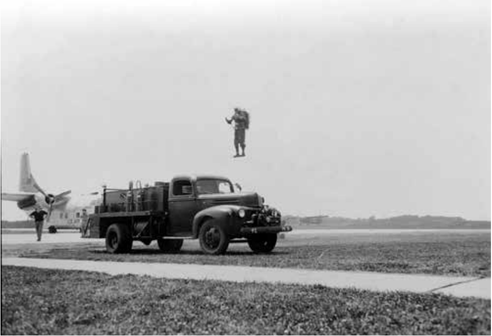
At Fort Eustis, Virginia, test engineer Harold M. Graham demonstrates a new twin-jet rocket-propulsion system, developed by the Bell Aerosystem Company. ( U.S. Army, National Archives Still Picture Branch )
