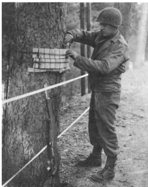
PLACING CHARGES TO DROP TREES across roadways.
