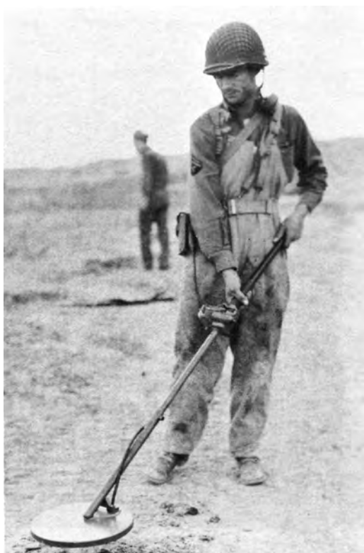
THE SCR-625 MINE DETECTOR in action on a Tunisian road.
