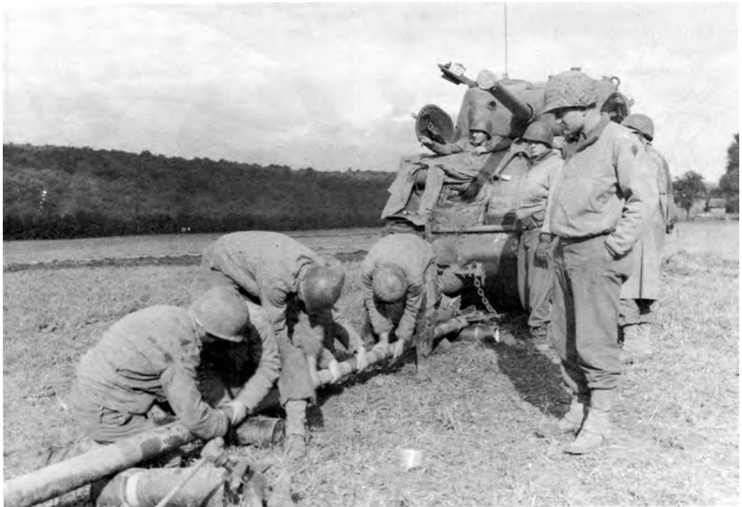
ENGINEERS ASSEMBLE AN EXPLOSIVE-LADEN "SNAKE" to clear a path in a minefield.
