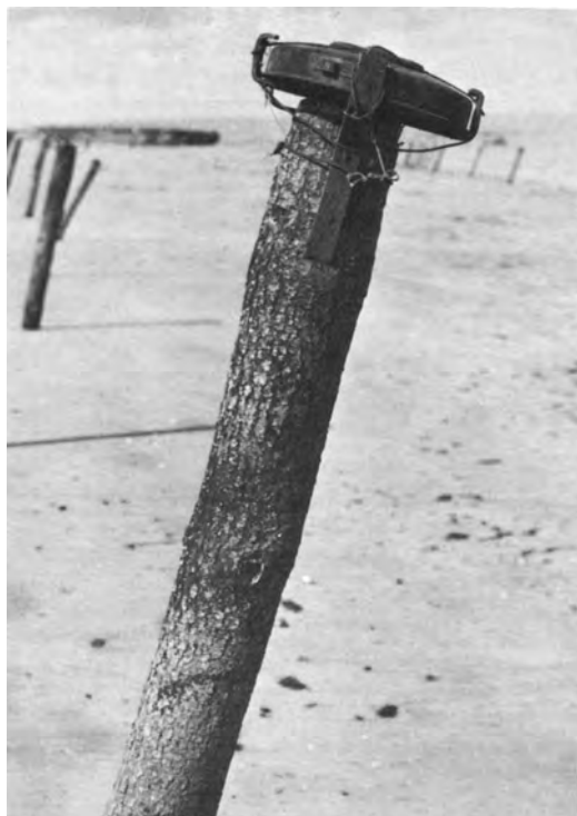
TELLER MINE ATOP A STAKE emplaced to impale landing craft on Utah Beach.
