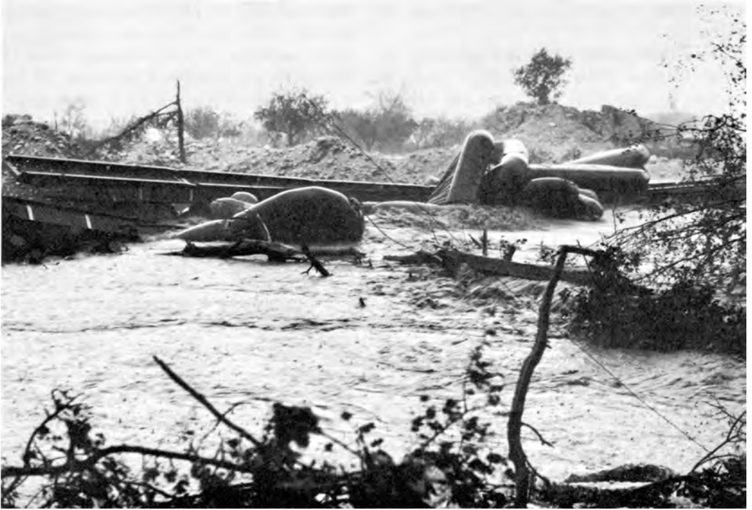
WRECKED M2 FLOATING TREADWAY ON THE VOLTURNO
