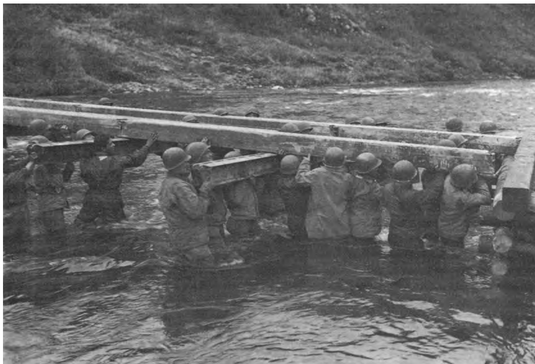
SEVENTH ARMY ENGINEERS INSTALL A BRIDGE ON THE ILL RIVER
