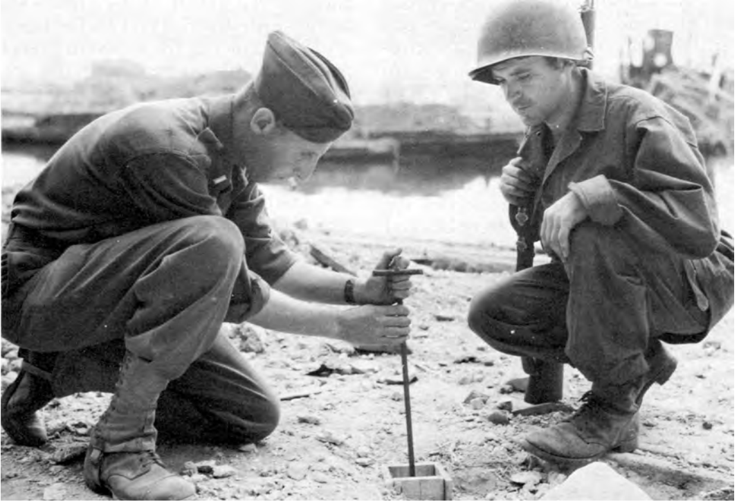
ENGINEER OFFICER PROBES FOR EXPLOSIVE CHARGE AT MARSEILLE
