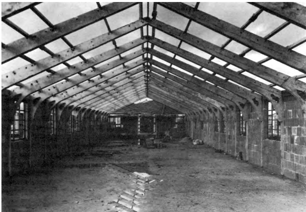
HOSPITAL CONSTRUCTION EMPLOYING PREFABRICATED CONCRETE ROOF TRUSSES
