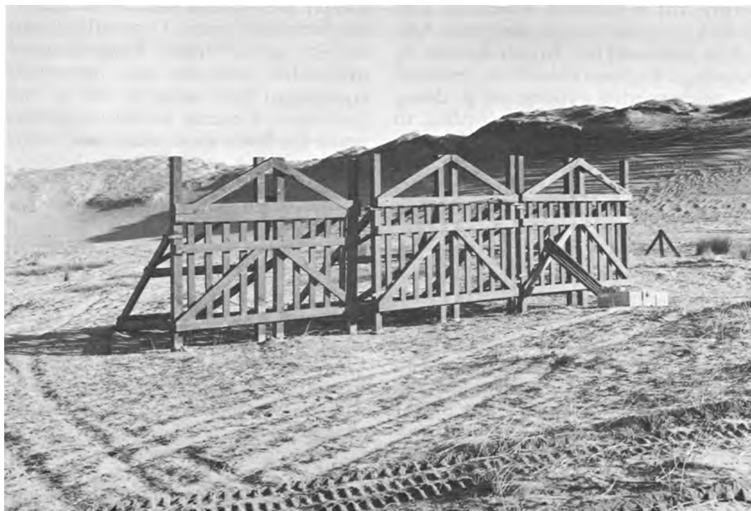
MODELS OF BELGIAN GATES, patterned after German obstacles on Normandy beaches.
