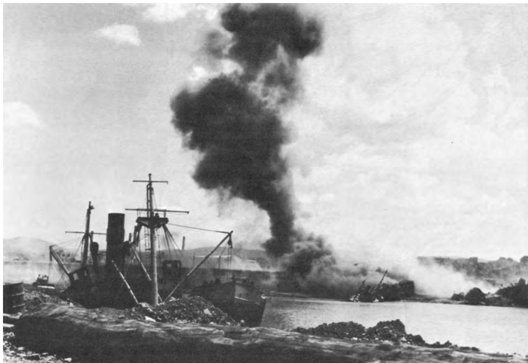
BLASTING OBSTACLES AT CIVITAVECCHIA, JUNE 1944
