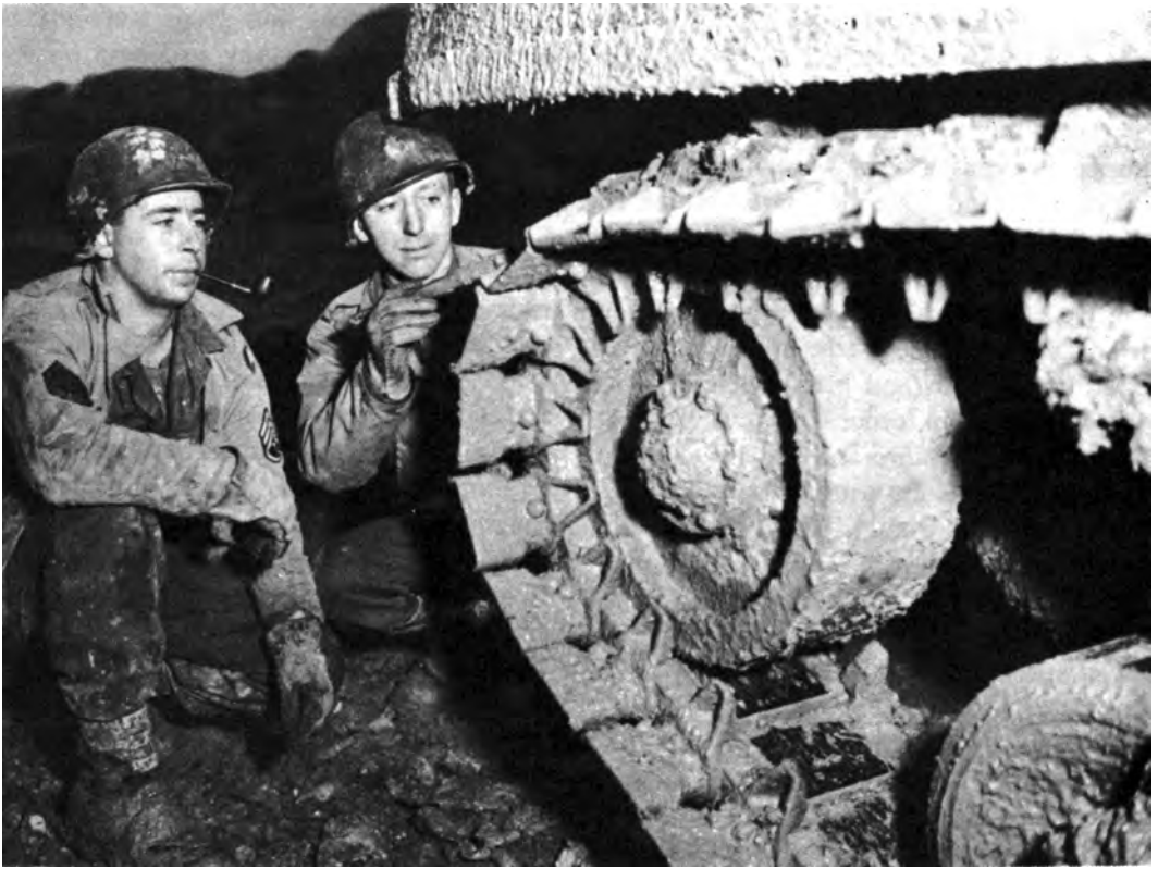
INSPECTING DUCKBILL EXTENSIONS ON TANK TRACKS
