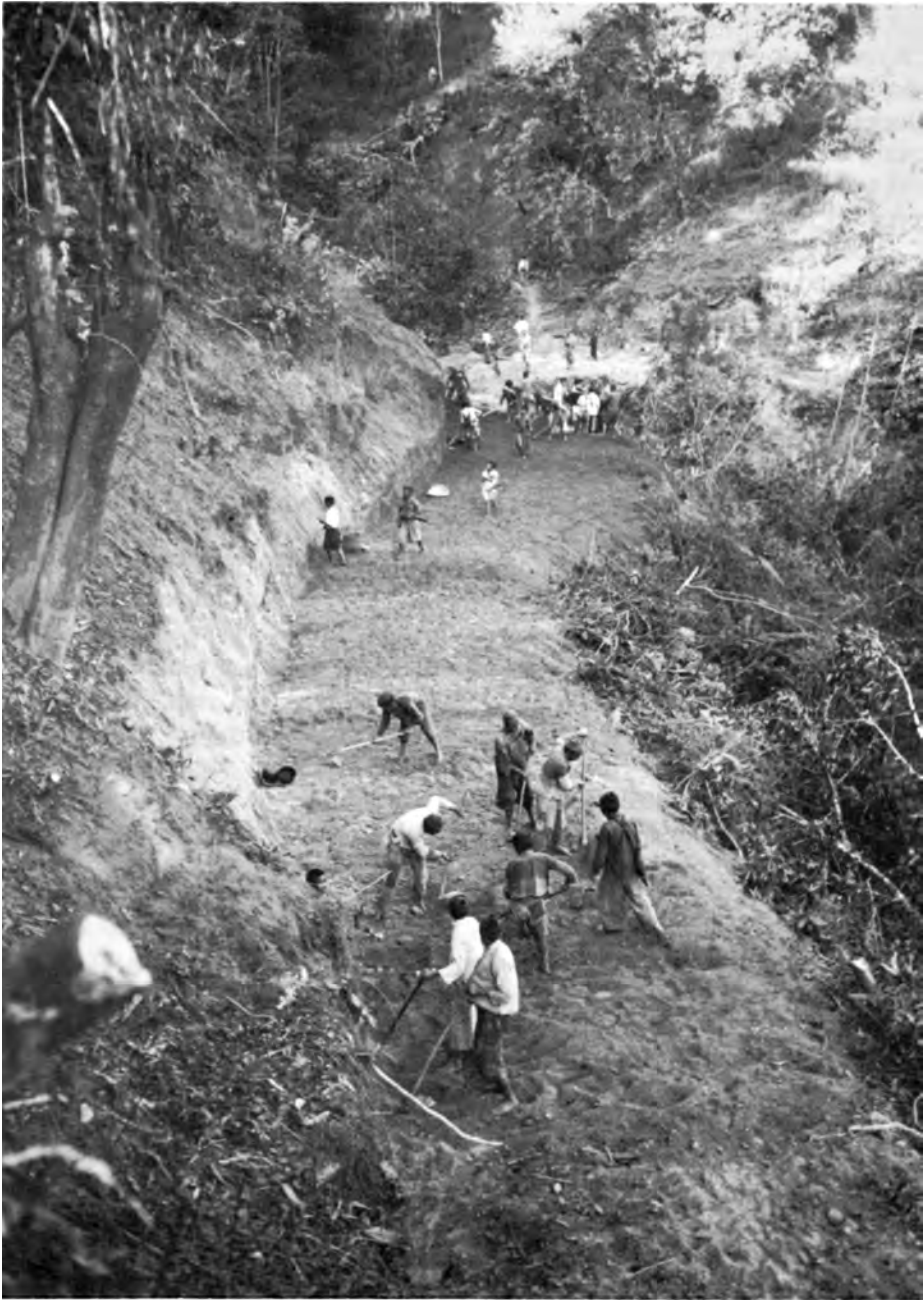
CHINESE COOLIES LEVELING A ROADBED for the Teng-chung cutoff route to Kunming.
