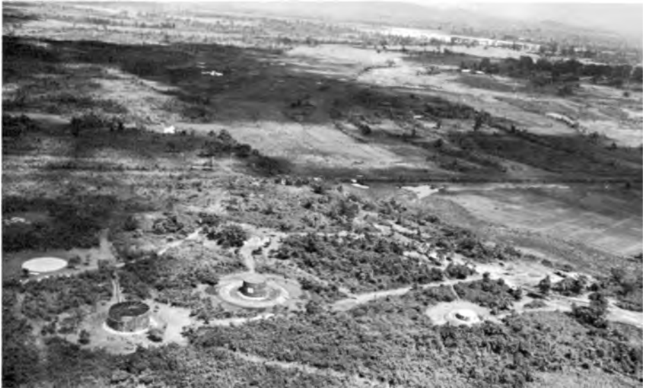
TANK FARM AT MYITKYINA. Gasoline delivered by pipeline was stored in these tanks until needed.
