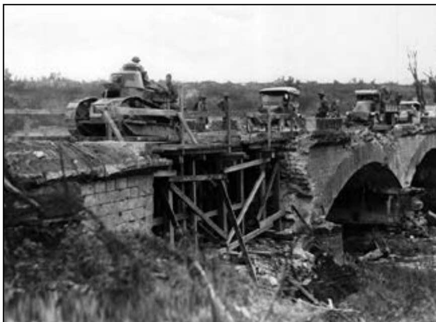
Figure 3.2. Renault FT tanks and other military vehicles cross a stone bridge repaired by Companies A and E, 103rd Engineers, 28th Division, near Beureuilles, Meuse, 28 September 1918. Courtesy of the US Army Engineer School.
