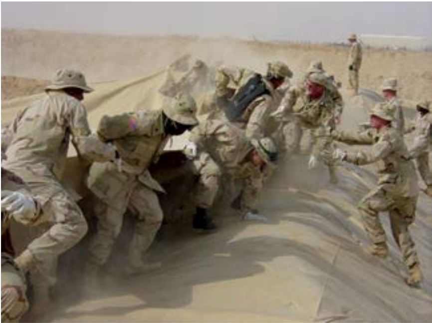
Figure 11.2. Bulk Fuel Tank Assemblies form the storage component of the Tactical Petroleum Terminals that connected the pipeline segments. When combat operations commenced, US forces had more than 4 million gallons of fuel in the TPTs. Photo courtesy of US Army Quartermaster Center and School.
