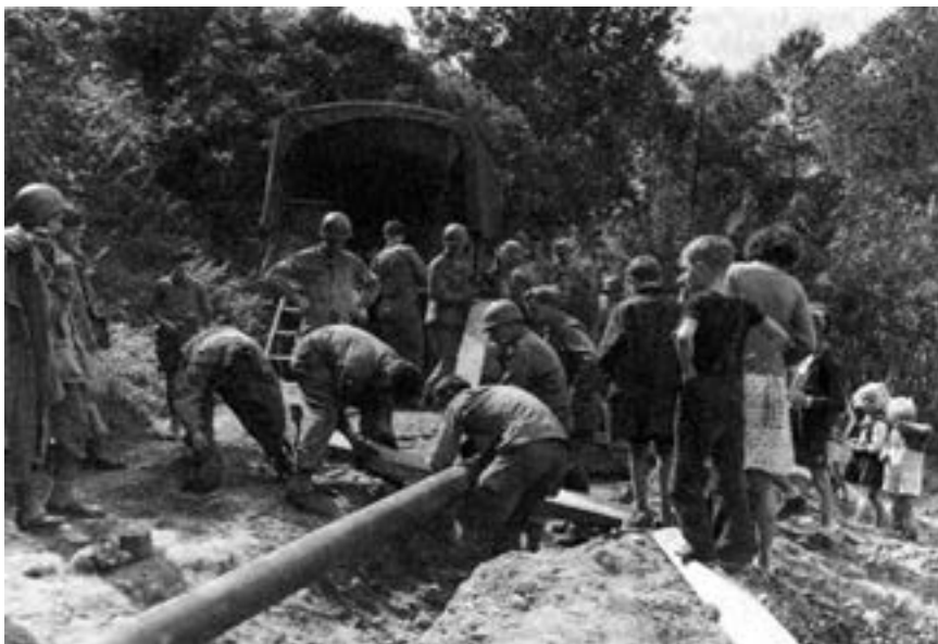
Figure 11.1. The World War II pipeline system consisted of steel pipe that required welding to connect the individual sections. The Army depended heavily on pipelines to move bulk fuel during the war. Photo courtesy of Army Signal Corps.
