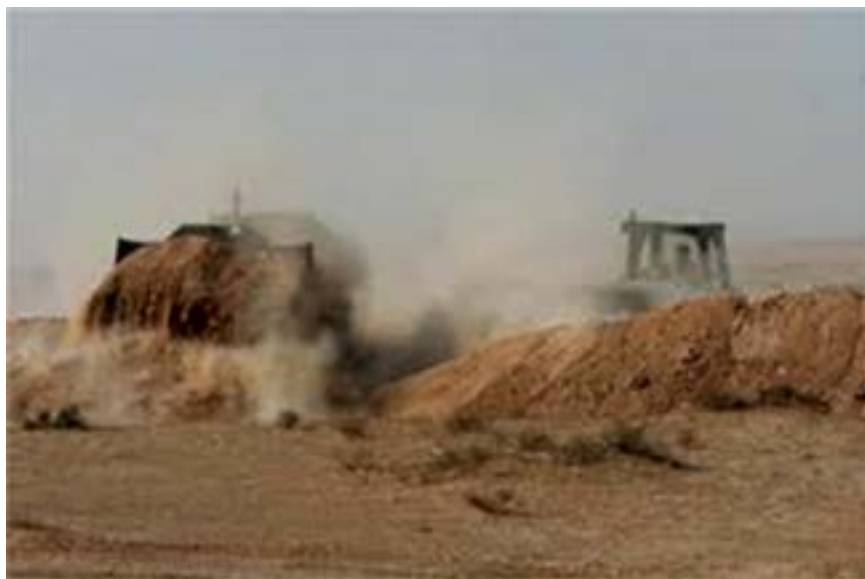
Figure 11.5. To prevent the damage to the pipeline caused by vehicles, engineers constructed 6-foot-high berms on both sides of the line. Ultimately, more than 130 miles of berms were erected. Photo courtesy of 416th Engineer Command.
