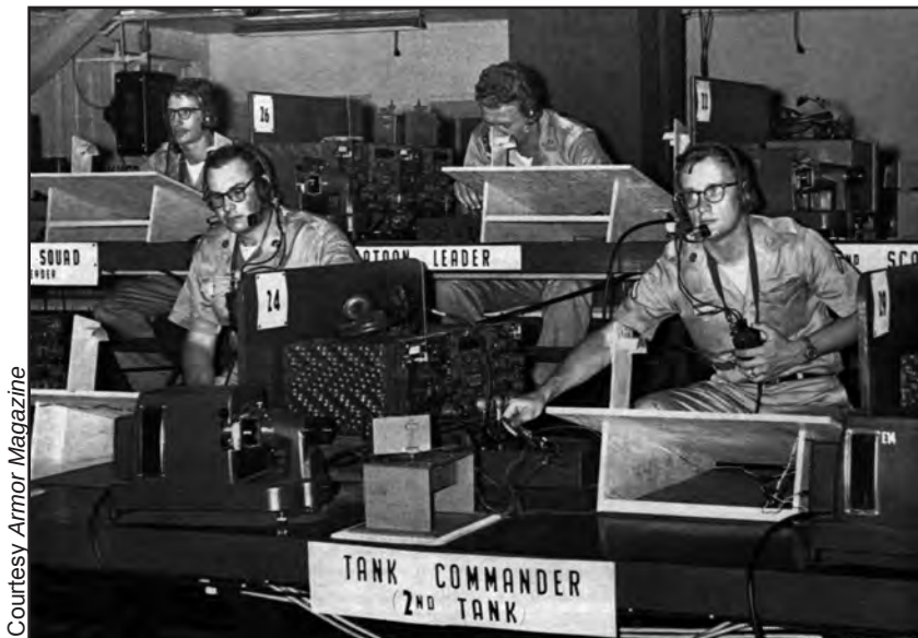
Figure 60. Armored cavalry trainer developed to improve the preparation of cavalry leaders through the integrated use of radios and movie projectors—the forerunner of computer-based simulators.
