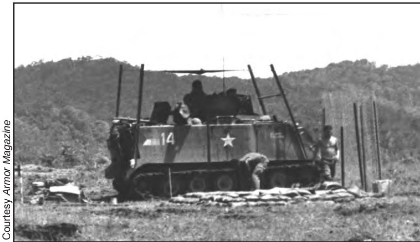
Figure 71. M113 behind chain link RPG screen intended to detonate prematurely incoming projectiles.
