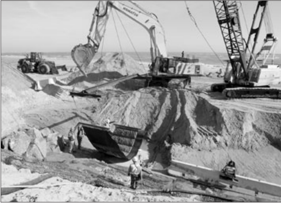
Placement of stone mat foundation for upgrading the Hereford Inlet Seawall, North Wildwood, N.J.
