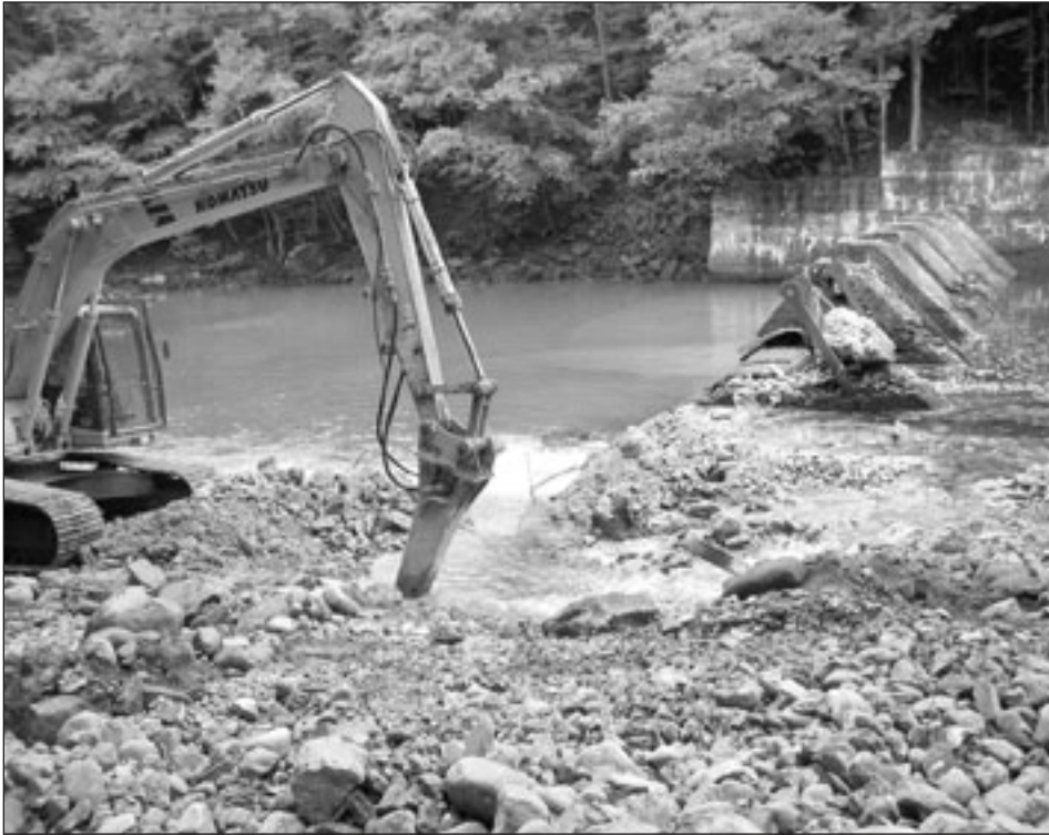
Removal of the old Cuddebackville Dam (above) and subsequent restored flow on the Neversink River (below)
