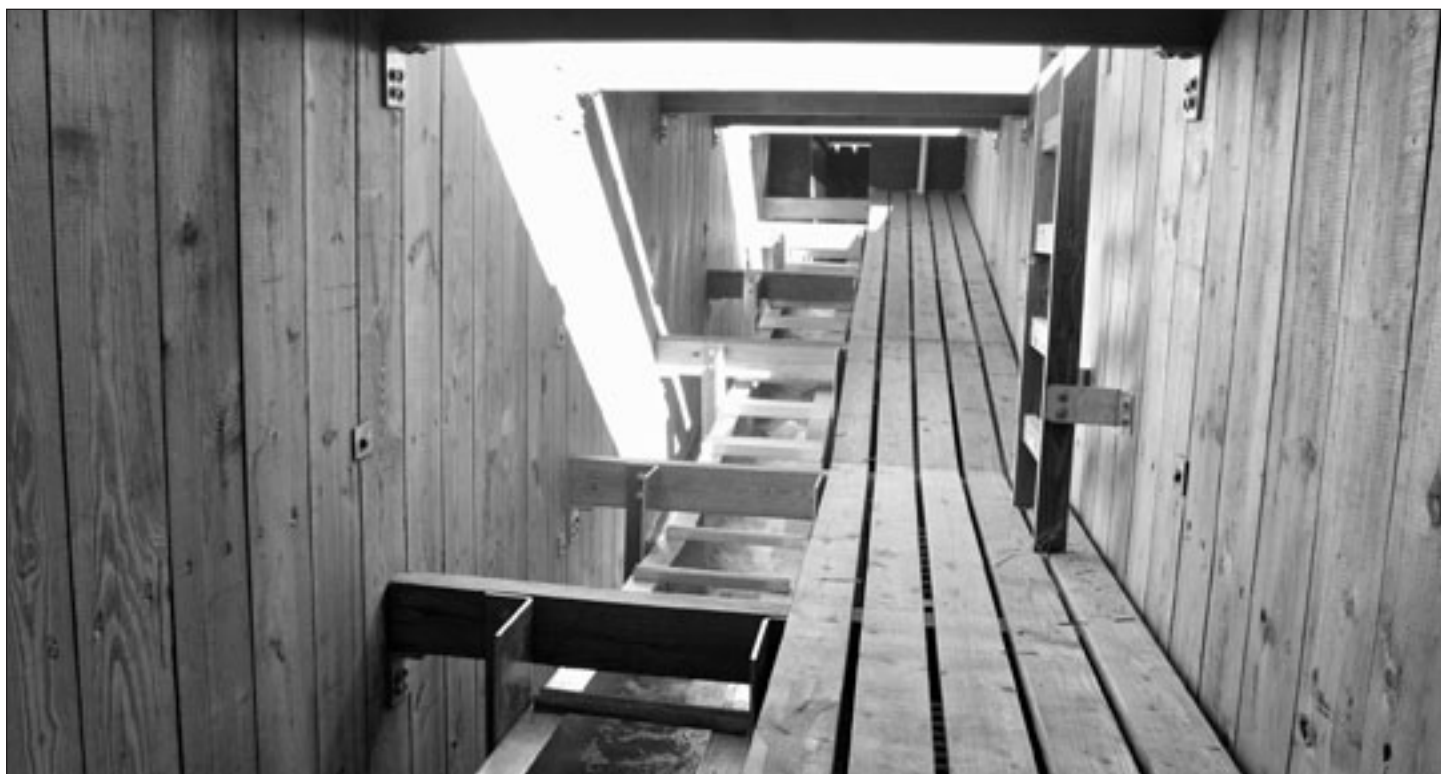
The Batsto River fishway restoration under construction (above) and an inside look at the removable wooden structures enclosing the fish ladders (below)
