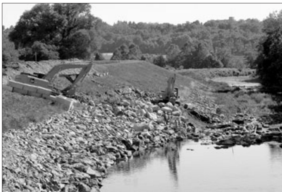
Repairs to a storm-damaged levee at Stroudsburg, Pa., under the Public Law 84-99 Rehabilitation & Inspection Program
