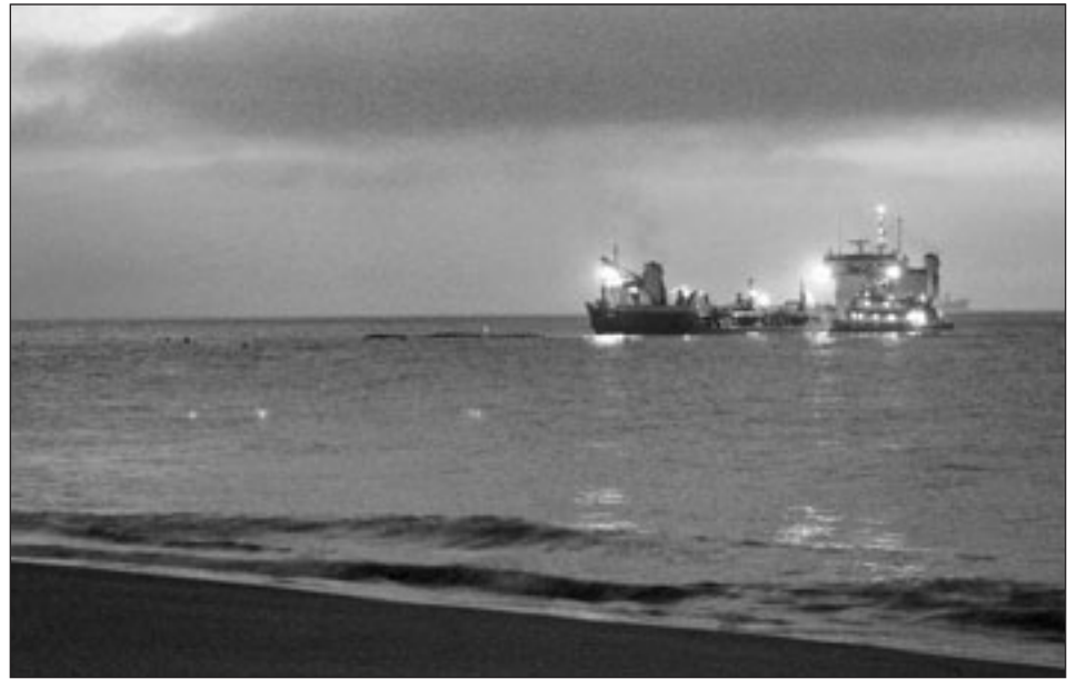
Dredging and pumping operations for beach nourishment contracts typically continued round the clock
