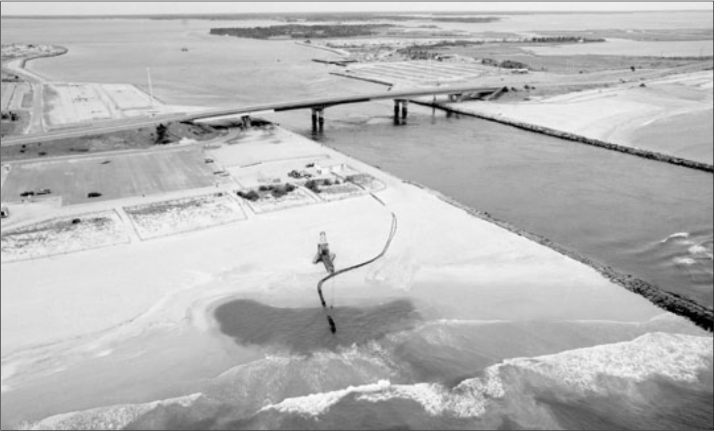
The sand bypassing plant at Indian River Inlet, Del., soon after construction in 1989
