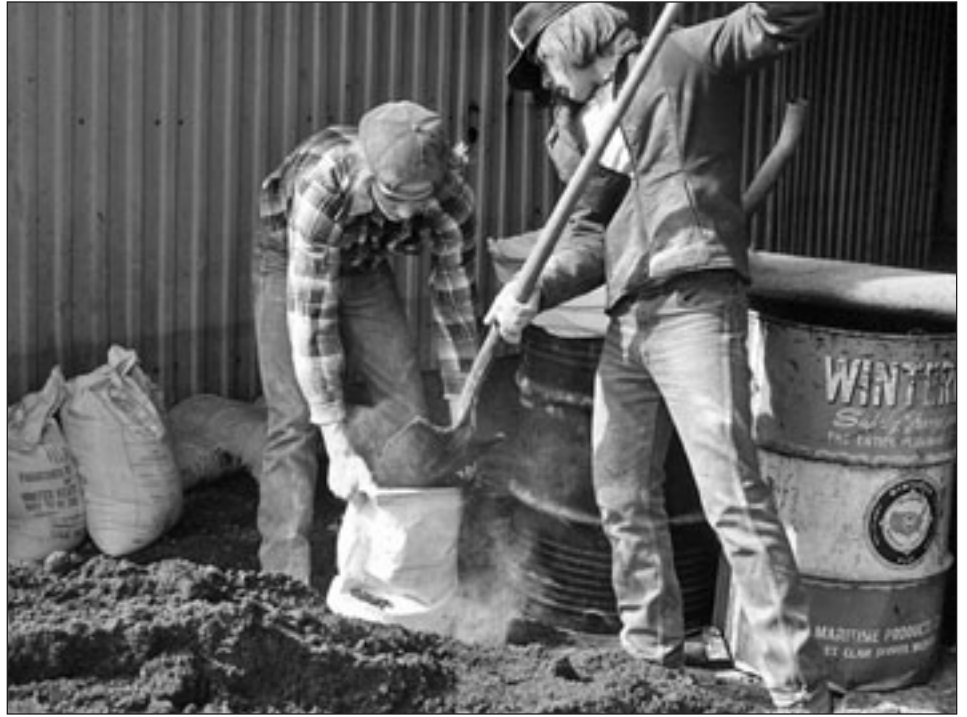
Filling sandbags for flood-fighting
