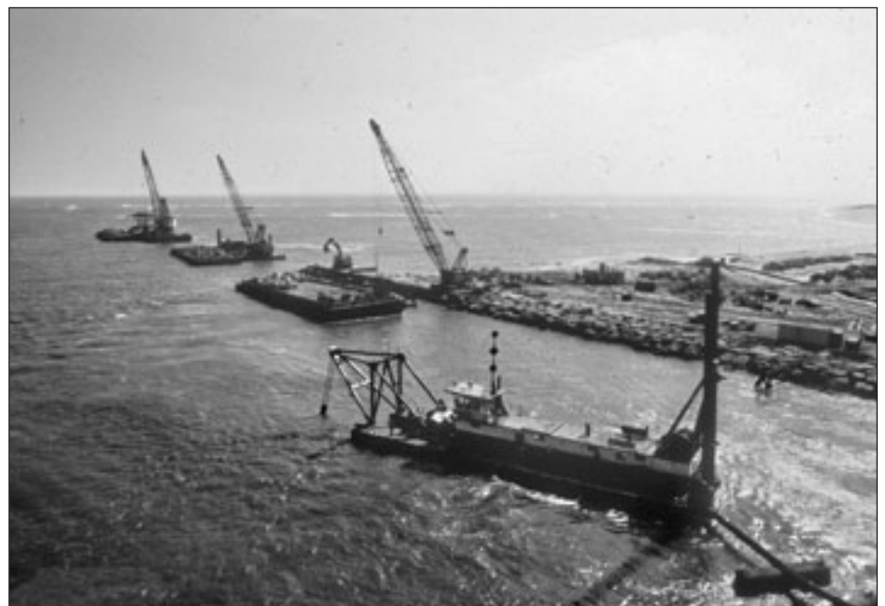
The plan for Barnegat Inlet involved construction of an entirely new south jetty backfilled with sand dredged from the inlet
