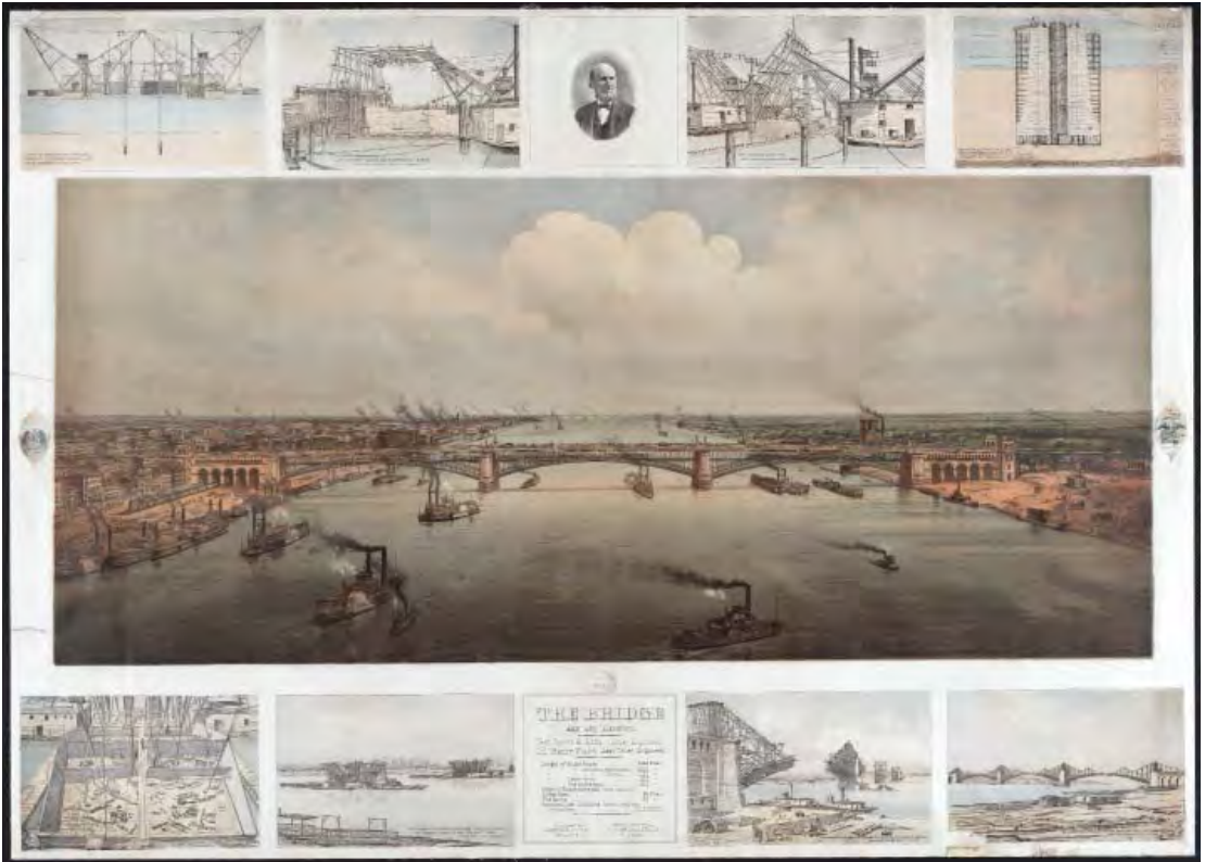
View of completed St. Louis Bridge with steamboats in Mississippi River and views of stages of bridge construction, based on photographs taken in 1874 by R. Benecke, sections of pier and machinery, and portrait of Capt. James B. Eads. 11437 U.S. Copyright Office, Copyright by Compton & Co. (1874) LOC
