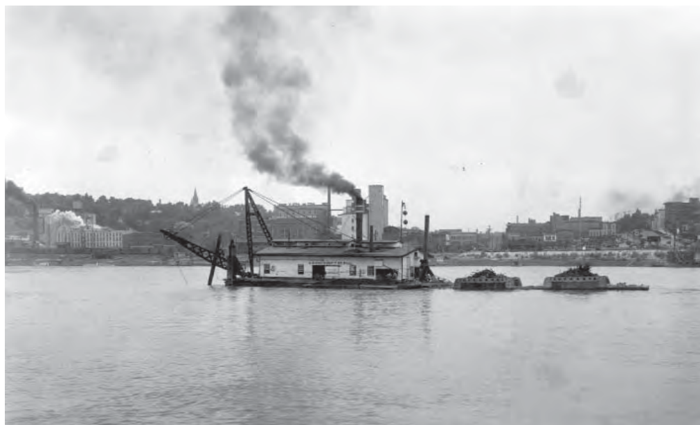
Dipper dredge St. Paul removing trailer dike near Lock and Dam No. 26
