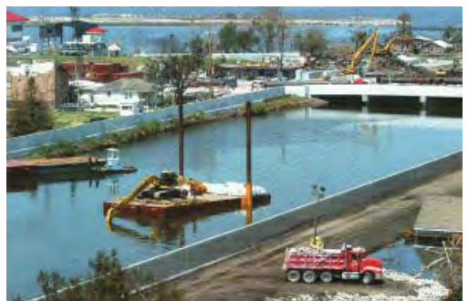
Flexiboat bridges used as waterbased platforms for closing of canal breaches
