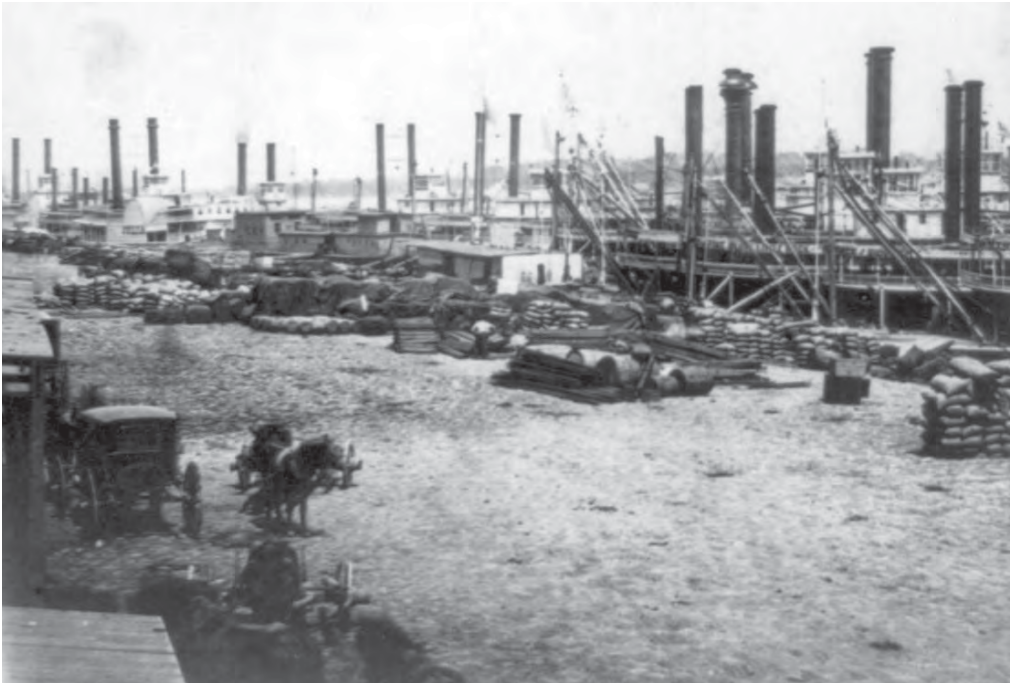
Levee, St. Louis, Missouri (LOC)
