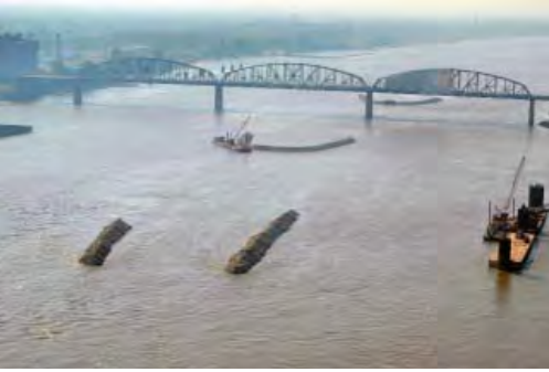
Construction of chevron dikes
