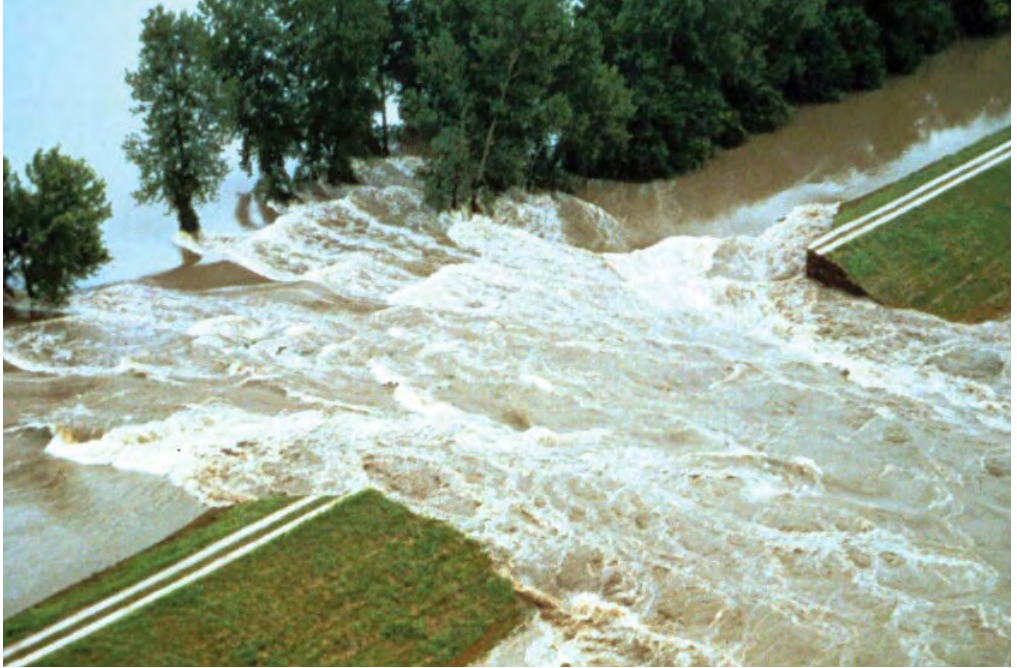
Levee overtopping during 1993 flood
