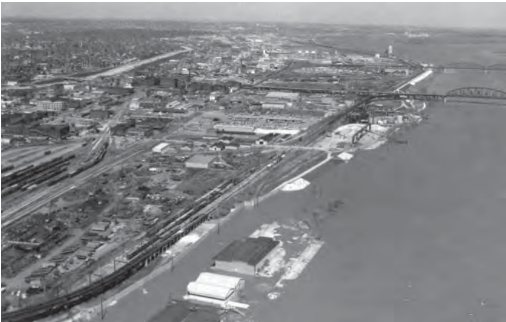
St. Louis floodwall that prevented flooding of large industrial areas during the 1973 flood
