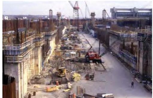
Second stage construction of main lock, November 1987
