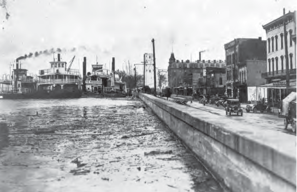
Cairo floodwall at the junction of the Ohio and Mississippi rivers during the 1927 flood
