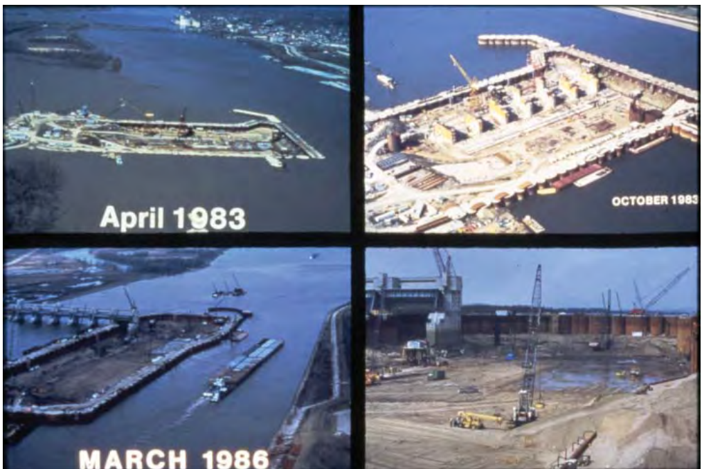
Construction stages at Lock and Dam 26R
