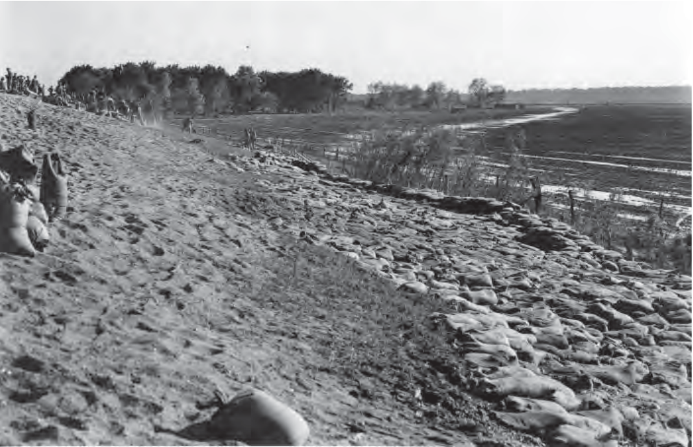
Flood fighting at Illinois River levee, 1943
