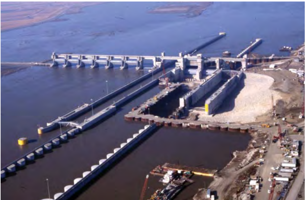
Third stage construction of auxiliary lock
