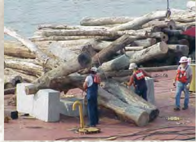
Logs being bundled for use as woody structures
