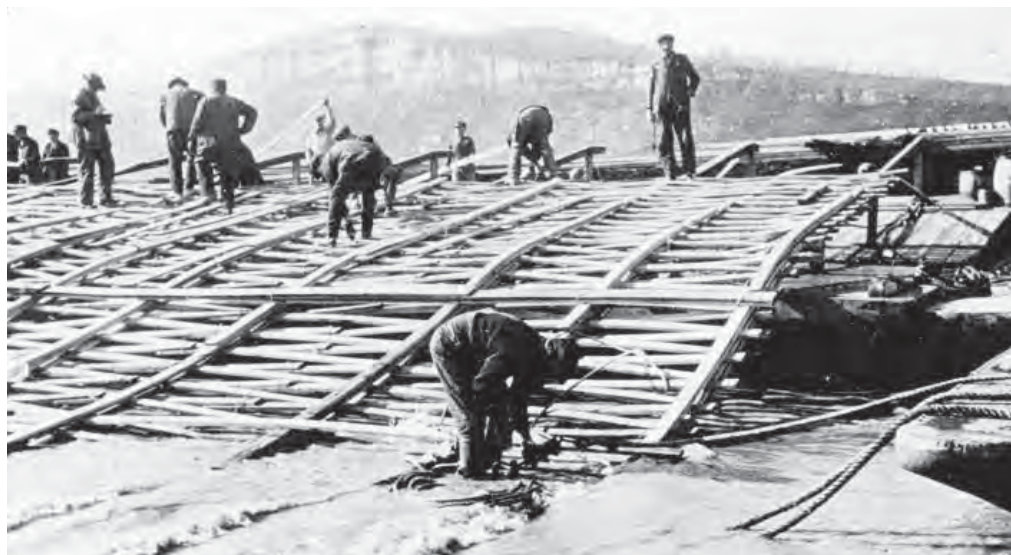
Construction of early mattress revetment
