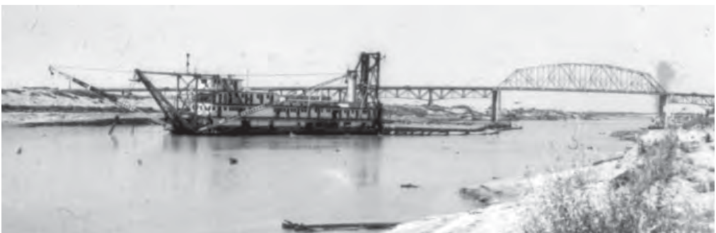
Dredge operations north of St. Louis, 1935
