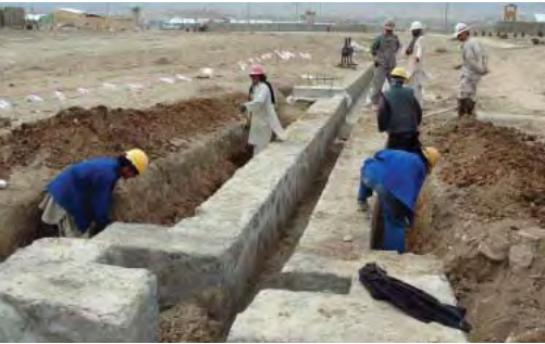
Corps personnel supervise Afghans constructing drainage trench
