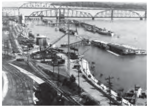
Lock and Dam 26 construction, 1938
