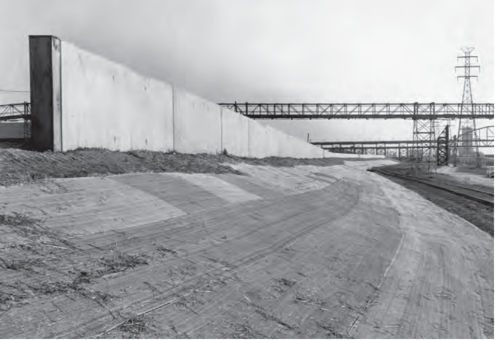
East St. Louis floodwall, 1951
