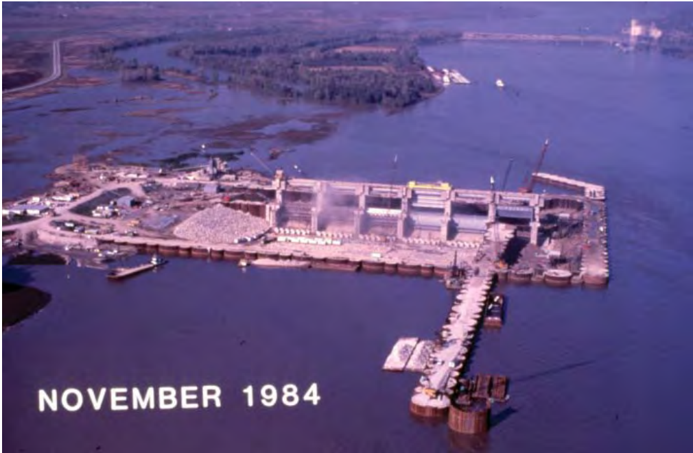
Stage one construction
