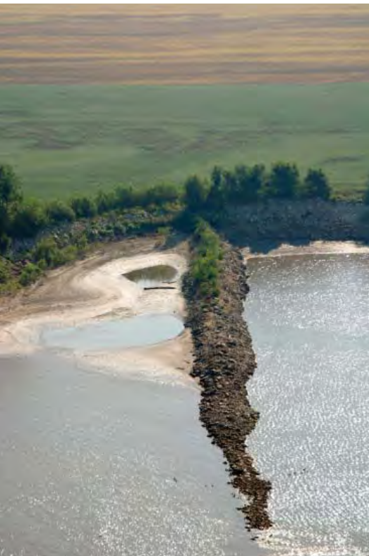
Dike using various sizes of rocks allowing for a greater diversity of habitats
