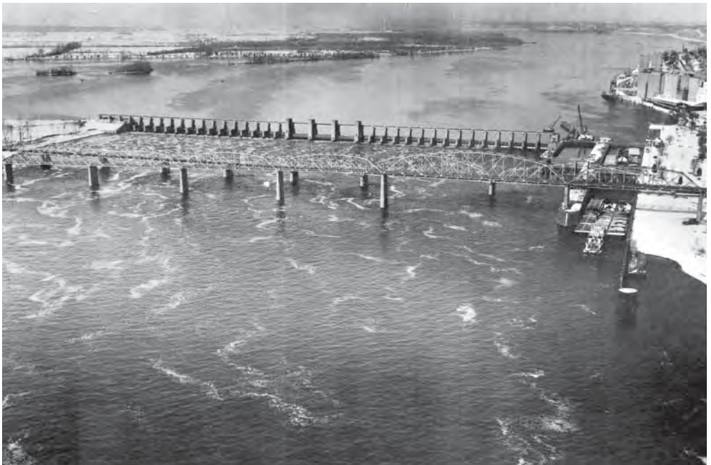
Aerial of old Lock and Dam 26
