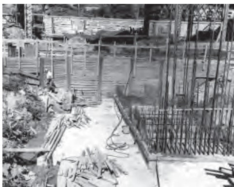
St. Louis Project floodwall, 1964
