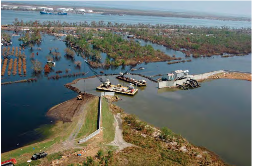
Repair of levee breach in New Orleans after Hurricane Katrina
