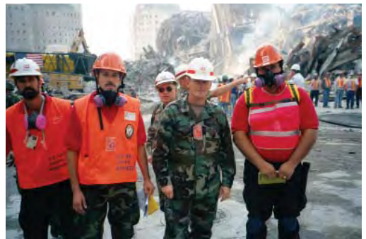
Corps personnel with Chief of Engineers Lt. Gen. Robert Flowers at World Trade Center
