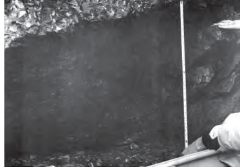
Closeup of crack in lock wall
