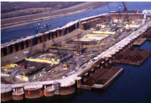
Second stage construction
