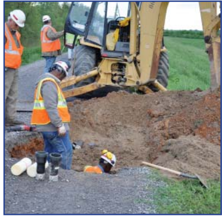
Memphis Engineer District work crews unearth the access wells at the Birds Point-New Madrid floodway fuseplug levee.
