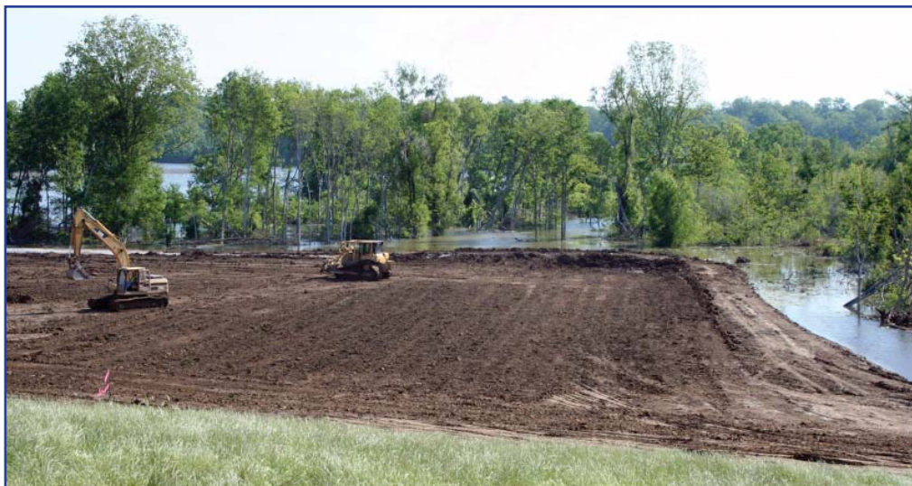
The clay cap nears completion at Buck Chute as water from Eagle Lake continues to rise.
