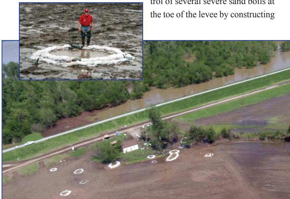
Sand boil rings near the toe of the levee surround a home in Fulton County.
