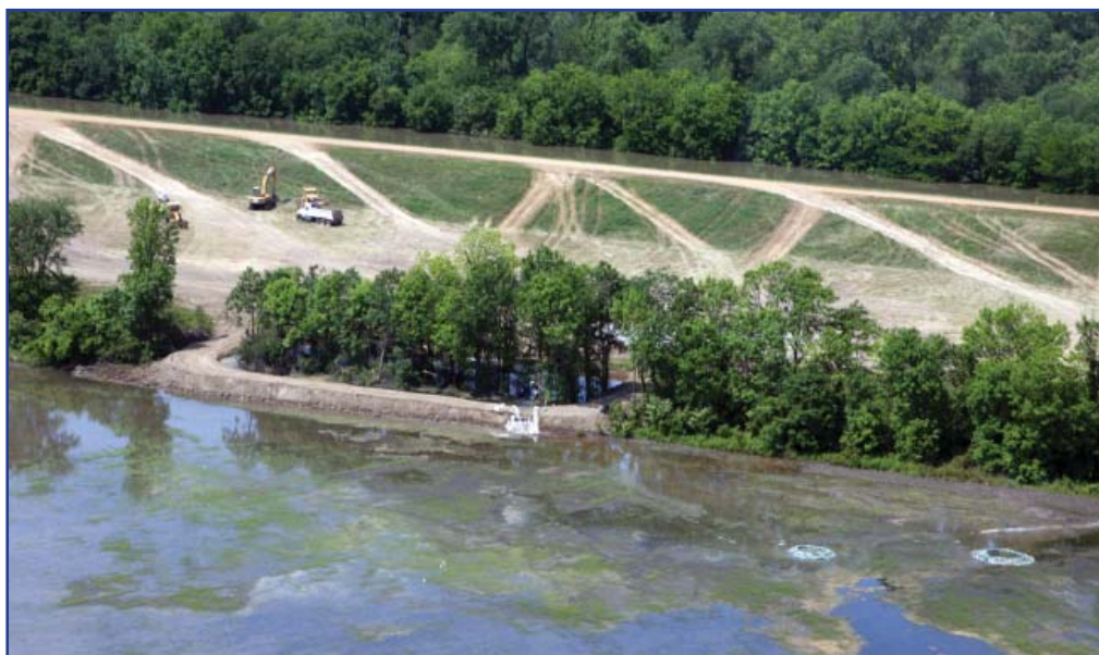
The completed water berm at Francis, Miss. Note the additional sand boil rings in the foreground and the river stage in the background.
