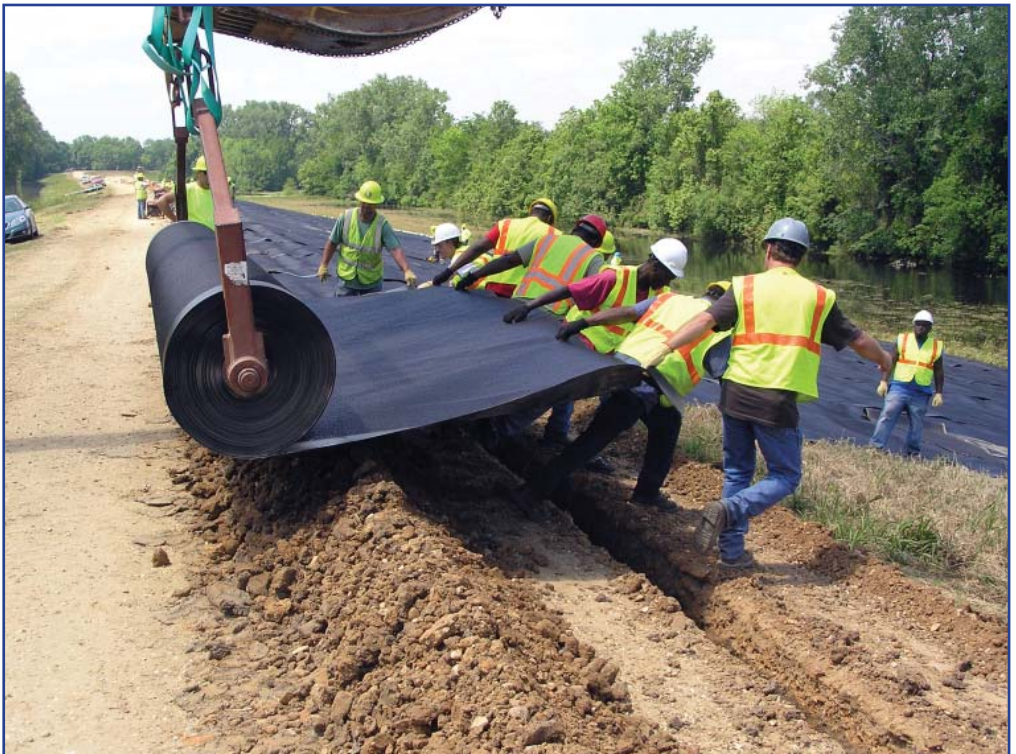
Armoring the Yazoo backwater levee.
