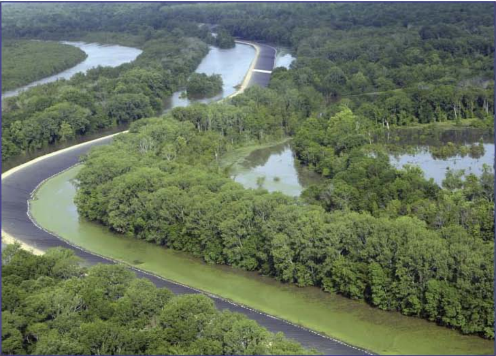
The river encroaches upon the gravel road at the crown of the armored Yazoo backwater levee. Note the trapped interior drainage to the right of the levee.
