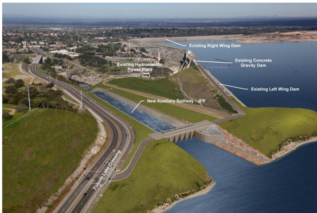
Figure 1-1. Existing Folsom Dam with a Rendering of the New JFP Auxiliary Spillway.
