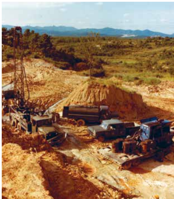
Drilling operation at Tunnel #3, June 1978.
