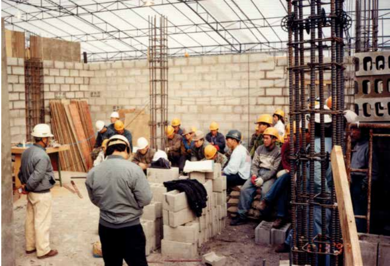
Standard-design barracks under construction at Camp Stanley, 1996.
