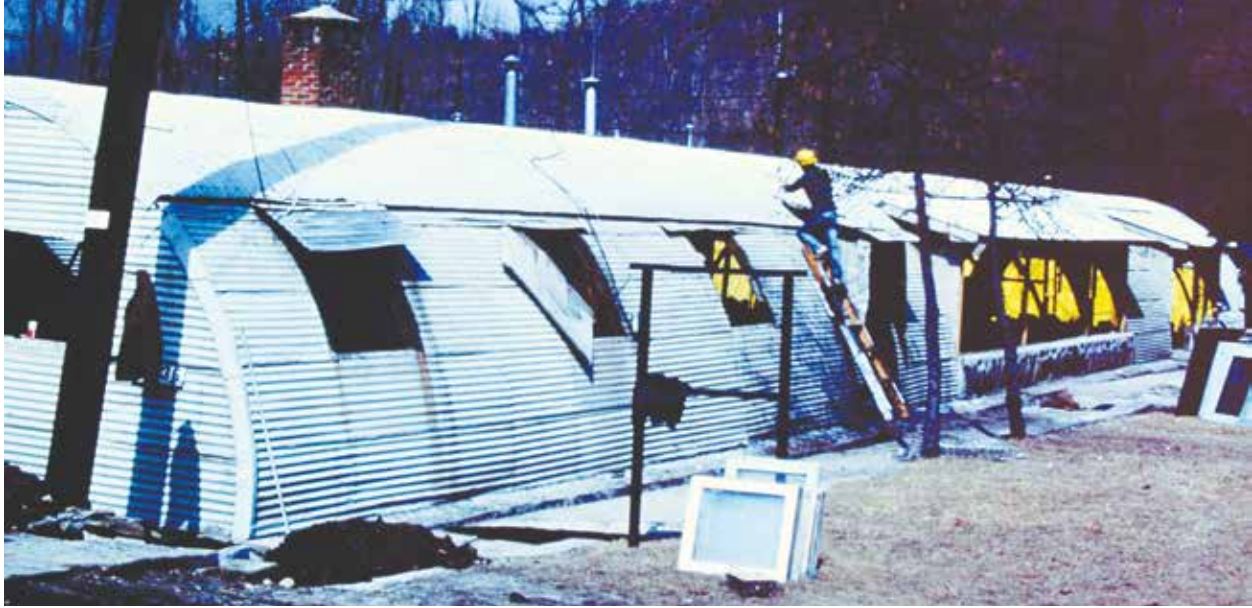
Rehabilitating Quonset huts in the Forward Area, circa 1979.
