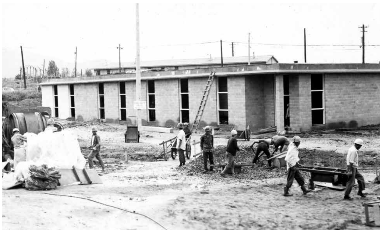
Construction of a new 500-man mess hall at Camp Red Cloud, September 1969.
