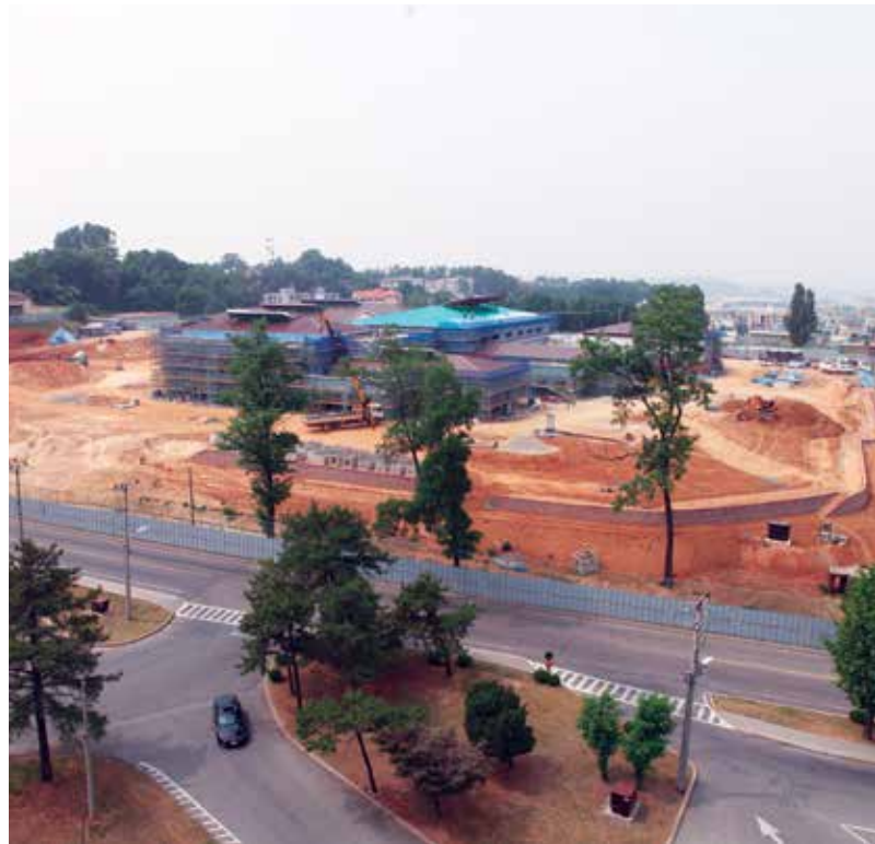
A new school under construction at Osan Air Base, 2015.
