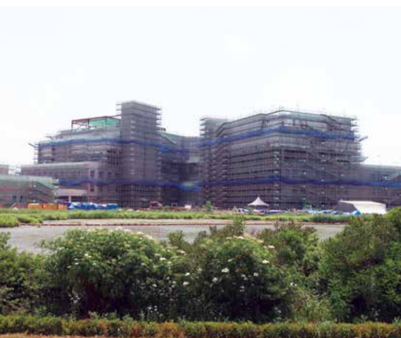
A new, state-of-the-art hospital under construction at USAG Humphreys, 2015.
