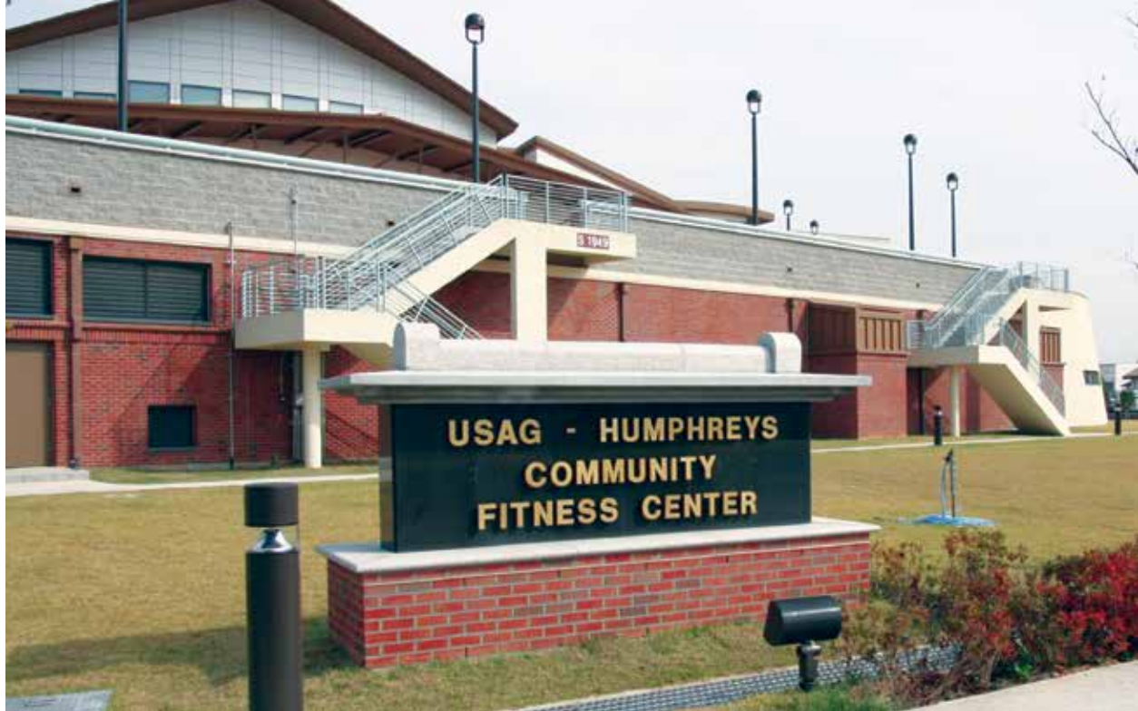
Exterior view of the Humphreys Community Fitness Center, 2008.
