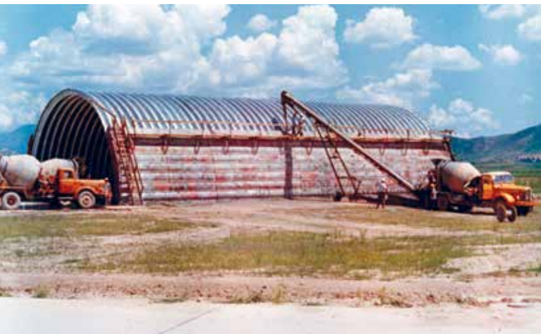
Placement of concrete cover on aircraft shelter, Kwangju Air Base, August 1969.
