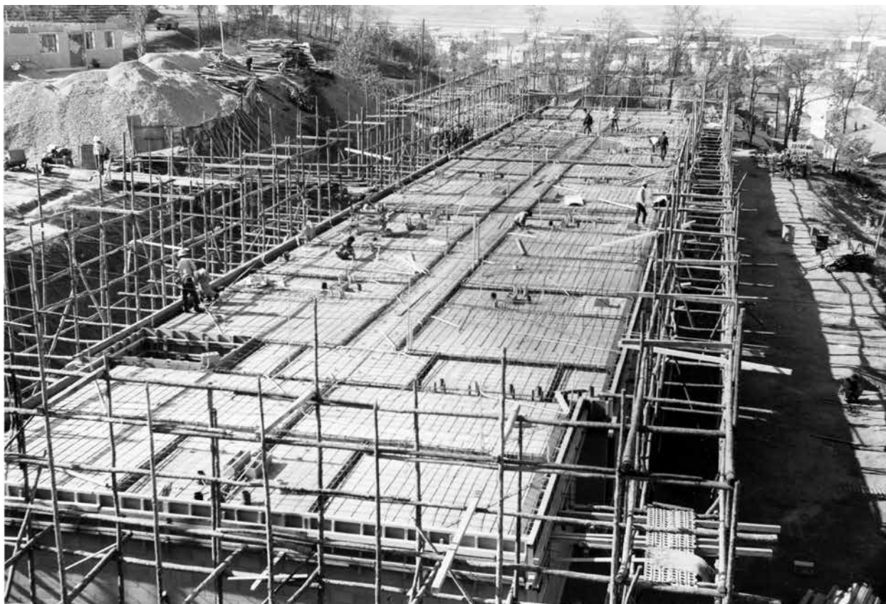
Officers quarters at Osan Air Base, November 1967.
