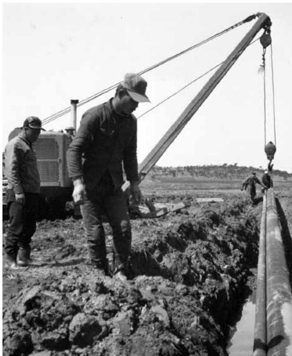
Pipeline casing being lowered into a trench, April 1969. Credit: NARA RG 111, CC-56300
