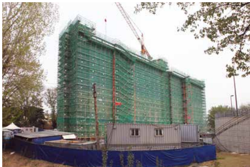
Barracks construction at Camp Carroll, 2015.
