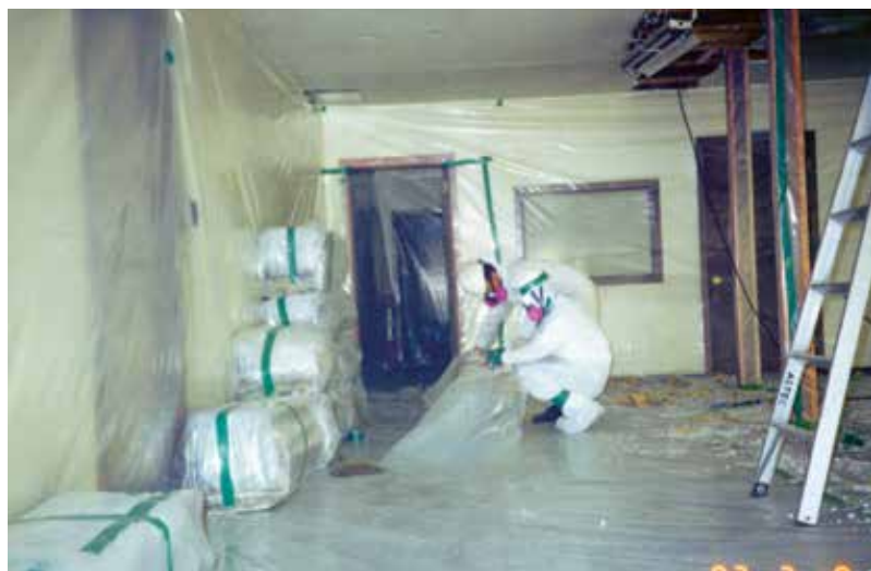
Asbestos abatement work in the 1990s.
