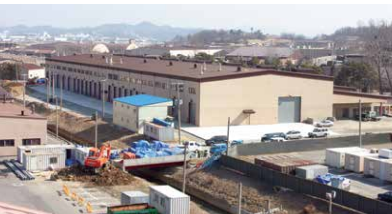
A maintenance and operations facility completed at Osan Air Base, 2005.
