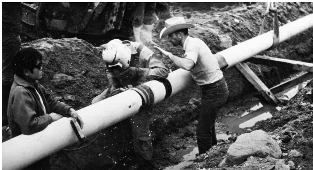
Welding together segments of the trans-Korea pipeline, circa 1969.
