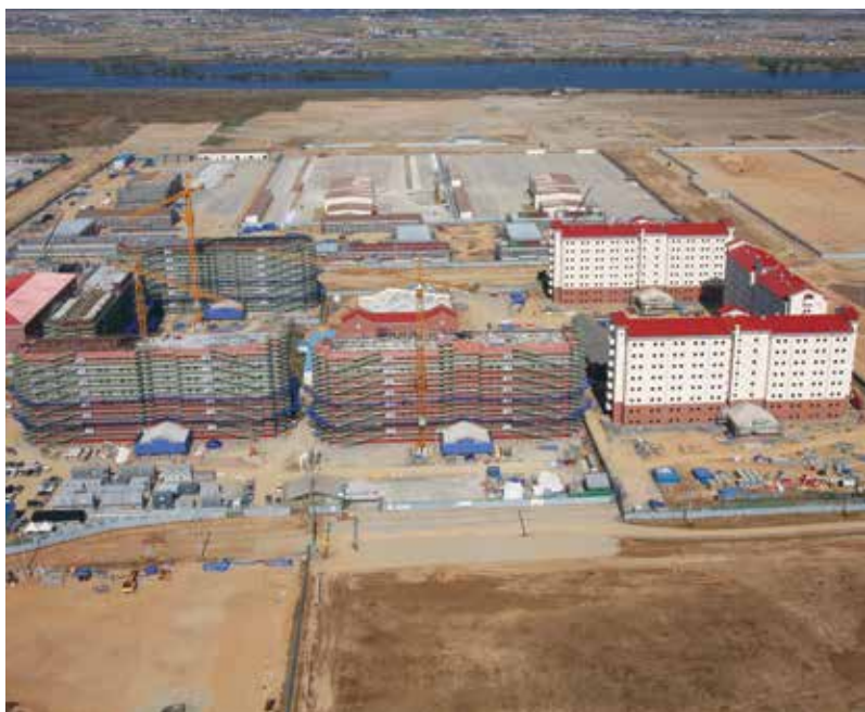
Barracks construction in full force at USAG Humphreys, 2013.
