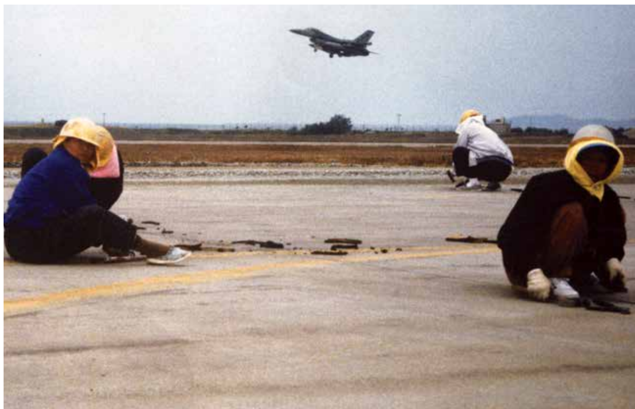
Runway repairs at Kunsan Air Base, 1990.
