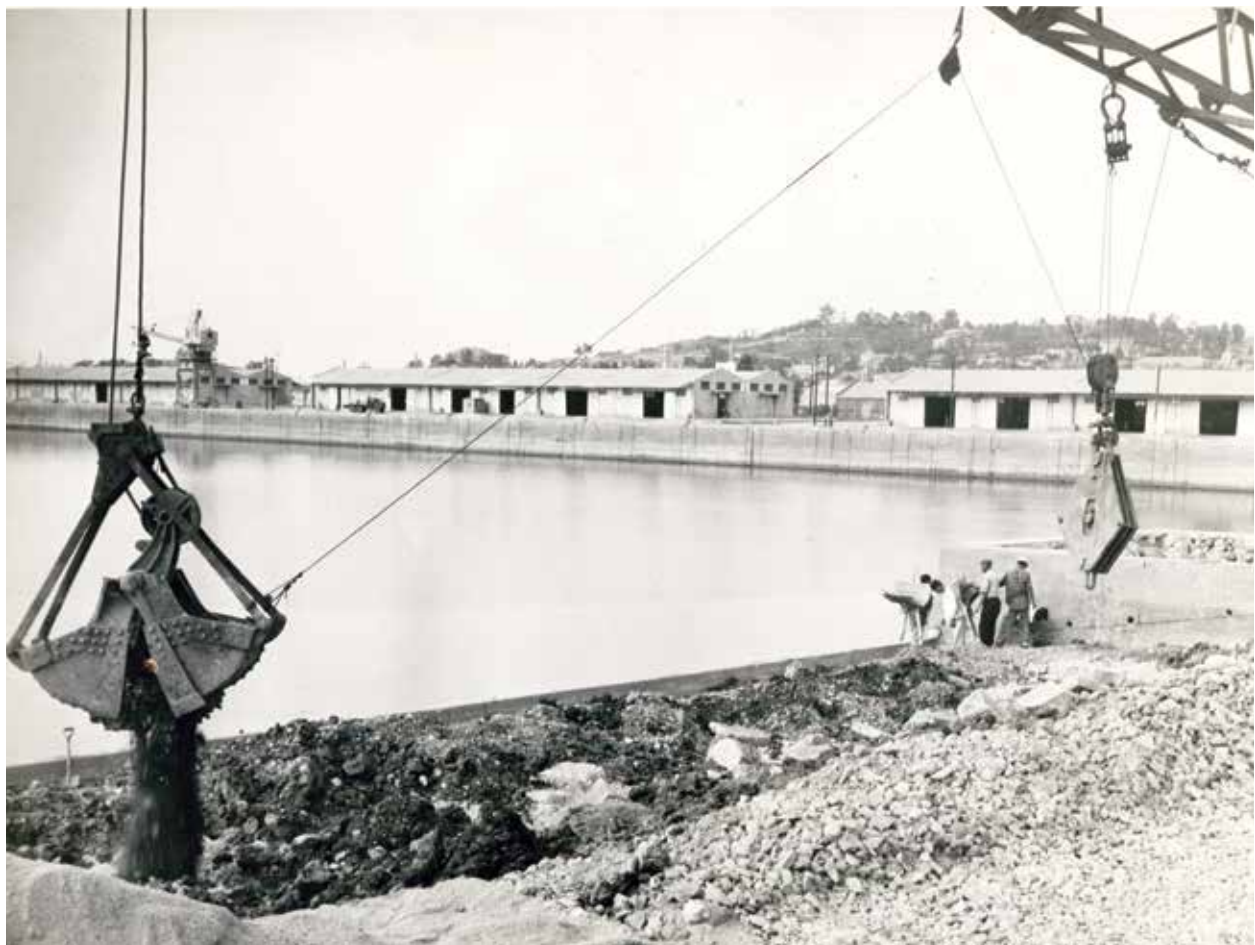
Placement of fill material at Incheon Tidal Basin, 1960. Credit: Photo by PFC D. Heyde, FED, FED-PAO Historical Files.
