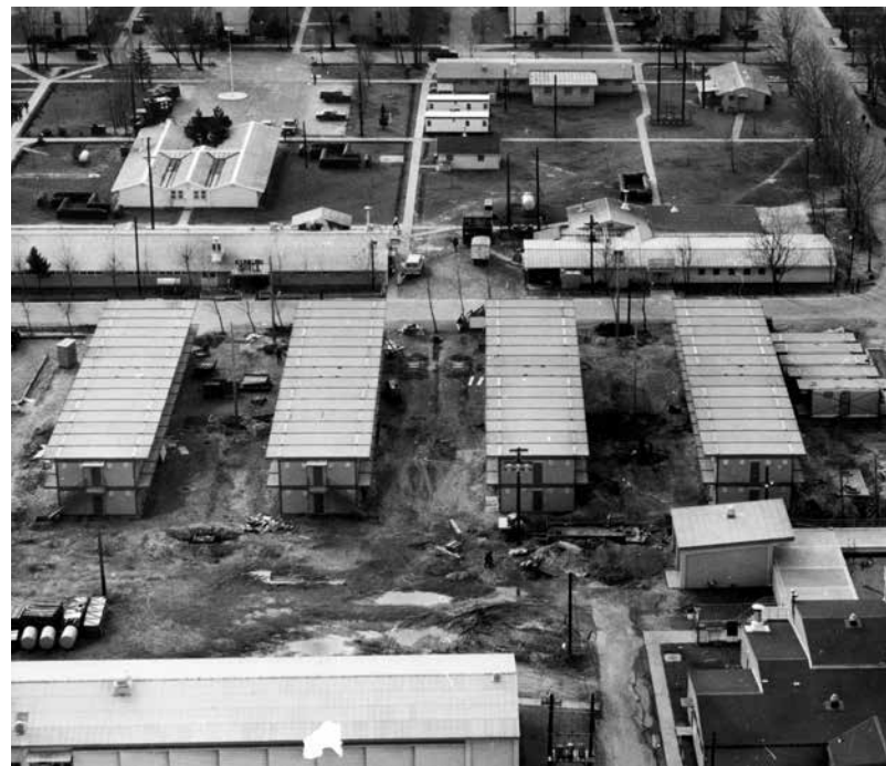
Modular dormitories at Kunsan Air Base, December 1968.
