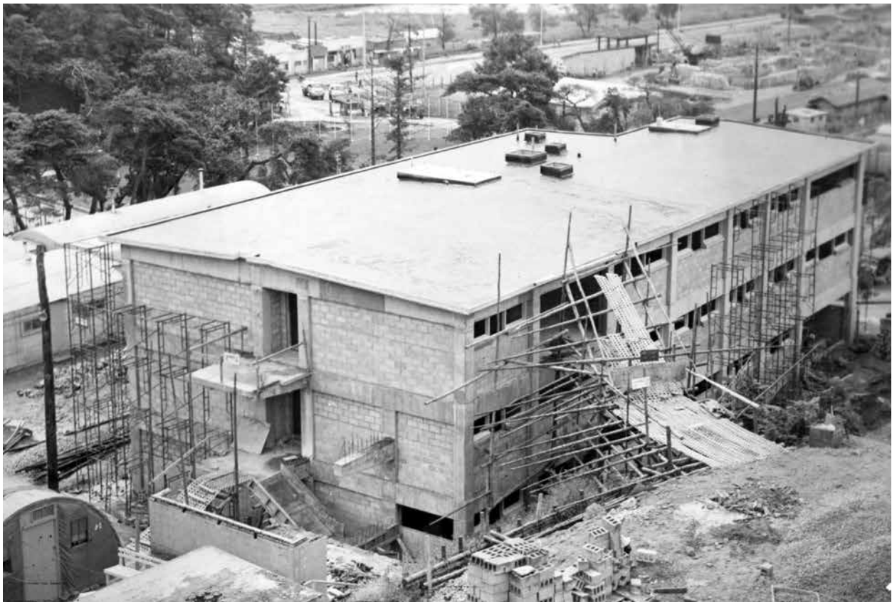
Barracks nearing completion at Camp Howze, September 1969.
