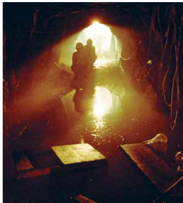
Workers in an intercept tunnel.
