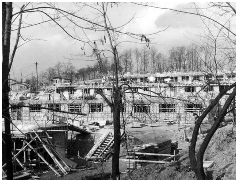
Construction of troop housing at Yongsan Army Base, 1975.
