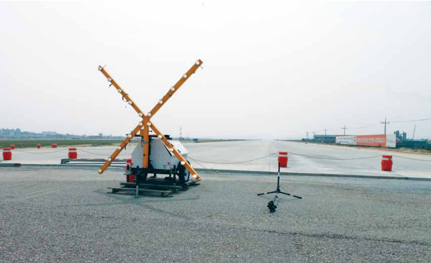
A recently completed runway at Osan Air Base, 2015.
