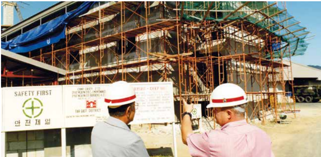
USACE personnel discuss progress of barracks construction at Camp Casey, 1988.
