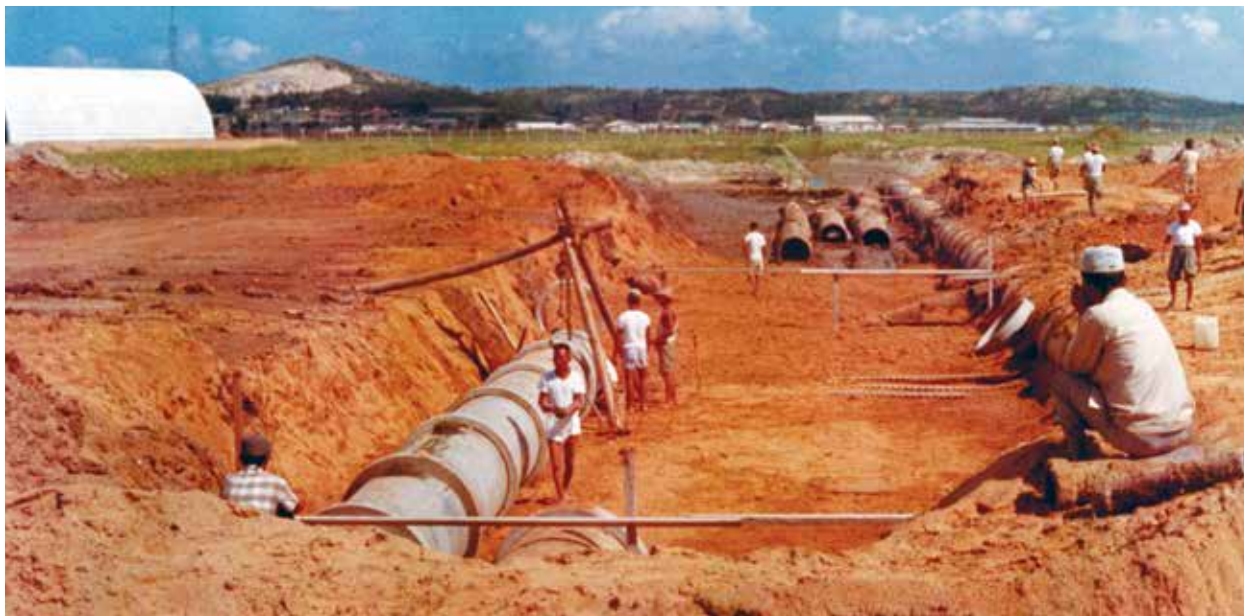
Laying concrete pipe for cross-wind runway at Kunsan Air Base, August 1969.
