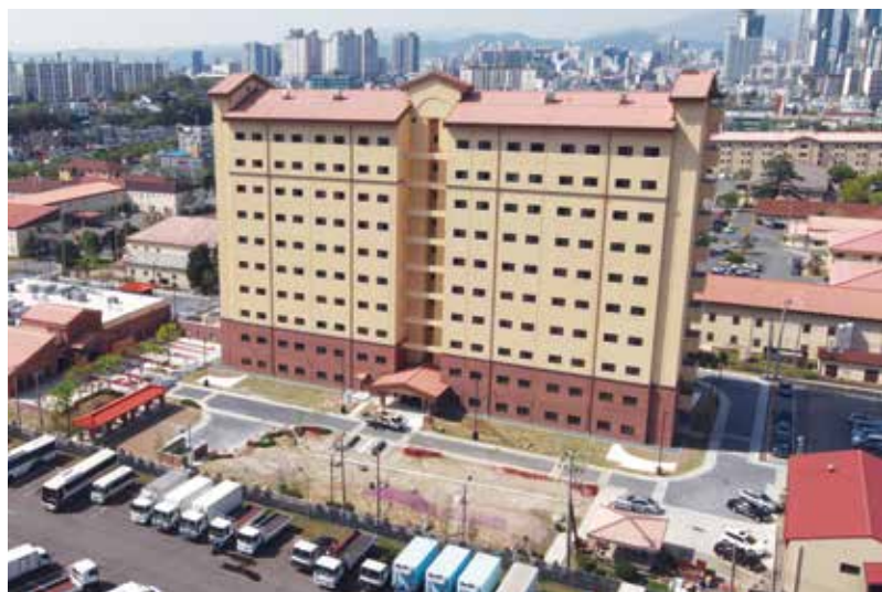
Barracks nearing completion for the U.S. Army at Daegu, 2015.
