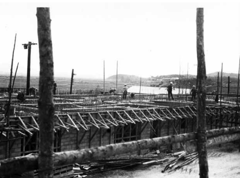
Construction of troop housing at Camp Humphreys, 1975.
