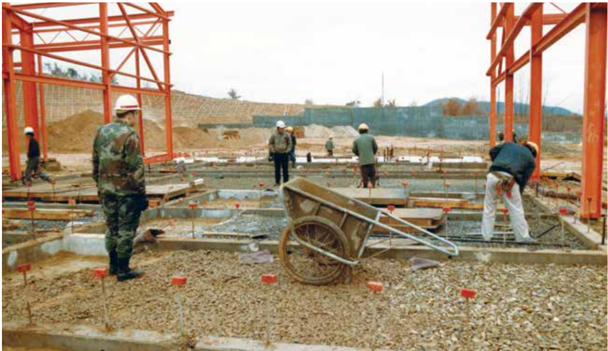
Workers at a Camp Carroll construction site.
