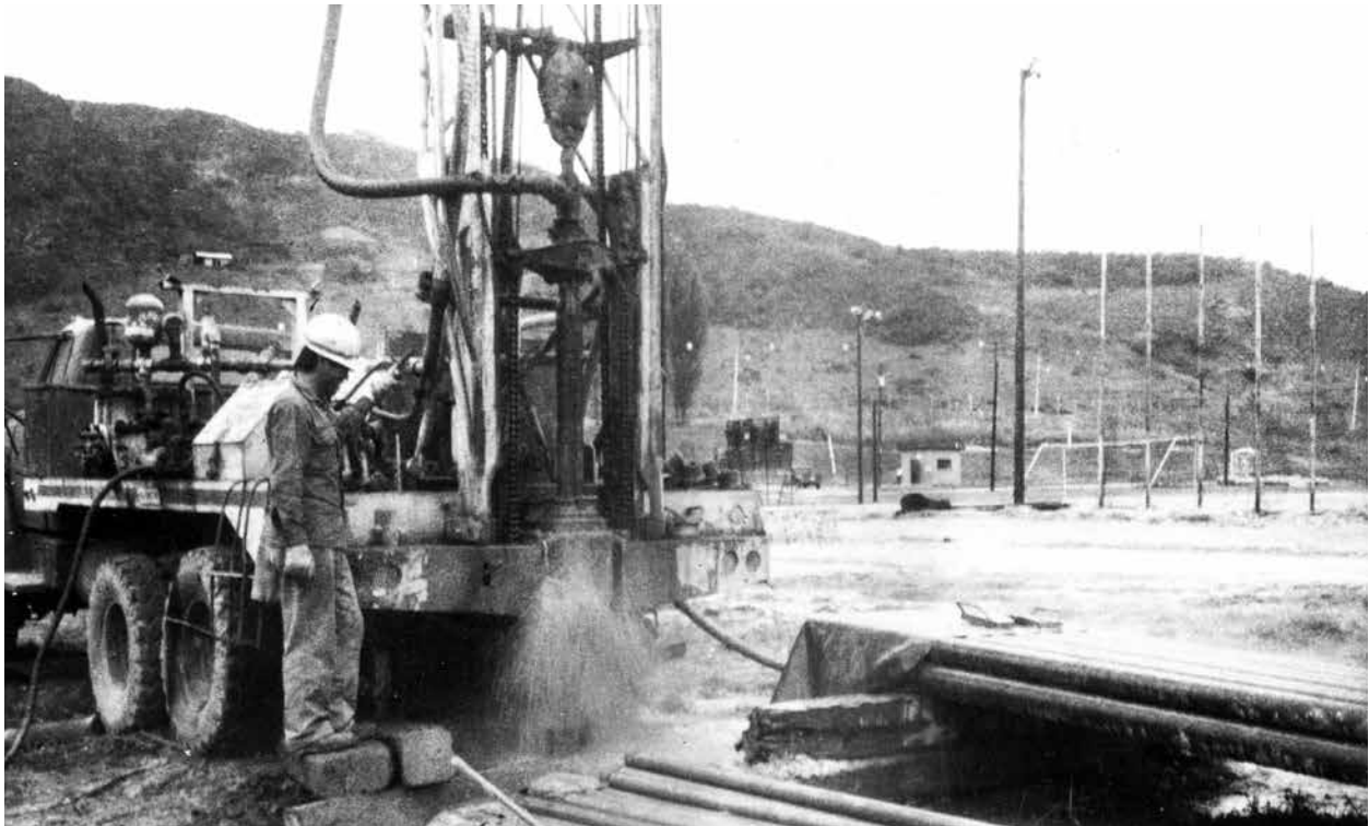
A worker drills a water well at Camp Hovey.
