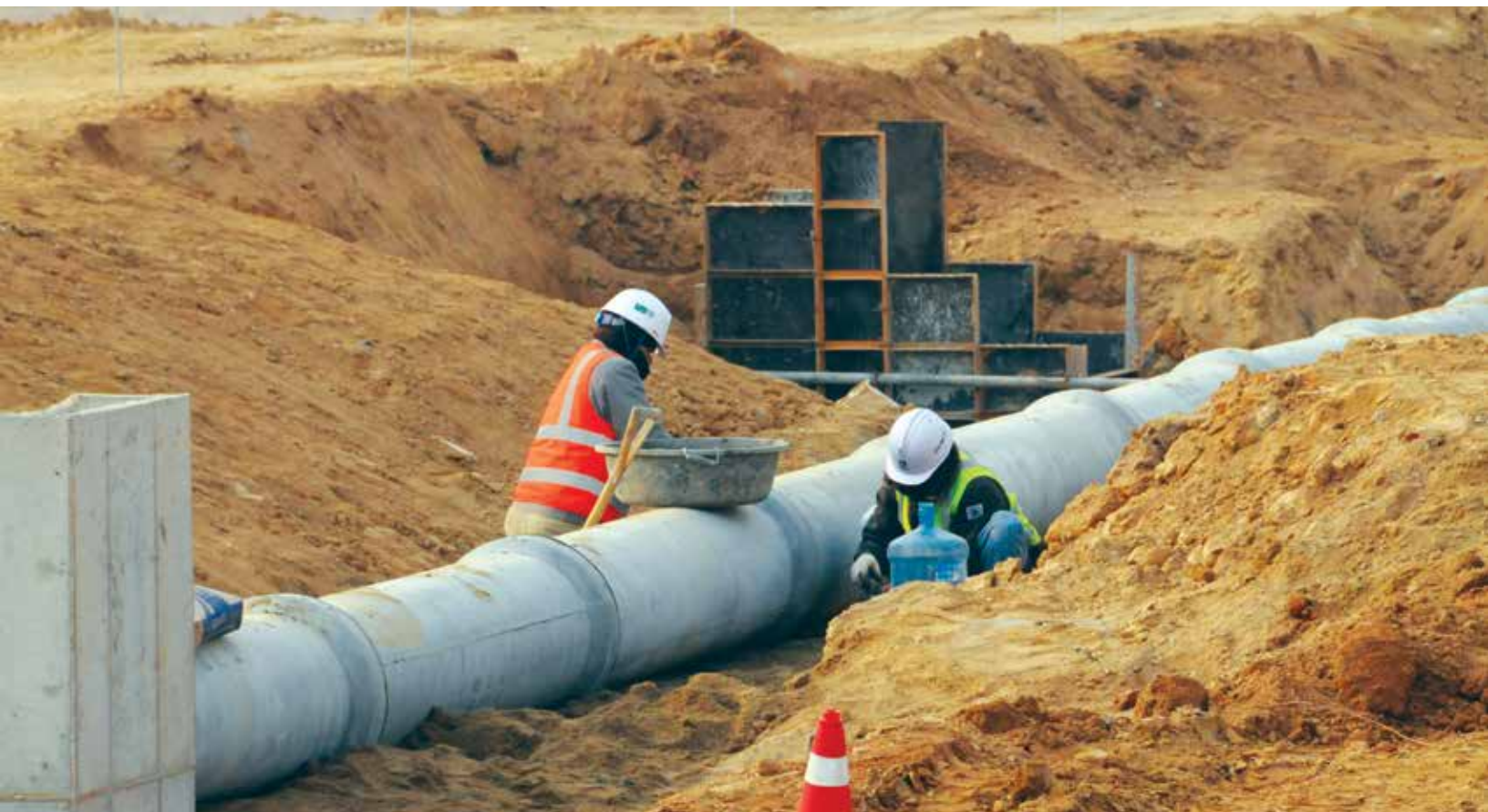
Contractors work on utility pipes at U.S. Army Garrison Humphreys, 2012.
