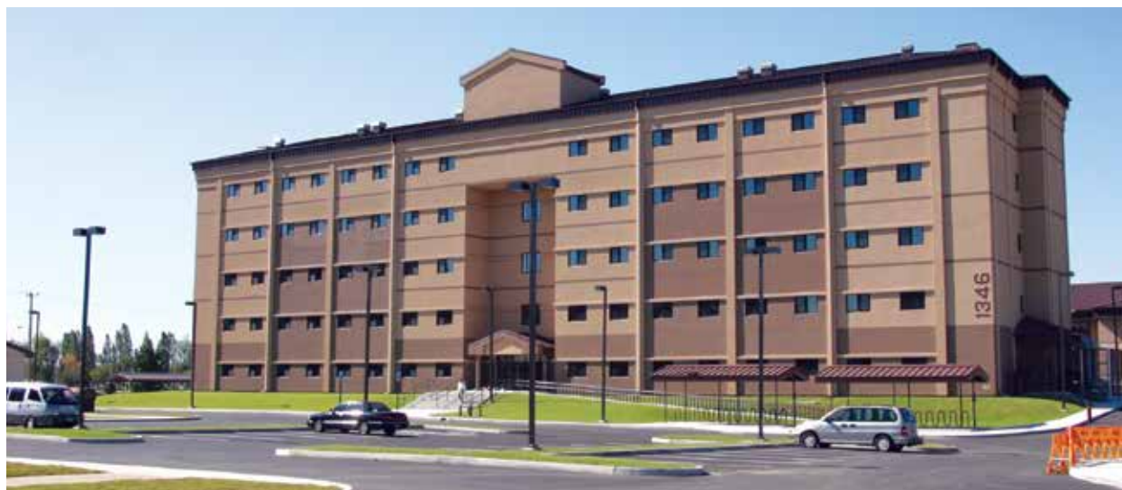
A new dormitory at Osan Air Base, 2006.
