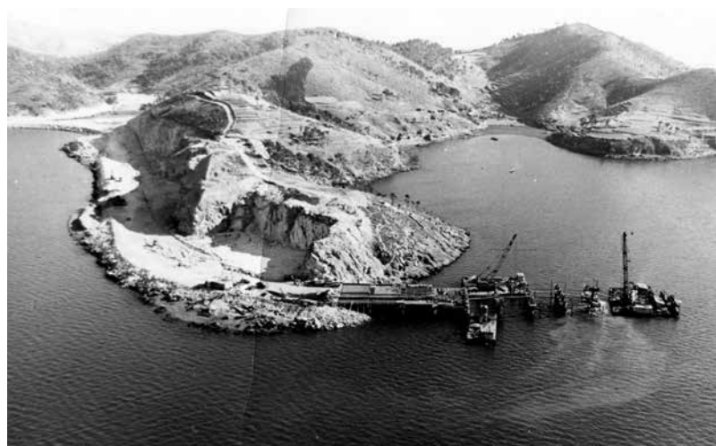
Construction of the pier at Chinhae ammunition port, 1970.
