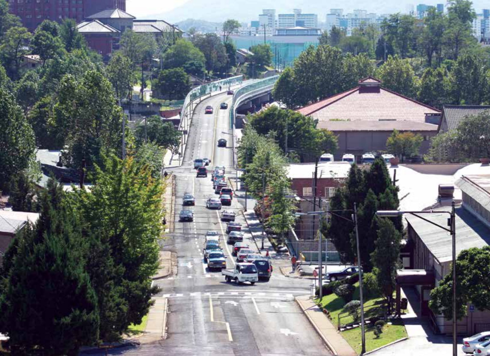
The Yongsan overpass allowed USFK to cross the base with ease, negating the numerous checkpoints used before the overpass was installed.
