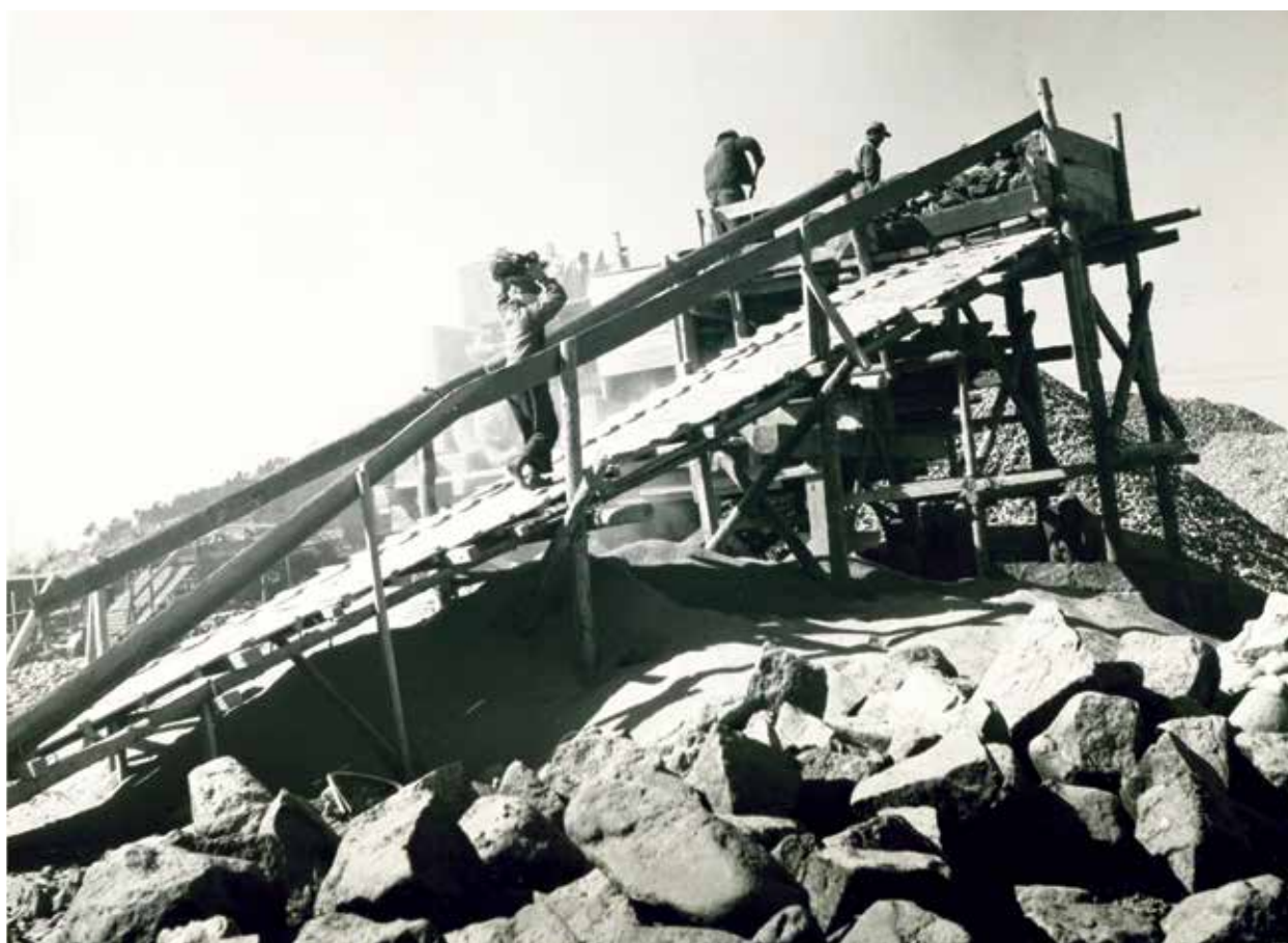
Korean workers transporting rocks by hand to a crusher at Incheon Tidal Basin, circa 1959, typical of the manual labor methods of the day. Credit: Photo by Sergeant Ray Boswell, FED, PAO-FED Historical Files
