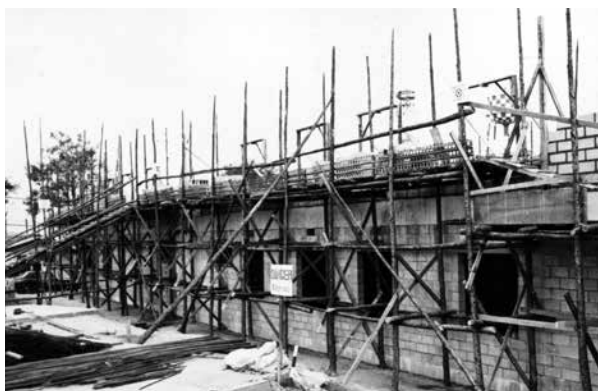
Camp Humphreys communication facility under construction, 1975.
