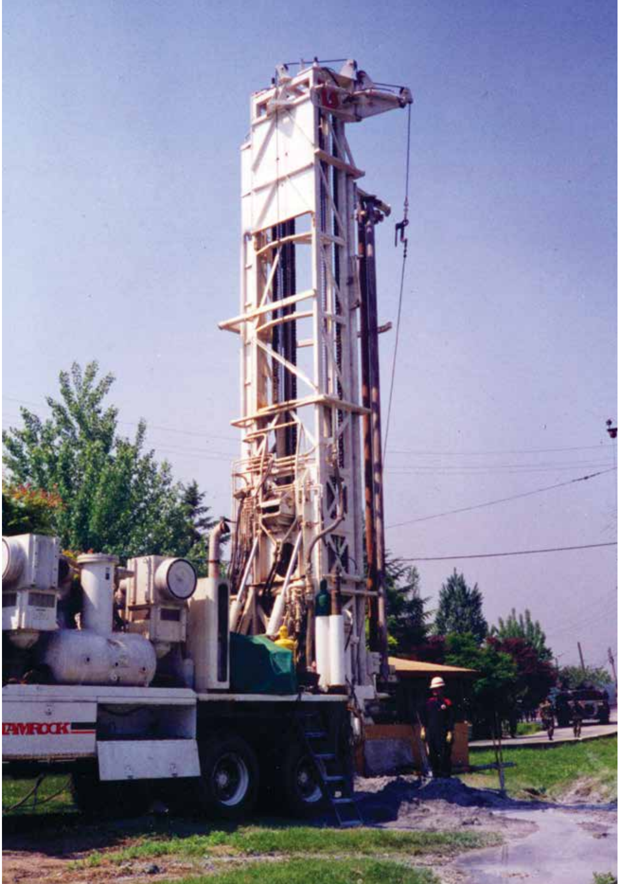
A Far East District well-drilling rig in operation, 1999.
