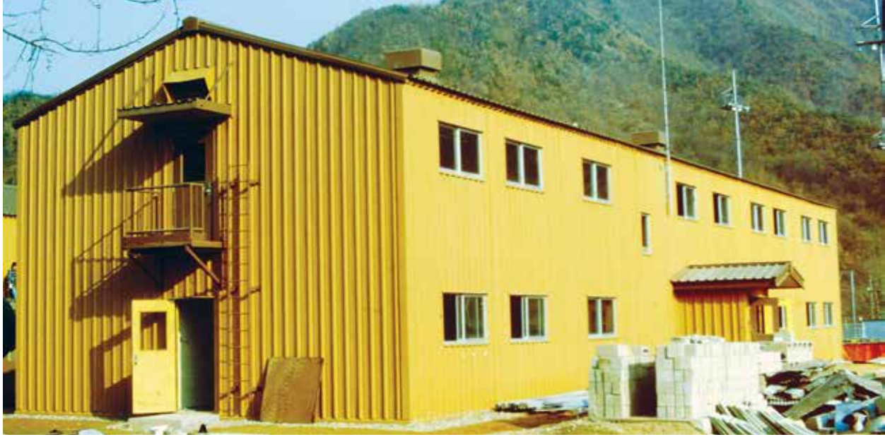
Two-story relocatable housing unit, circa 1979.
