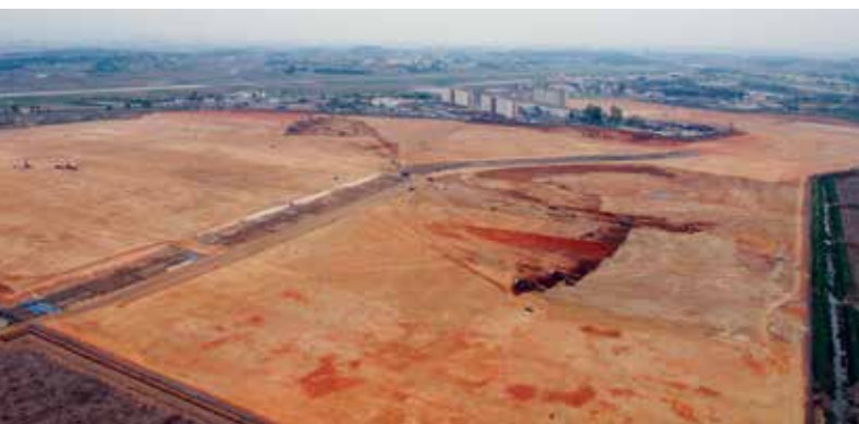
Land being prepared for new construction at Camp Humphreys in 2008.
