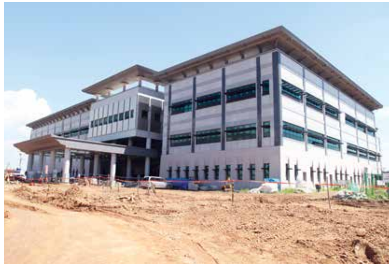
Eighth Army headquarters building under construction at USAG Humphreys, 27 August 2015.
