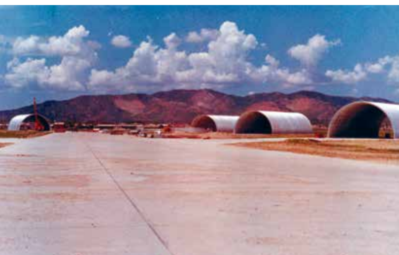
Kwangju pavement improvements and corrugated sheet-metal for aircraft shelters, 1969.
