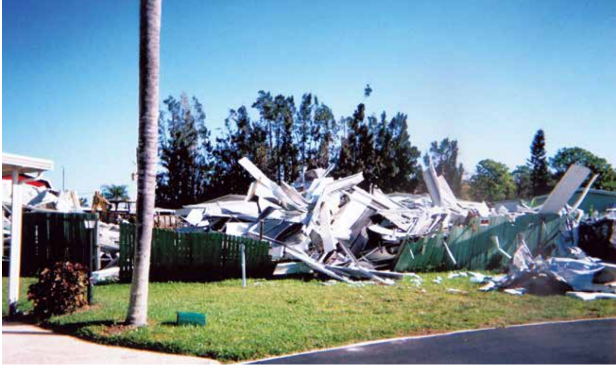
Destruction from Hurricane Wilma, 2005.
