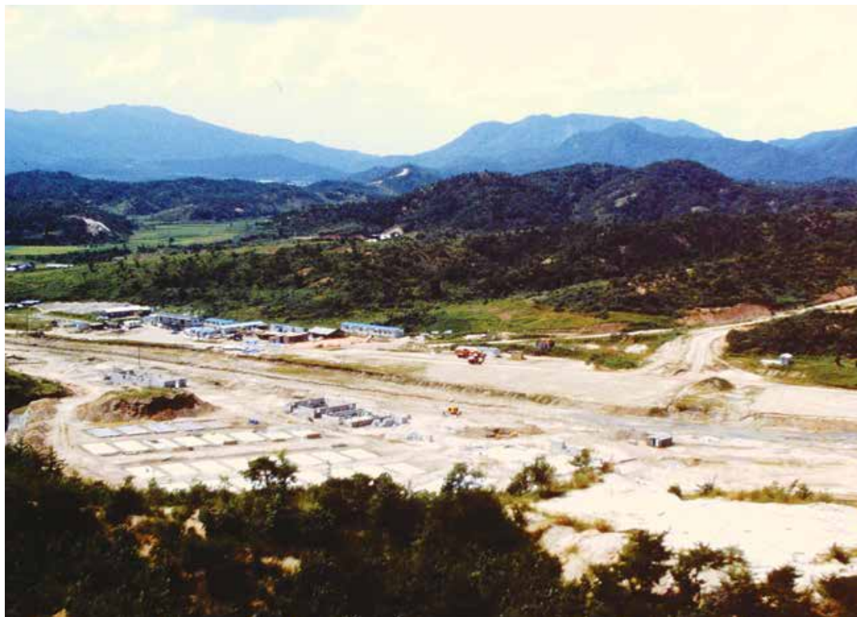
The Rodriguez Live Fire Complex under construction, 1986.
