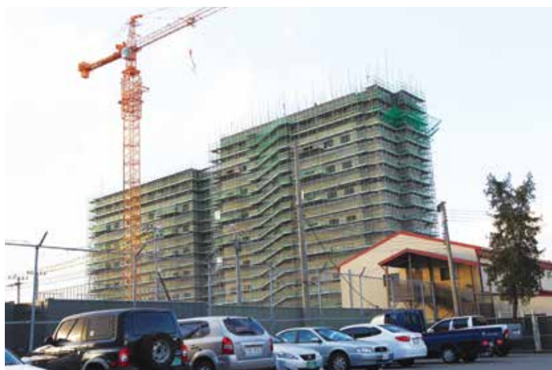
Barracks construction at Camp Henry, 2013.
