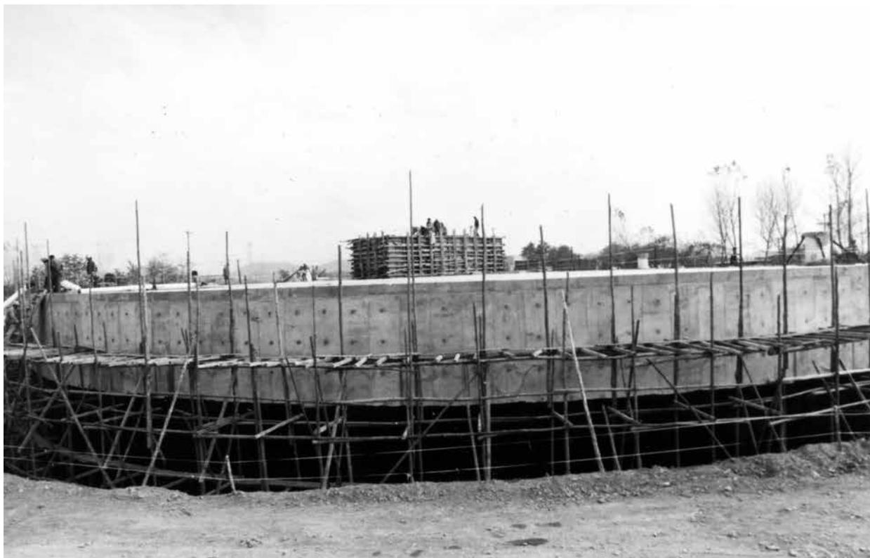
Construction of a 100,000-barrel jet fuel storage tank at Kwangju Air Base, 1983.
