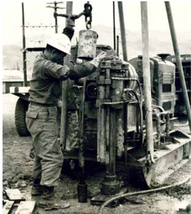
A FED employee takes a core sample for soil moisture at Hialeah Compound, near Pusan, February 1960. Credit: Photo by Sergeant Ray Boswell, FED, PAO-FED Historical Files
