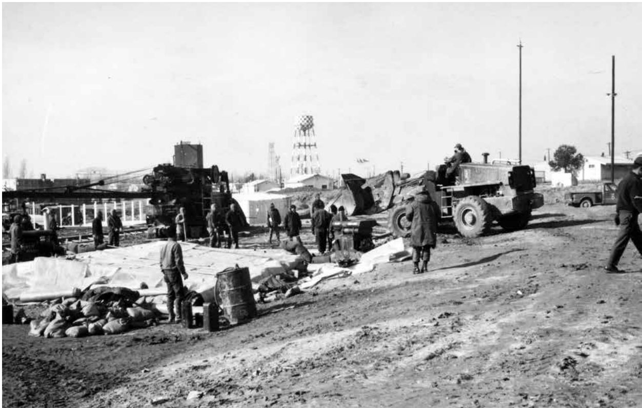
Construction workers at Camp Humphreys, circa 1972.
