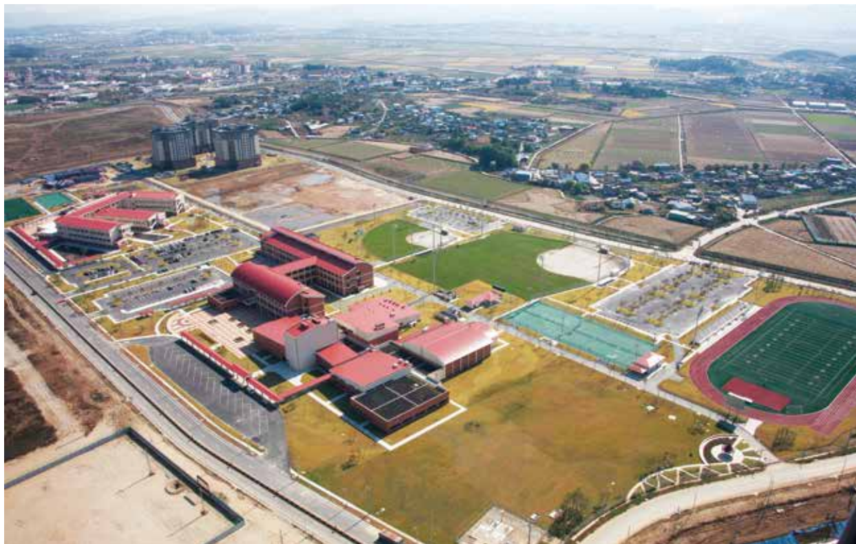
Aerial view of the school campus at USAG Humphreys, 2013.
