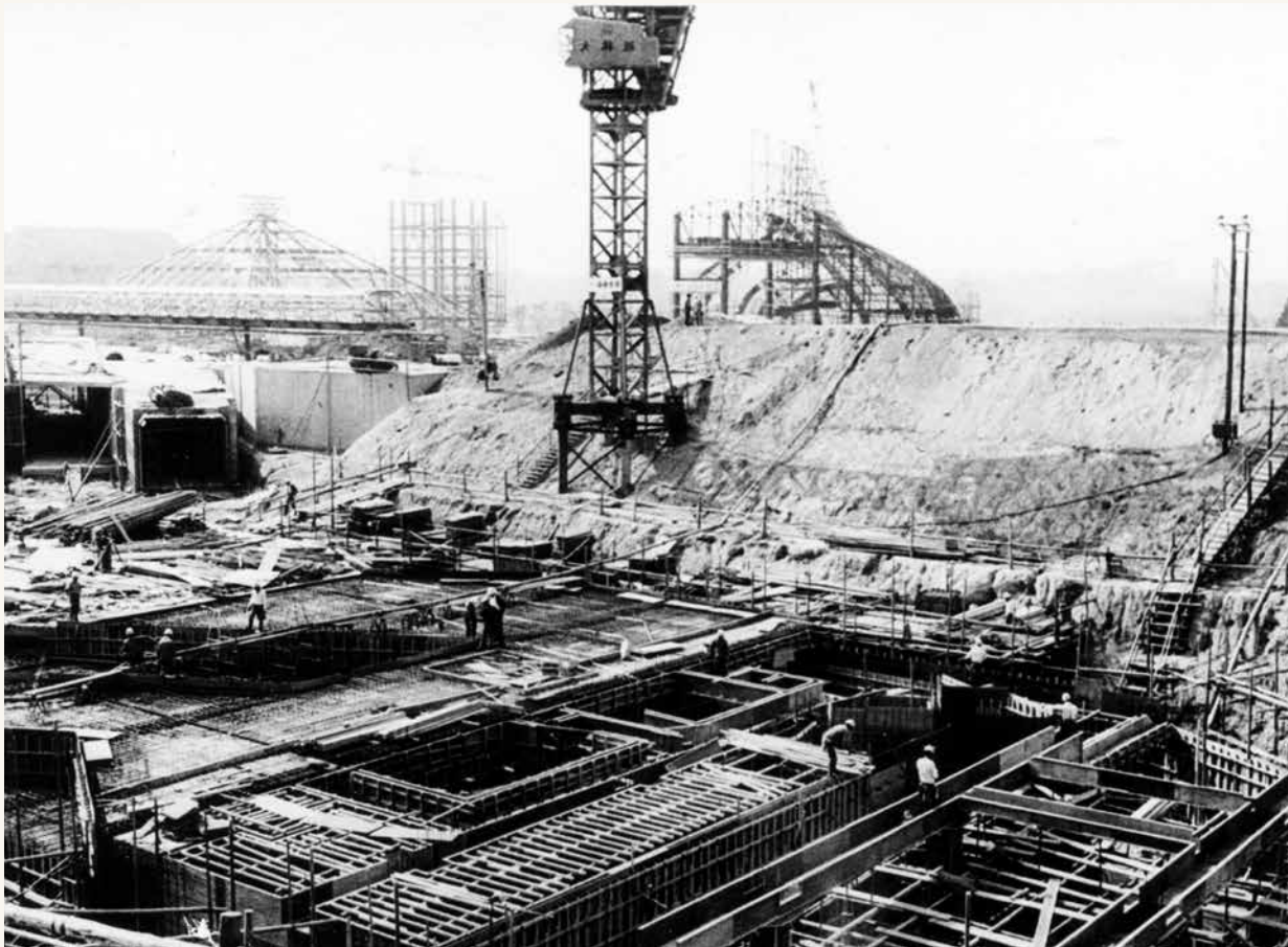
Construction at Expo '70 in Osaka, Japan, May 1969.
