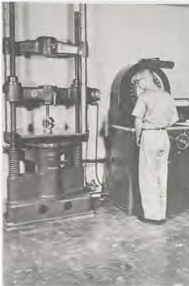
Marshall stability test in progress
