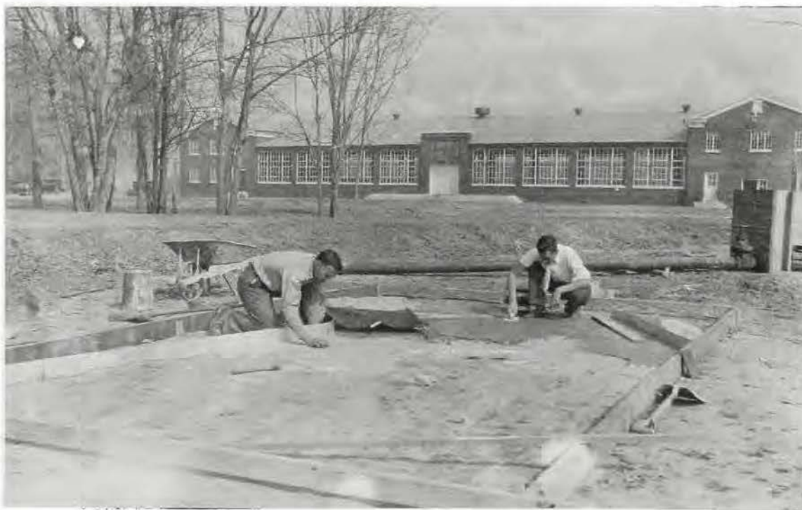
Construction of Bonnet Carré model
