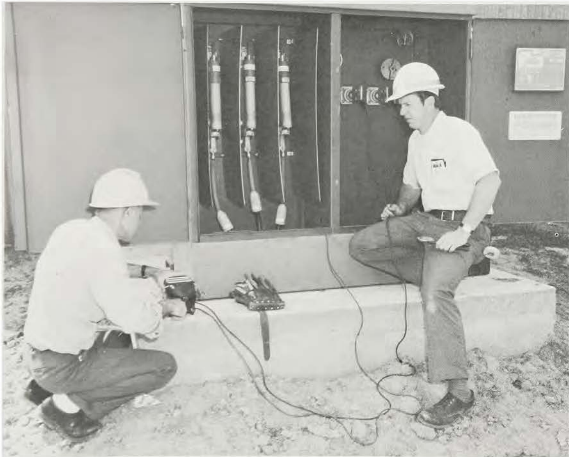
Engineering and Construction Services Division electricians check the insulation value of wiring in the power substation for WES' new Advanced Scientific Computer
