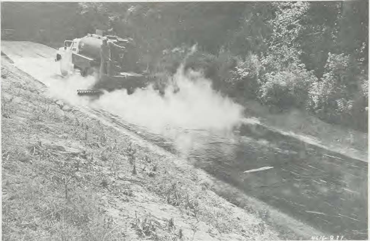
Final application of asphalt over polypropylene on experimental road at WES
