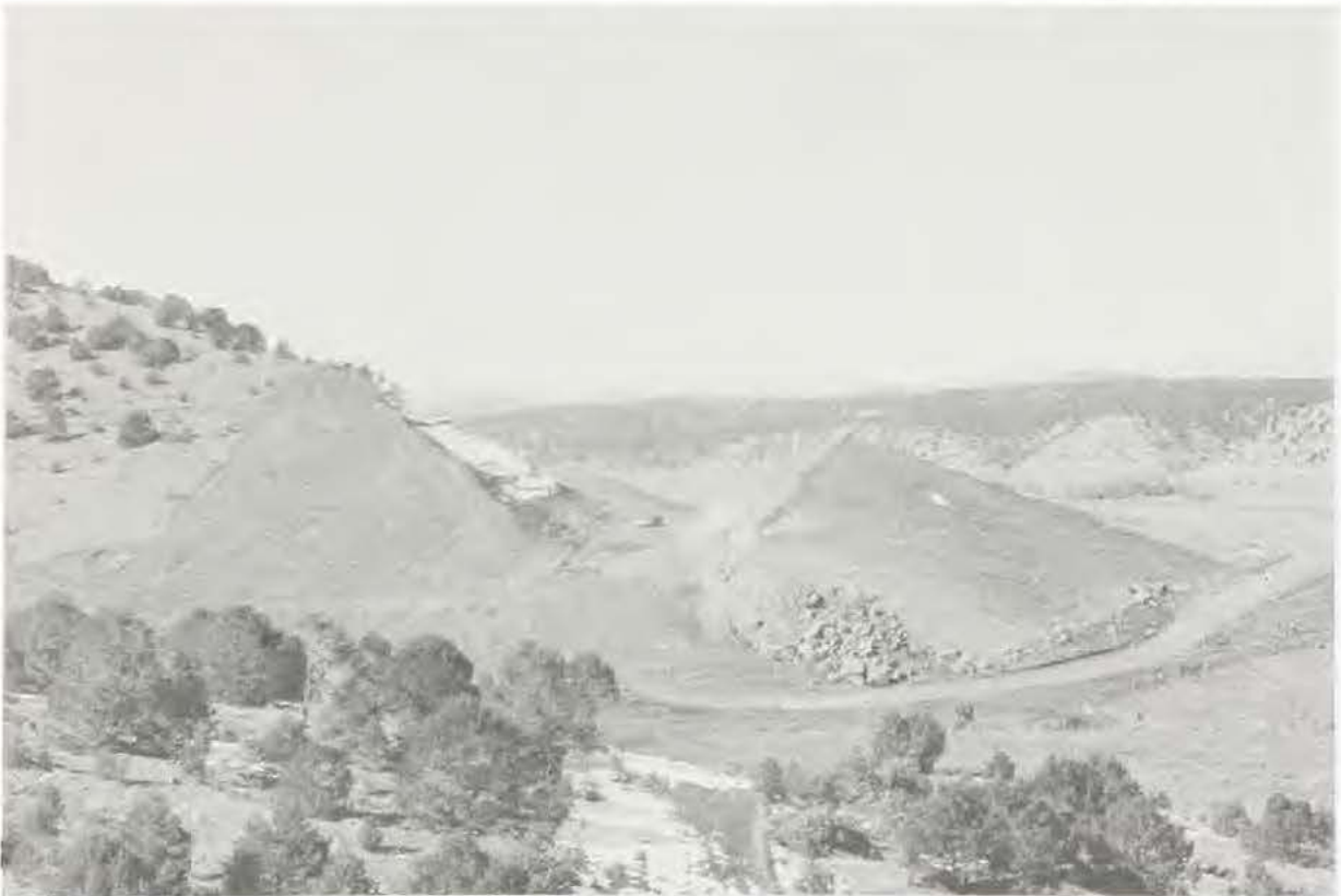
Railroad cut made by explosives
