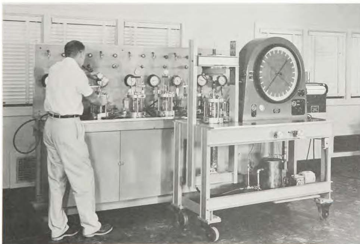
WES-built triaxial test apparatus
