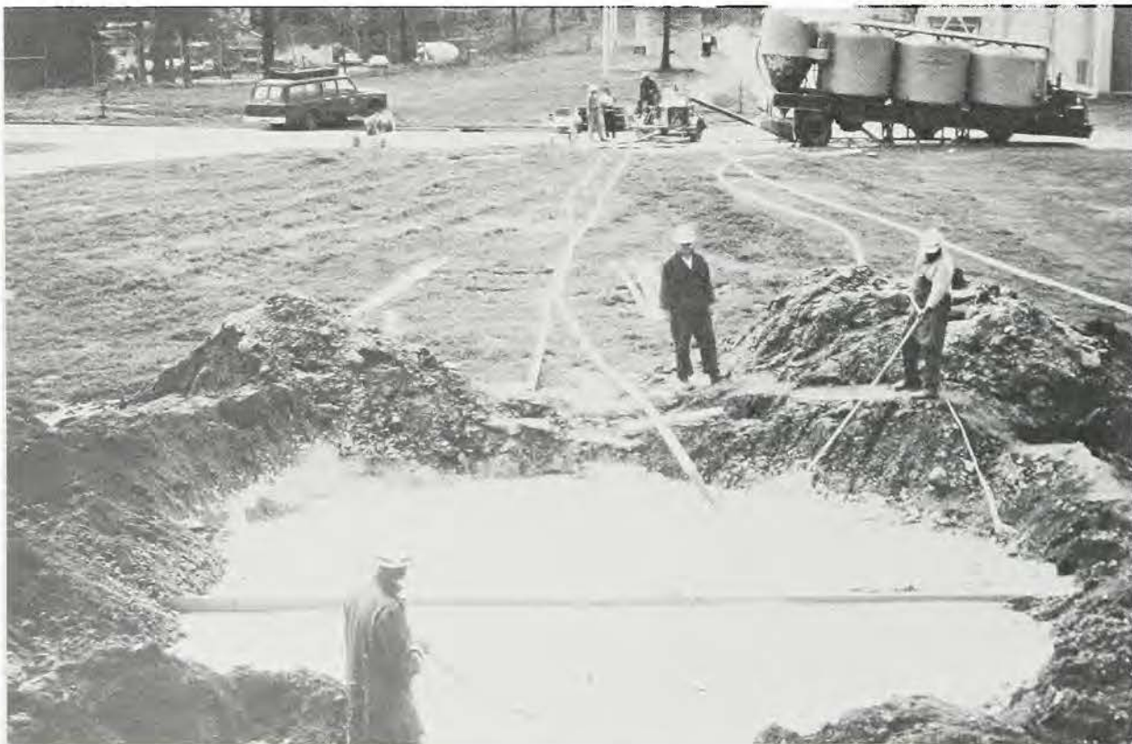
Placement of foam concrete
