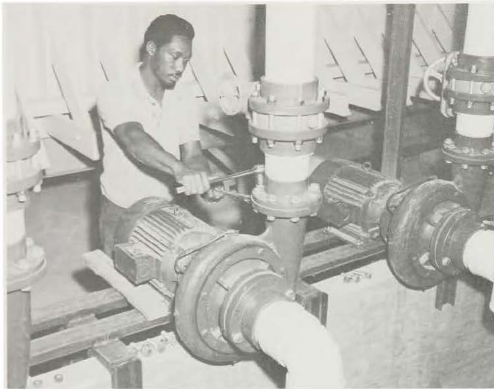
Pipe fitter working on the Pumping Station Research Facility
