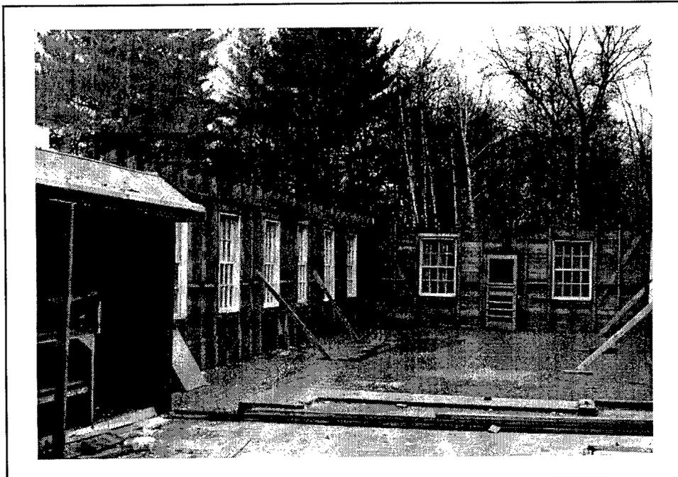
Figure 6. Wood-framed barracks in process of deconstruction.
