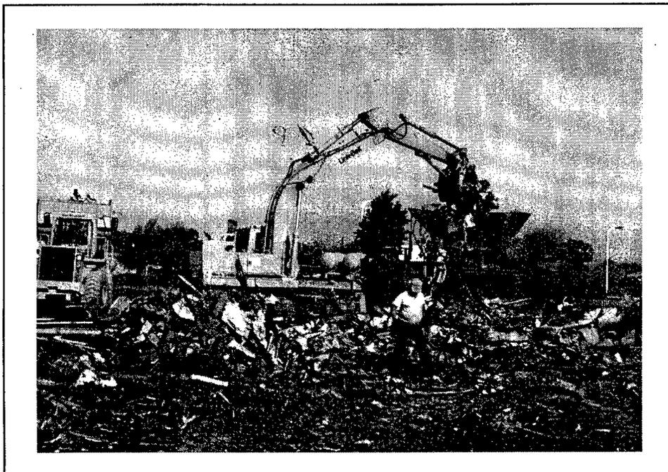
Figure 12. Demolition debris being loaded into debris compactor.
