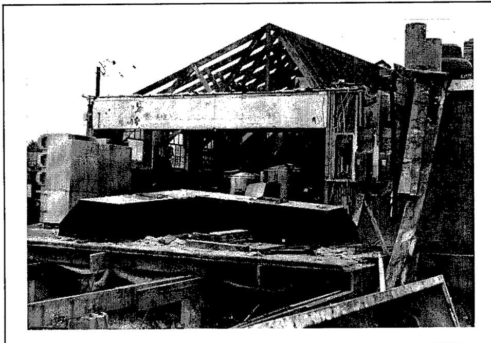
Figure 7. Wood-framed mess hall in process of deconstruction.
