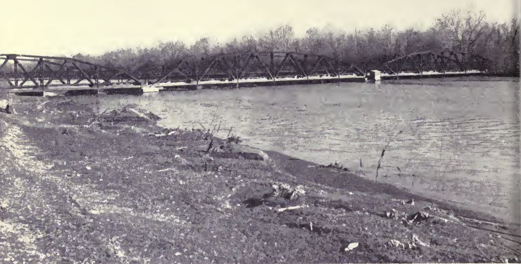
Highway bridge across Rio Grande River, near San Marcial, New Mexico, in summer 1952. Washout of the bridge is imminent and is due to backwater sedimentation caused by Elephant Butte dam below. (Photo by C. E. Redman.)
